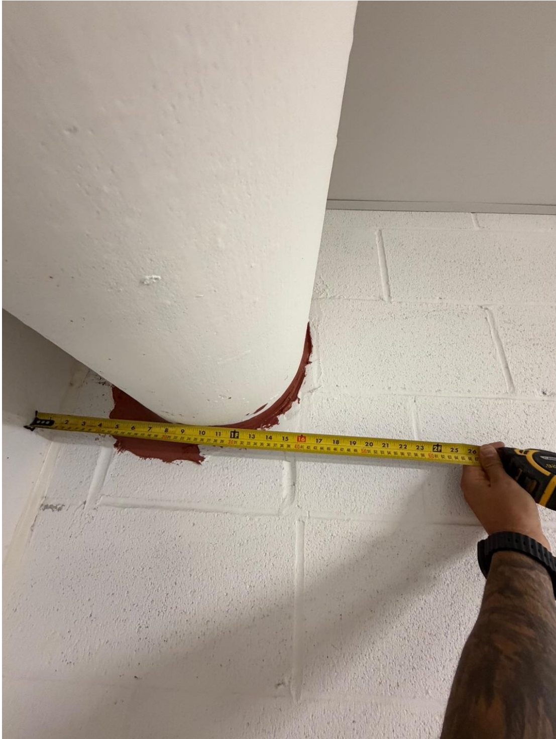
Photograph 2 – showing the distance between the building wall and the location where the Stormwater Pipe no longer affects the Building Code vertical clearance (2.0 metres) which is approximately 1.5 feet (0.45 metres) from the building wall
