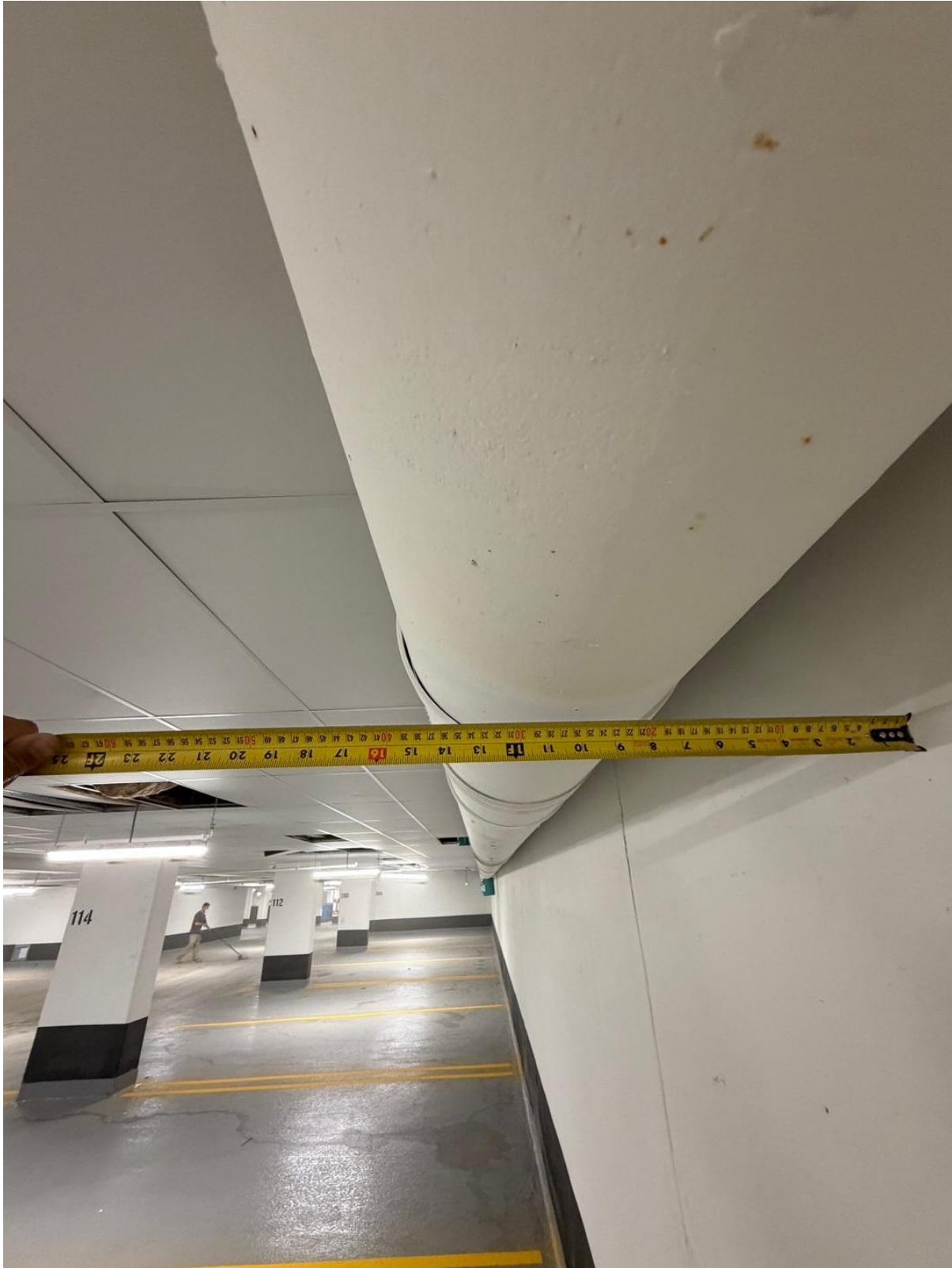
Photograph 3 – showing the location of the Stormwater Pipe from the wall from another angle
