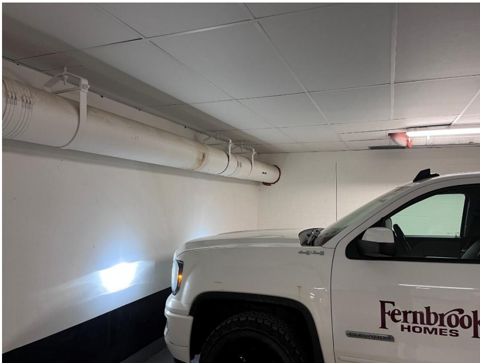
Photograph 5 showing a Fernbrook truck parking at the building wall from another angle
