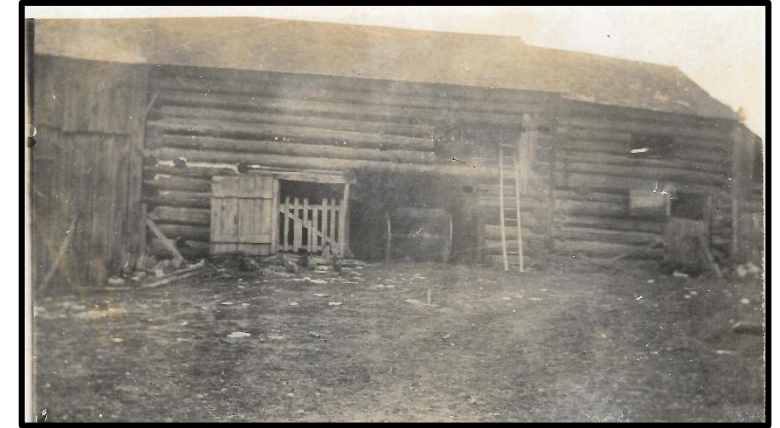
Original barn with attached sheds constructed in 1854
