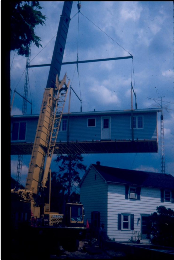
Rear addition to the historic log house constructed in 1991
