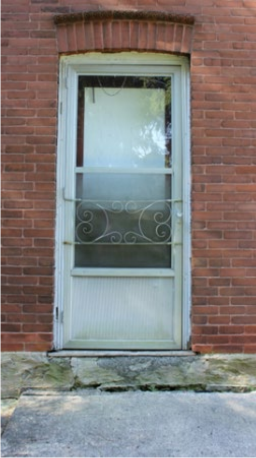
Exterior view of entrance door at Northwest elevation
