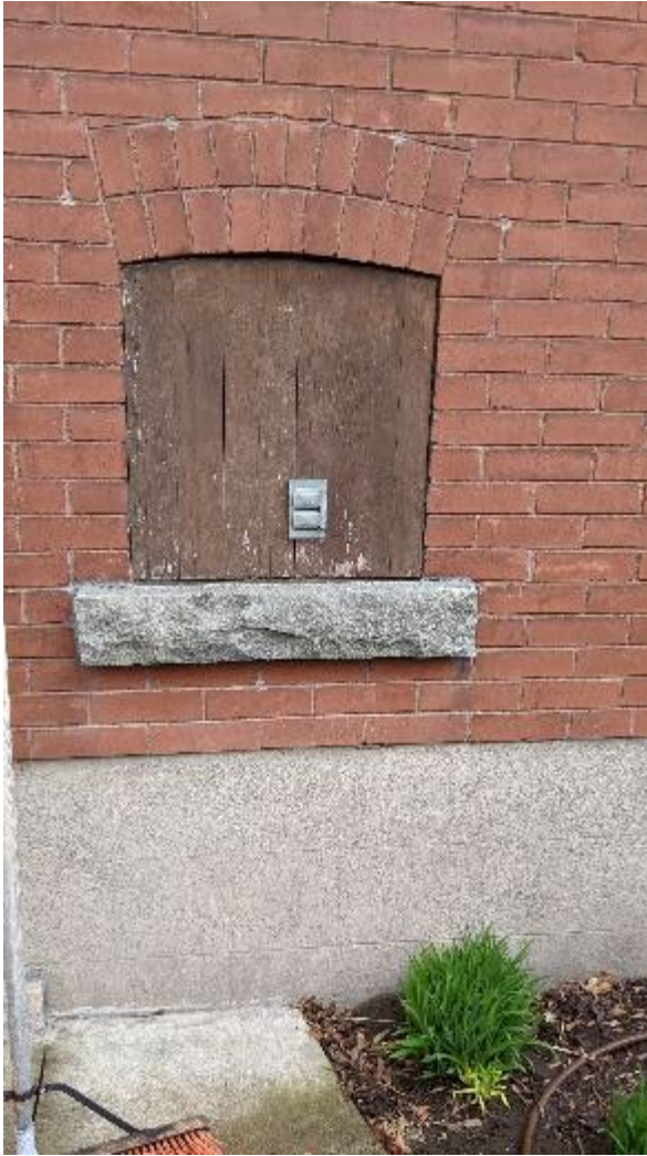
Window at West elevation
