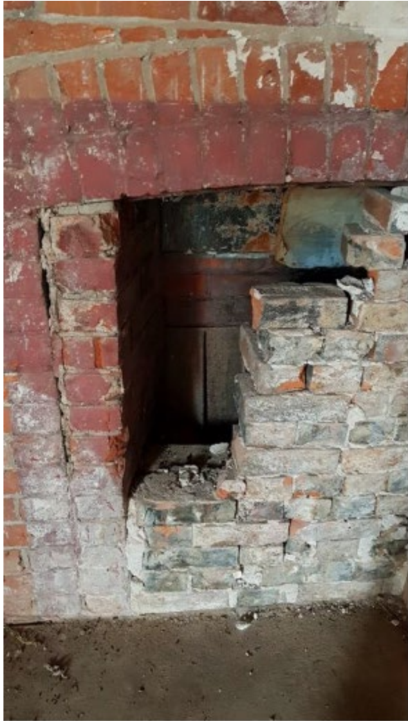
Prior to restoration Fireplace 1
