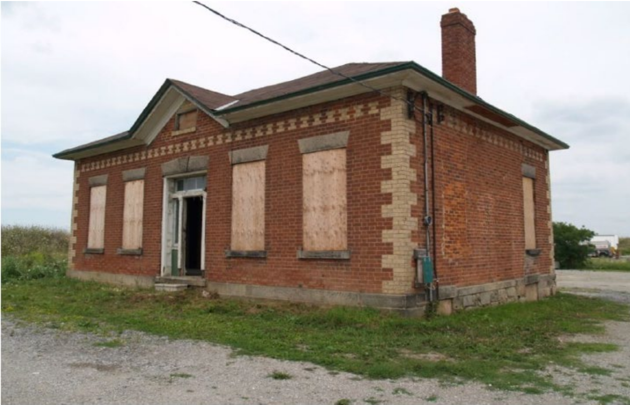
West and South Façade Before Rehabilitation
