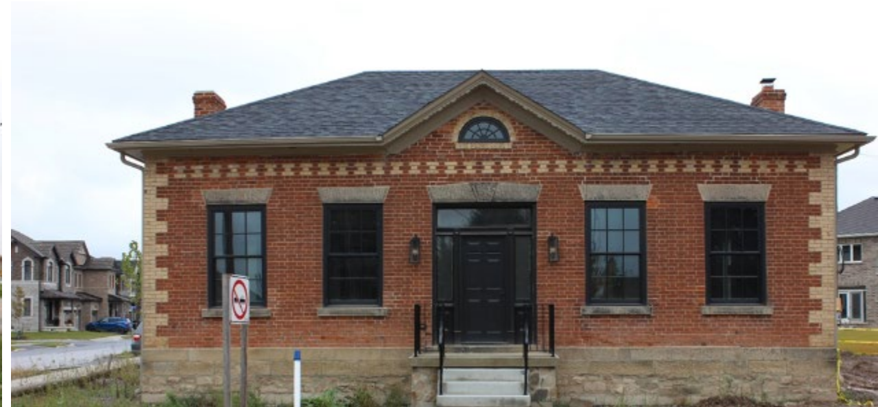
West Façade After Rehabilitation
