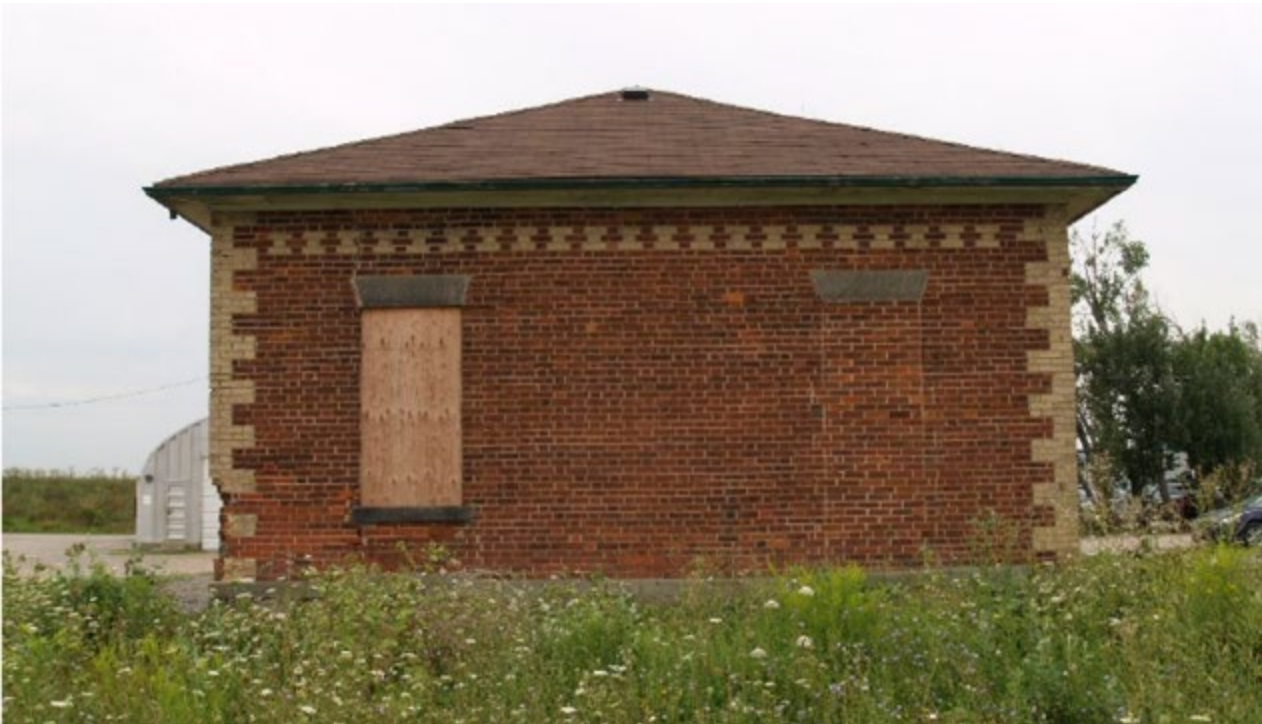
North Façade Before Rehabilitation
