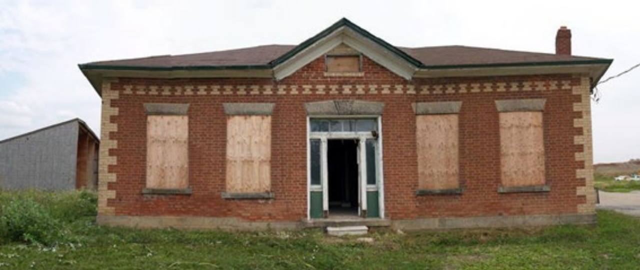
West Before Rehabilitation
