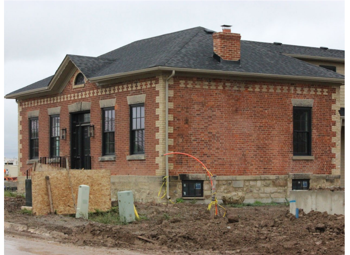
West and South Façade After Rehabilitation
