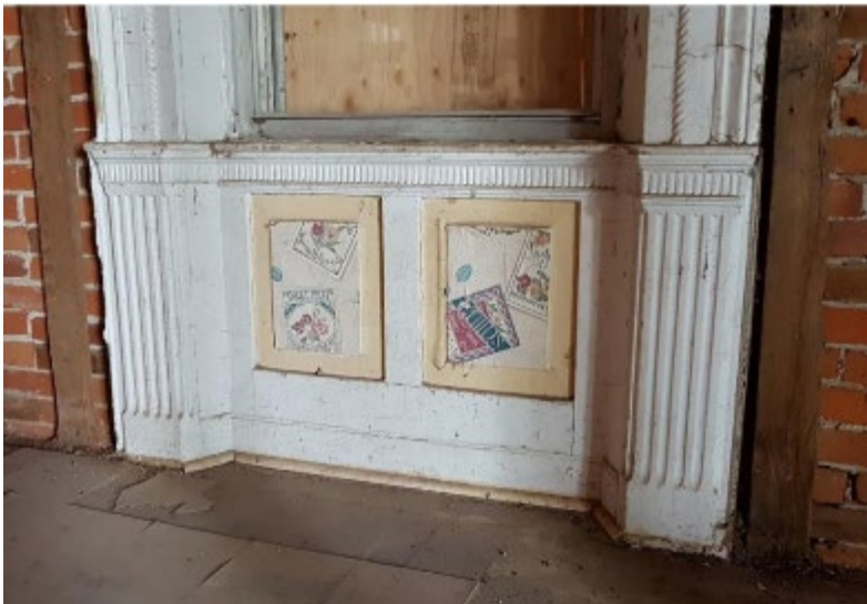
Prior to restoration
