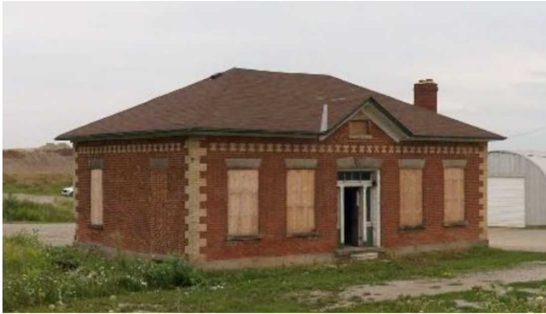
North East Façade Before Rehabilitation
