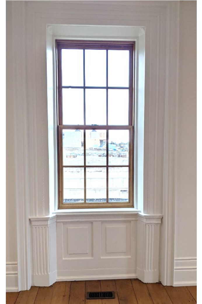
Restored Window Casing
