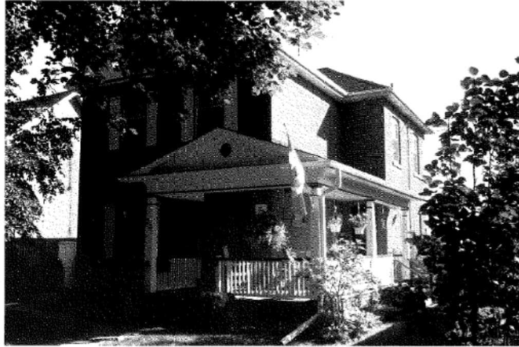
This is a post World War I, Eclectic Style, two-storey brick home with a cross gable plan and a gable facing the street. Segmental brick arches and stone sills are features of the construction. The side hall entrance has a pedimented wrap-around porch.
