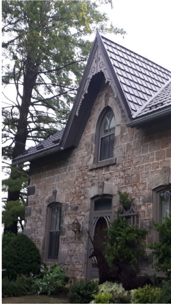
Decorative Verges on the North Elevation
