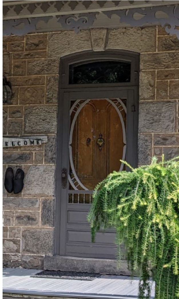
Door on West Elevation
