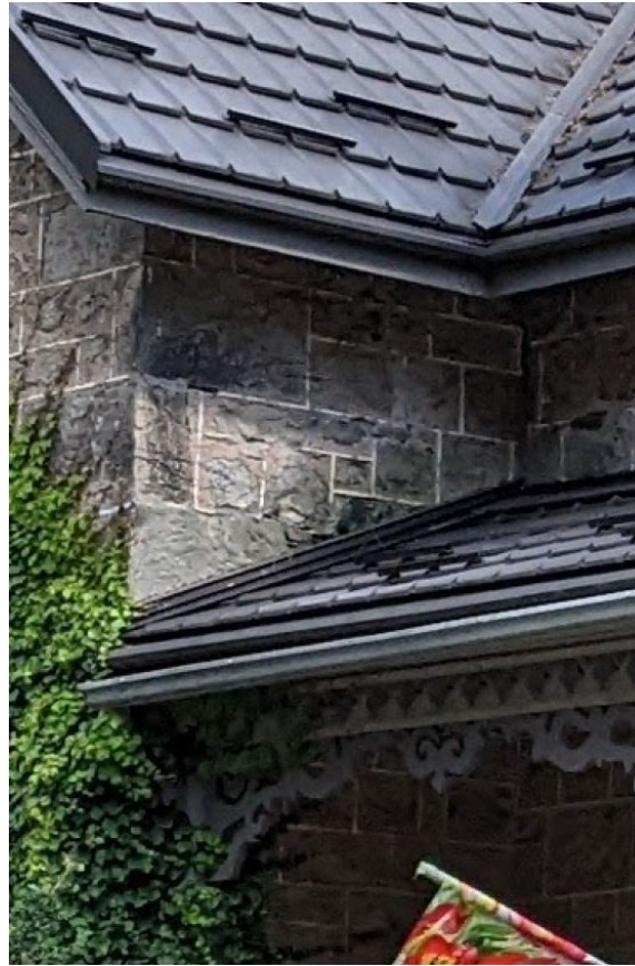
West Elevation at Porch
