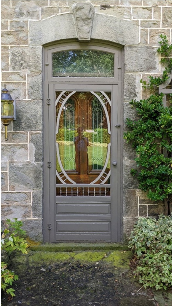
Door on North Elevation
