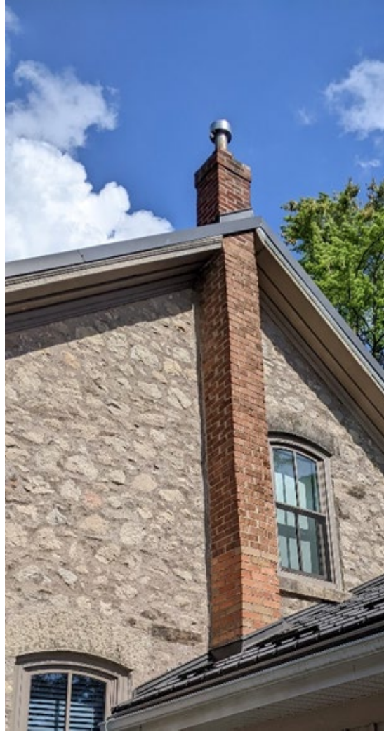
Chimney South Elevation
