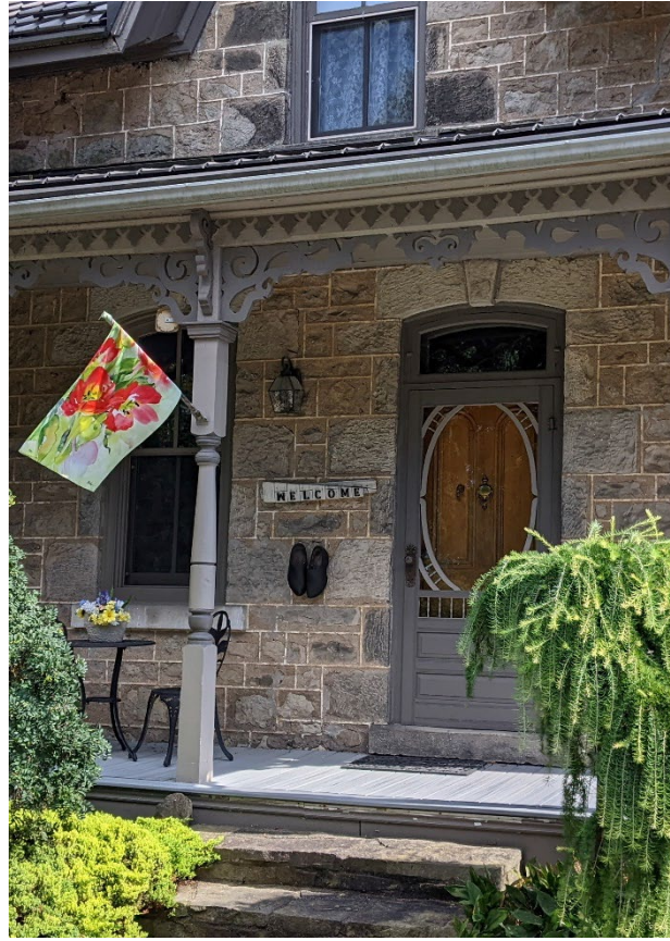
Side Entrance Porch Door
