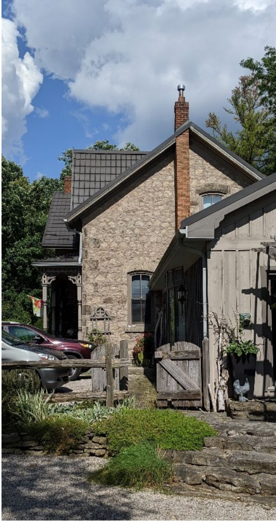
Chimney South Elevation
