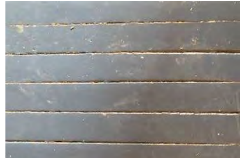
Original Maple floor
