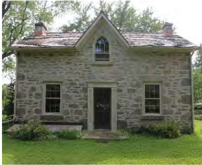
Chimneys at East and West End
