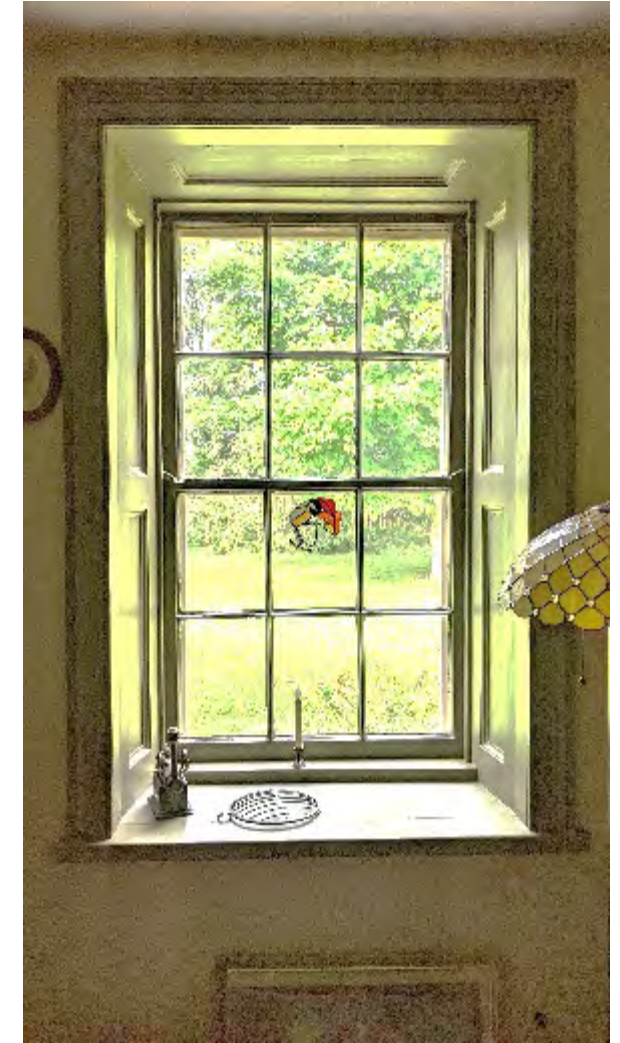
Interior View of Windows
