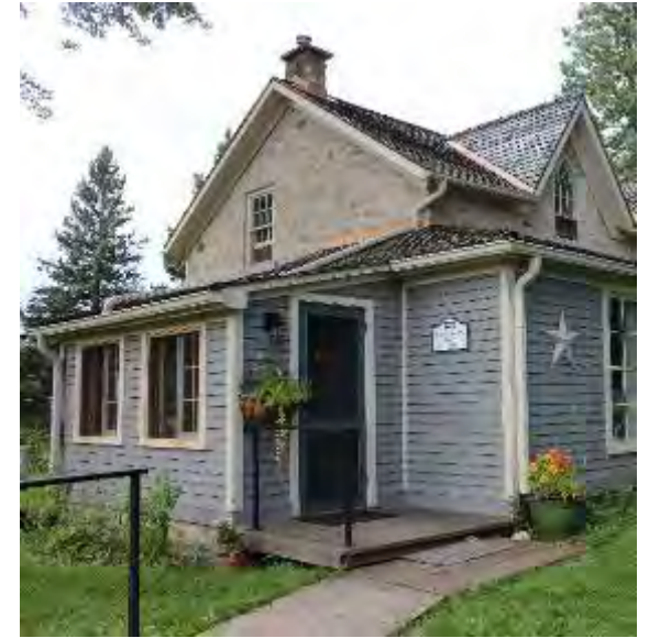
Chimney at South End
