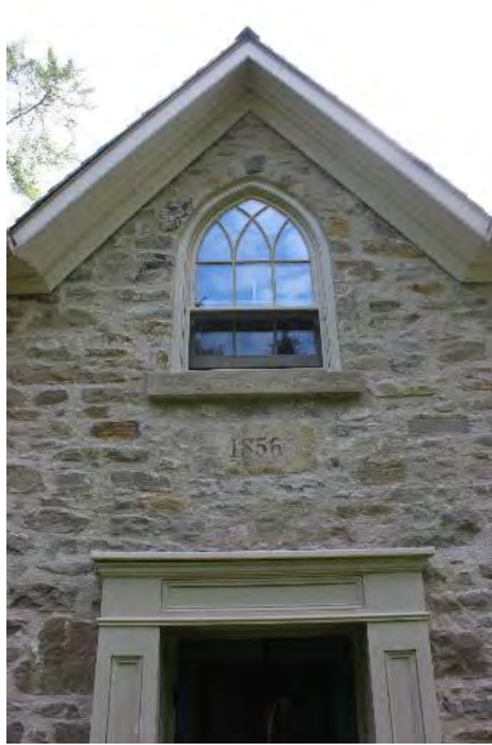
North Elevation Gothic Window 1984
