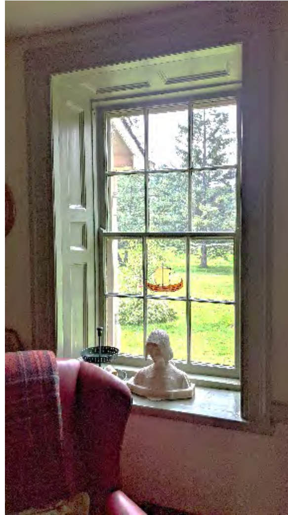
Interior View of Windows
