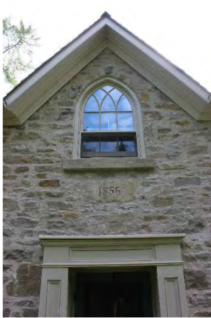
North Elevation Gothic Window 1984
