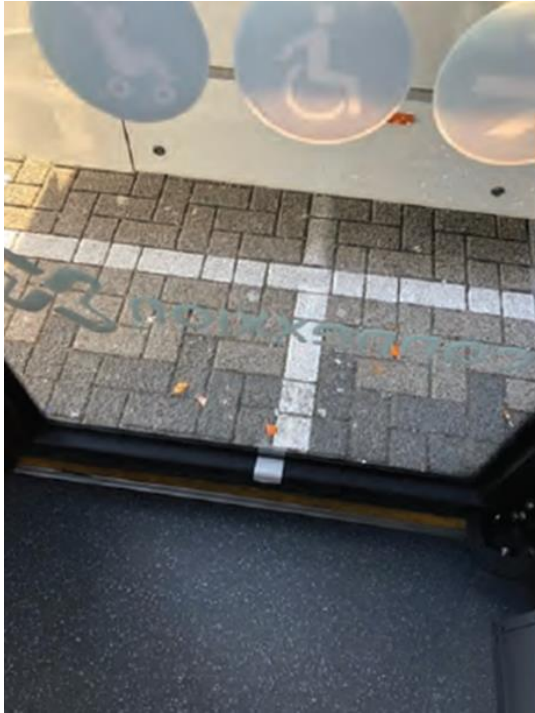
Figure 26. Example of Alignment Markers for Proper Bus Positioning 11
