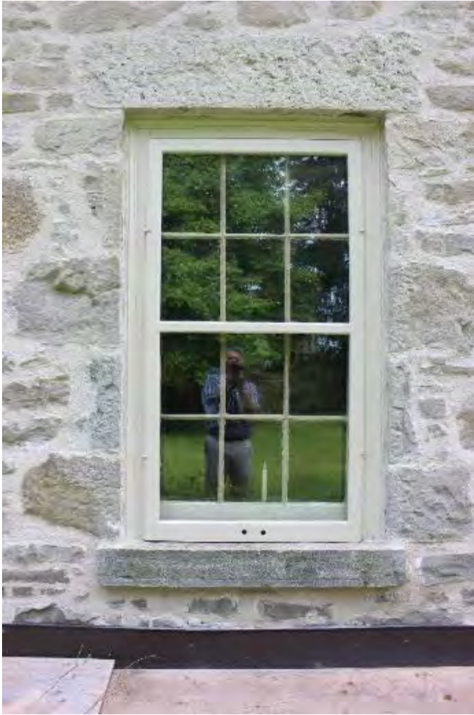
North Elevation Window
