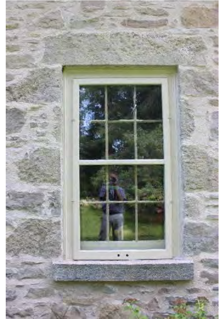
North Elevation Window
