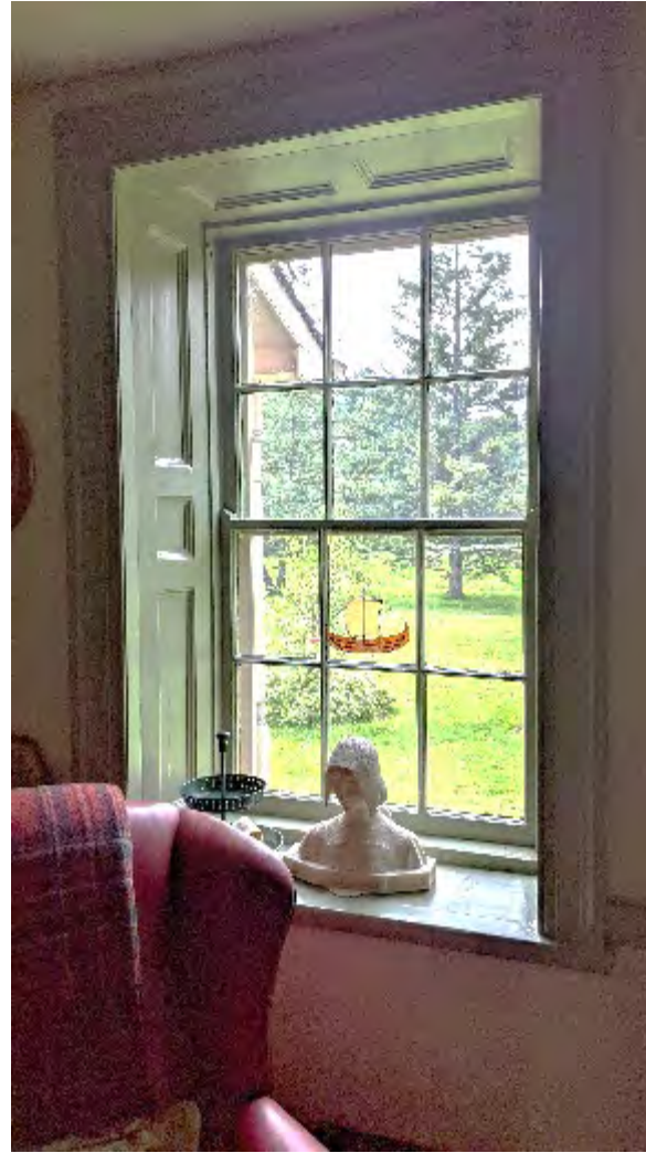
Interior View of Windows
