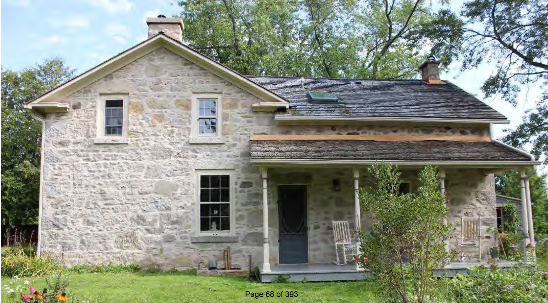
West Elevation _ Porch added 1996
