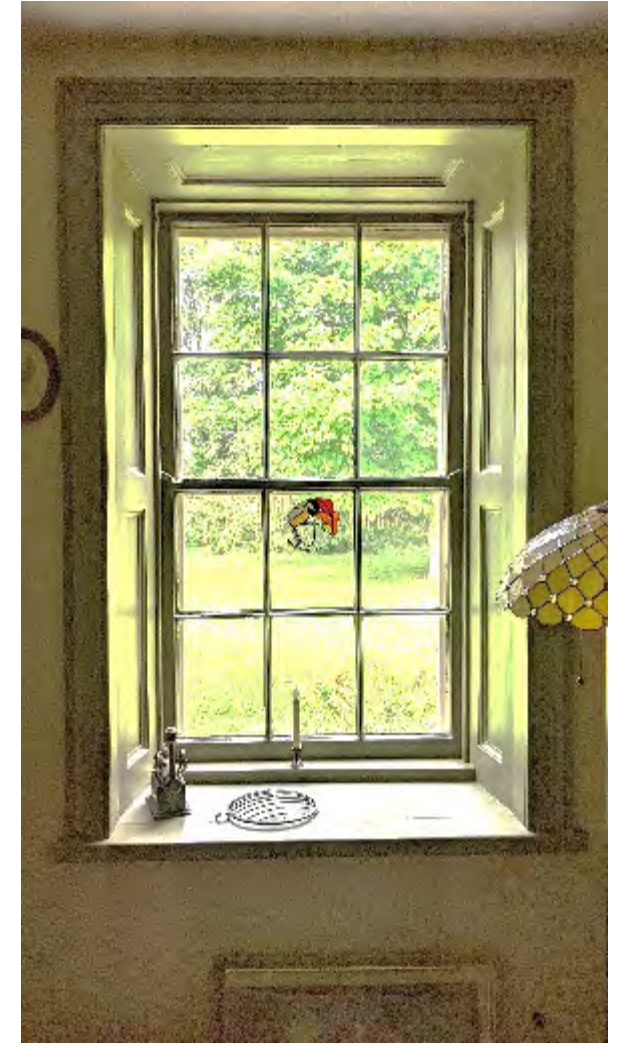
Interior View of Windows
