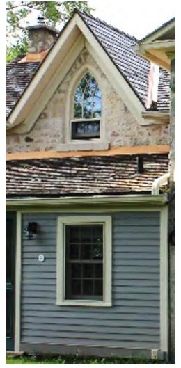
East Elevation Gothic and Six over Six Windows
