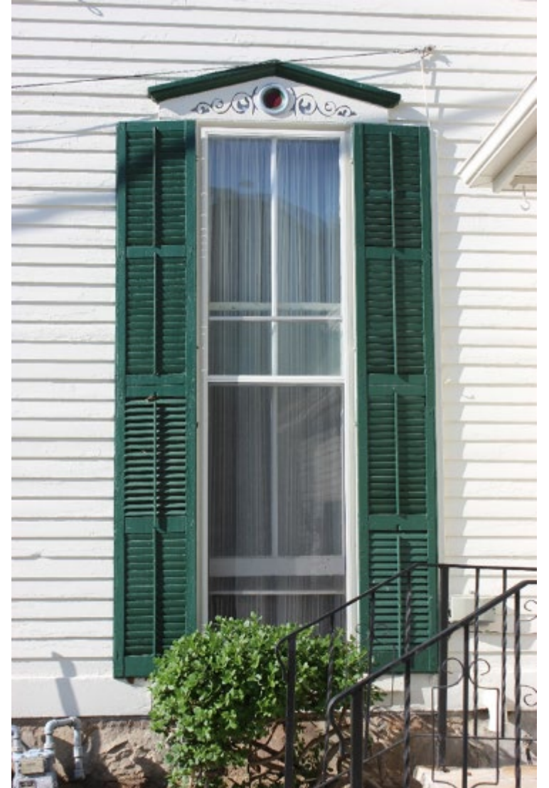
Ground Floor East Elevation Window
