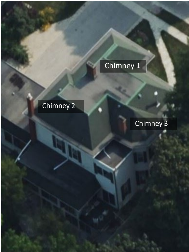
Location of Chimneys
