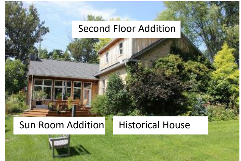
Rear sun room addition
