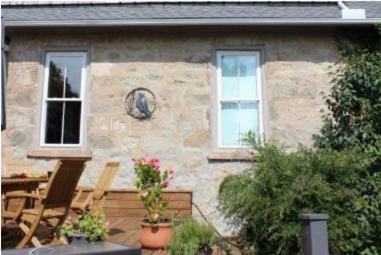
Stone wall at rear elevation
