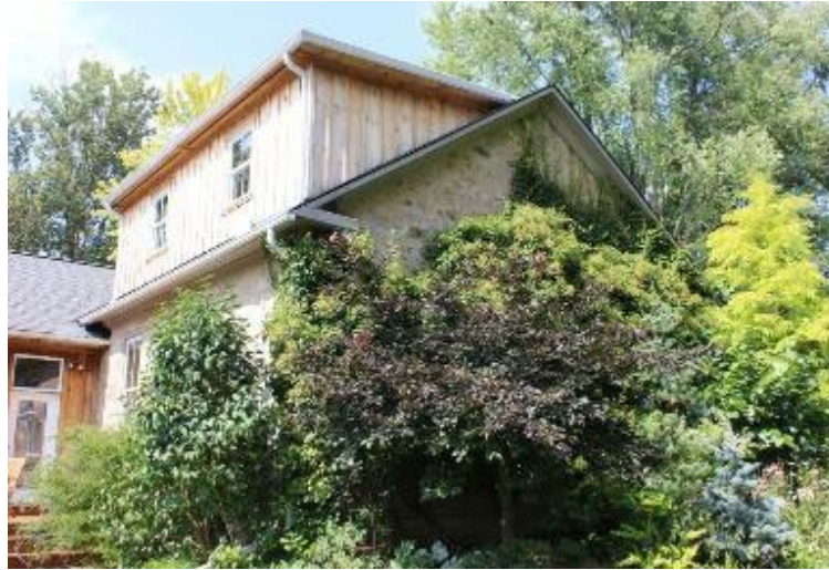
Second floor addition at rear
