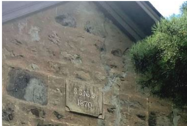
1870 Date Stone below gable roof
