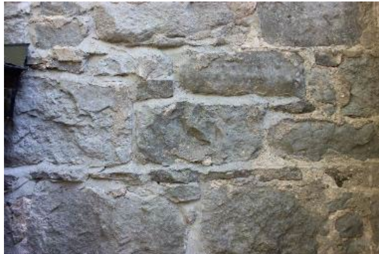
Exterior random rubble stone wall
