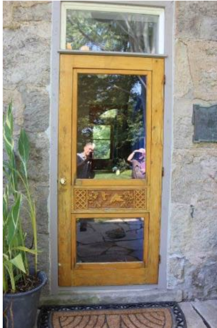
• Front Entrance Door
