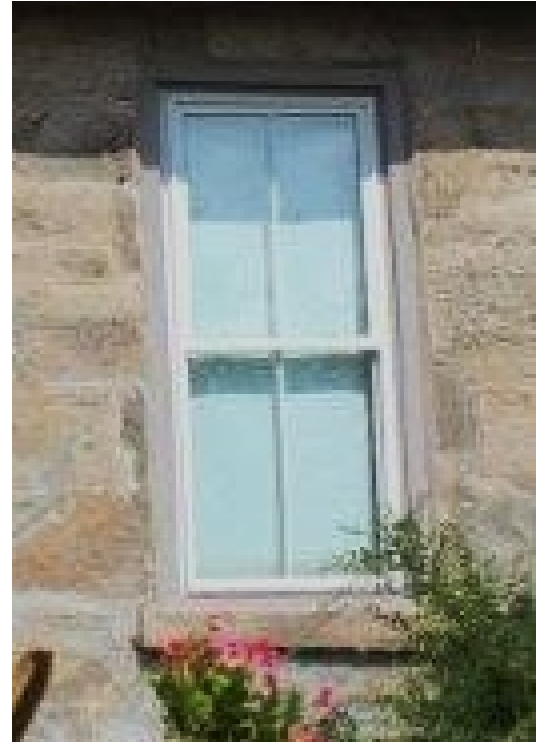
Rear Elevation Window
