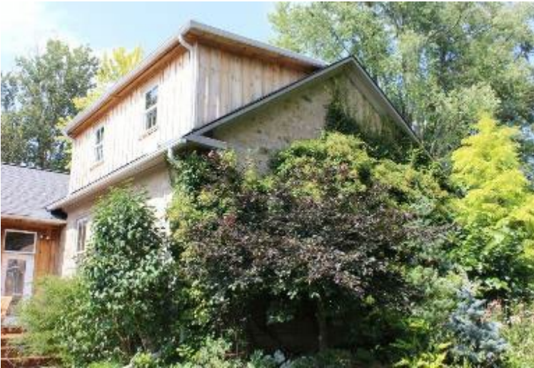
Second floor addition at rear
