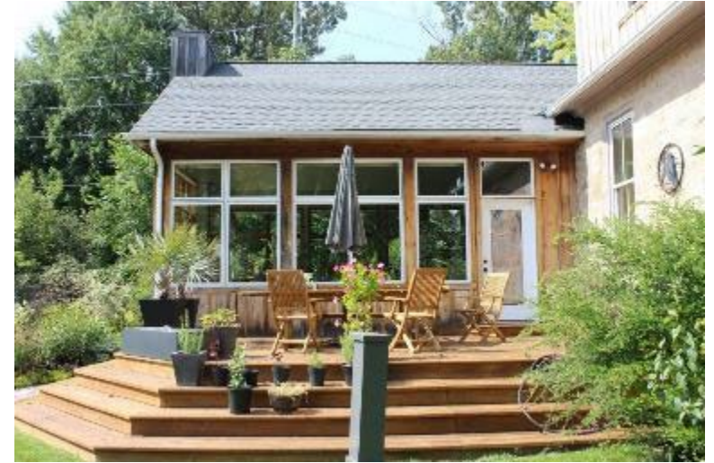
Southern Elevation Sun Room Addition
