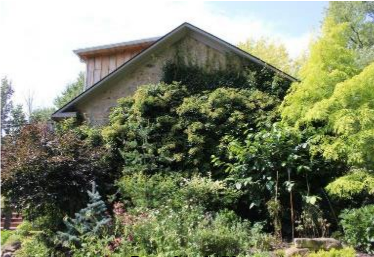
Historical House Side Elevation (South)
