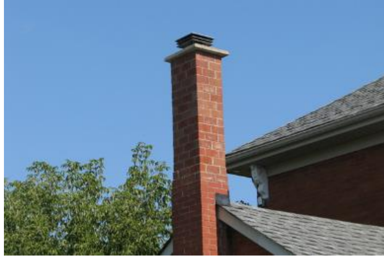
Second Chimney seen from the rear elevation
