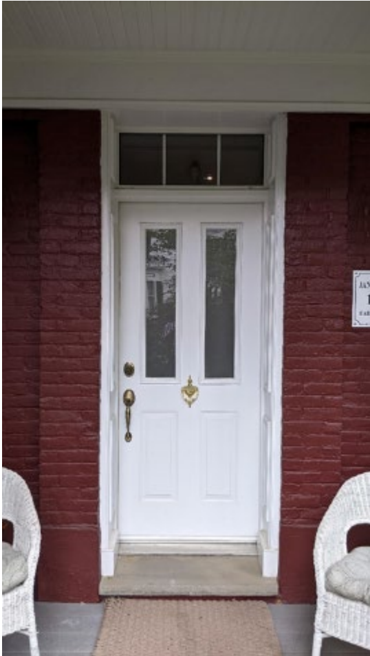
Central Entrance door
