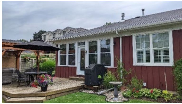
South (Rear) Elevation showing additions
