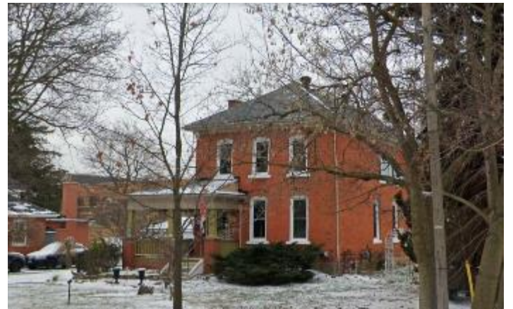
Chimney seen from Martin Street
