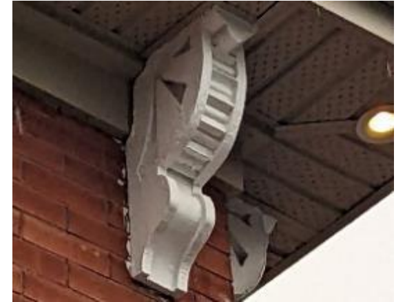
Roof Brackets details
