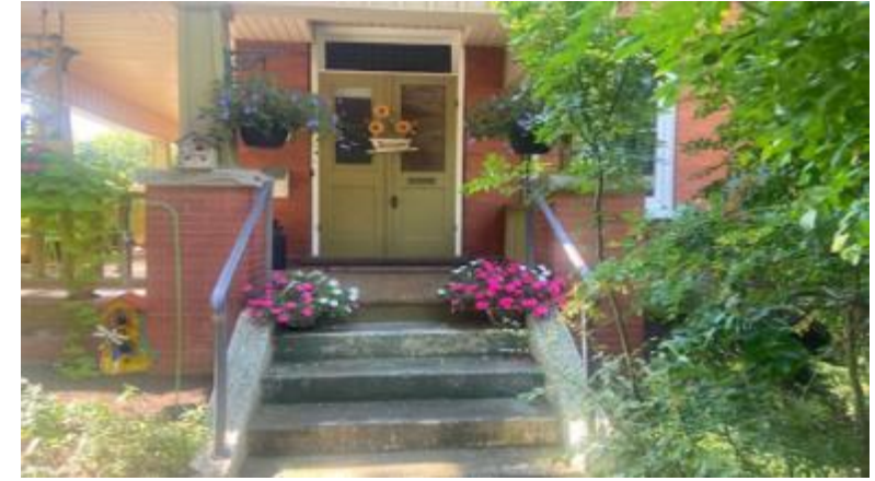
Wrapped Around Porch entrance at front elevation
