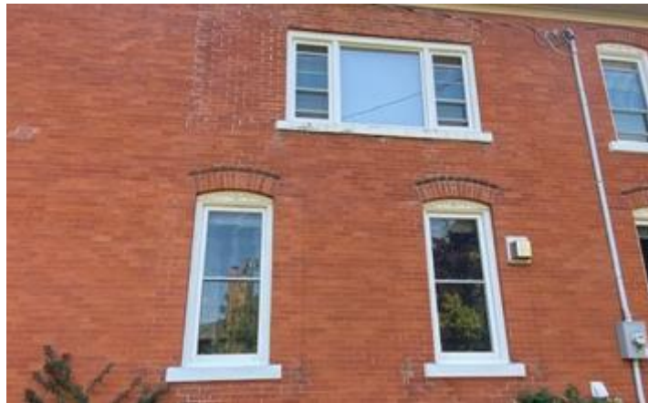
Windows on South Elevation
