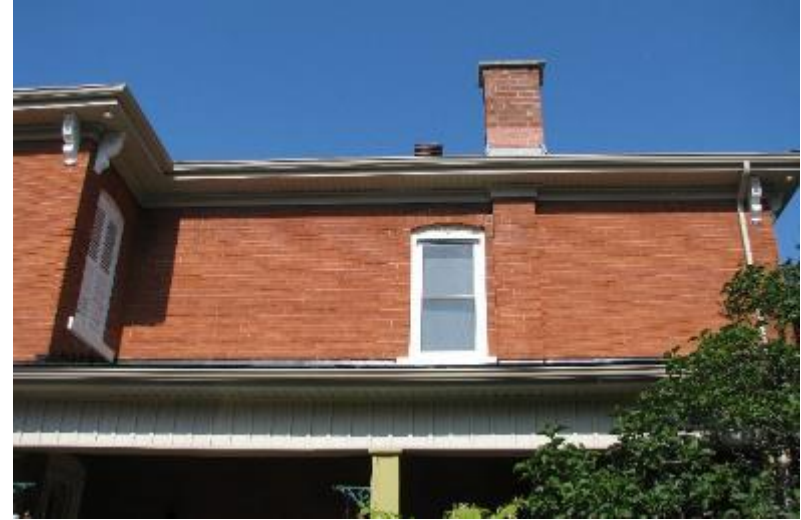
Chimneys seen from the south elevation
