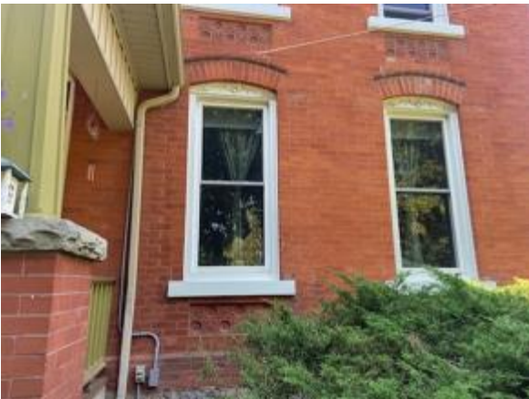
Double Sash Windows on ground Floor
