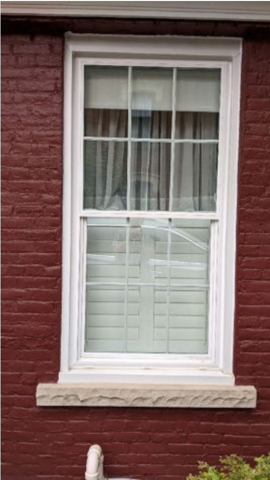
East Elevation Windows
