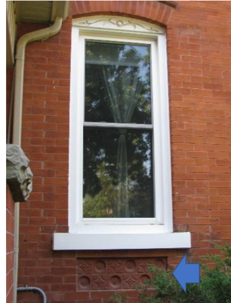
Location of Brick tiles along Front Elevation
