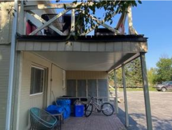
East Elevation at Deck
