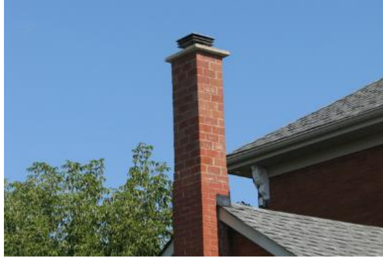
Second Chimney seen from the rear elevation
