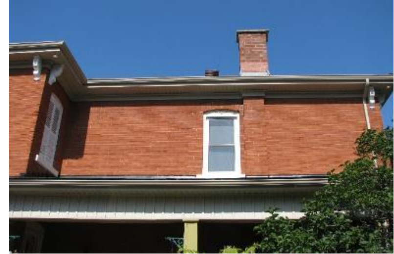
Chimneys seen from the south elevation
