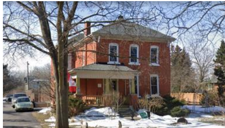
East Elevation along Martin Street, 2022
