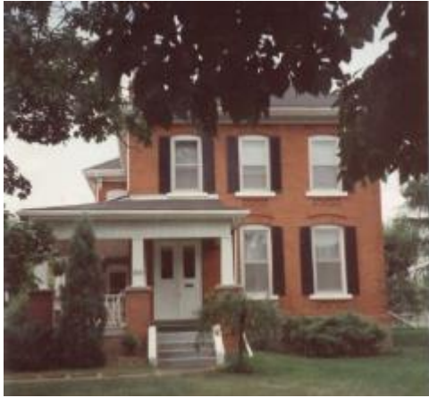
East Elevation along Martin Street, 1991
