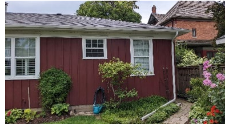
South Elevation (1995 additions)
