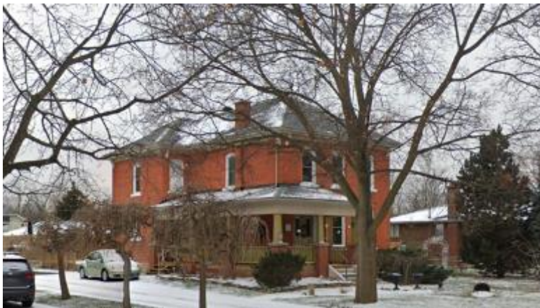
East Elevation along Martin Street, 2022
