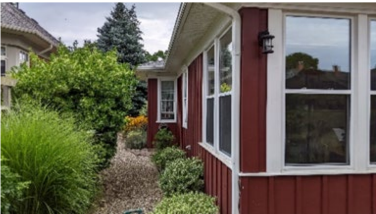
West Elevation (1995 additions)
