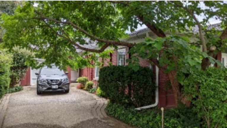
Elevation along Victoria Street, 2023
