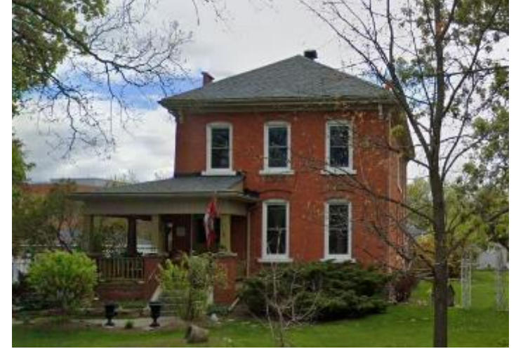
East Elevation along Martin Street, 2023
