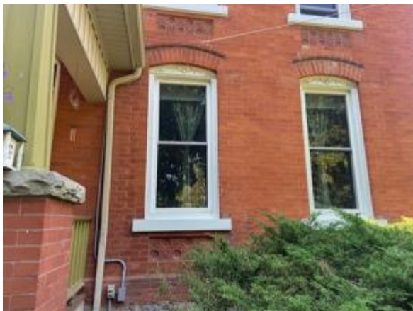
Double Sash Windows on ground Floor
