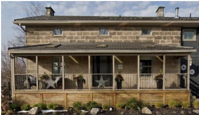
Elevation along Mill Street, 2023
