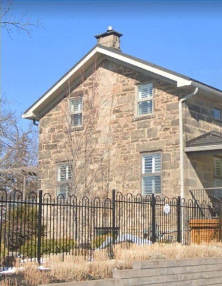
Windows on West Elevation
