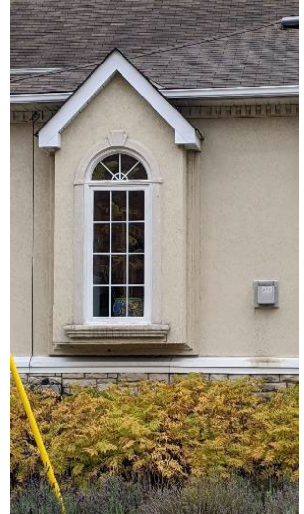
Existing Window West Elevation
