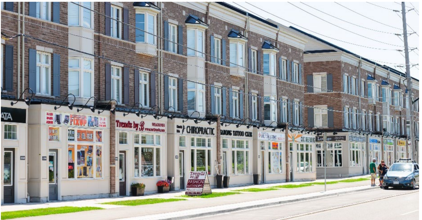
Figure 38. Mixed use employment and residential apartments (Town of Milton files).
