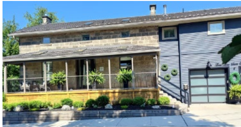
View of the Historical House and Additions
