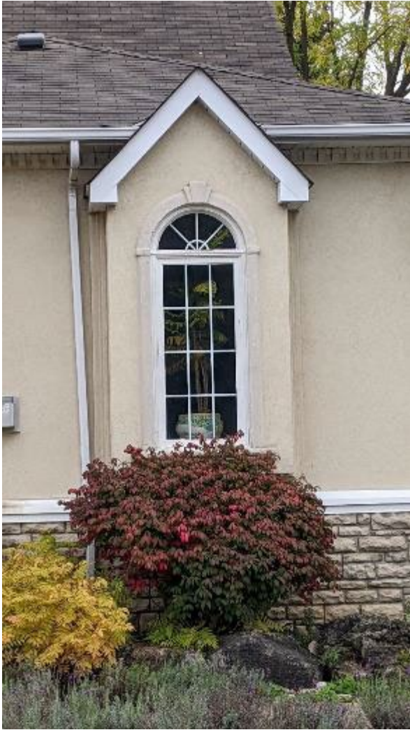
Existing Window West Elevation
