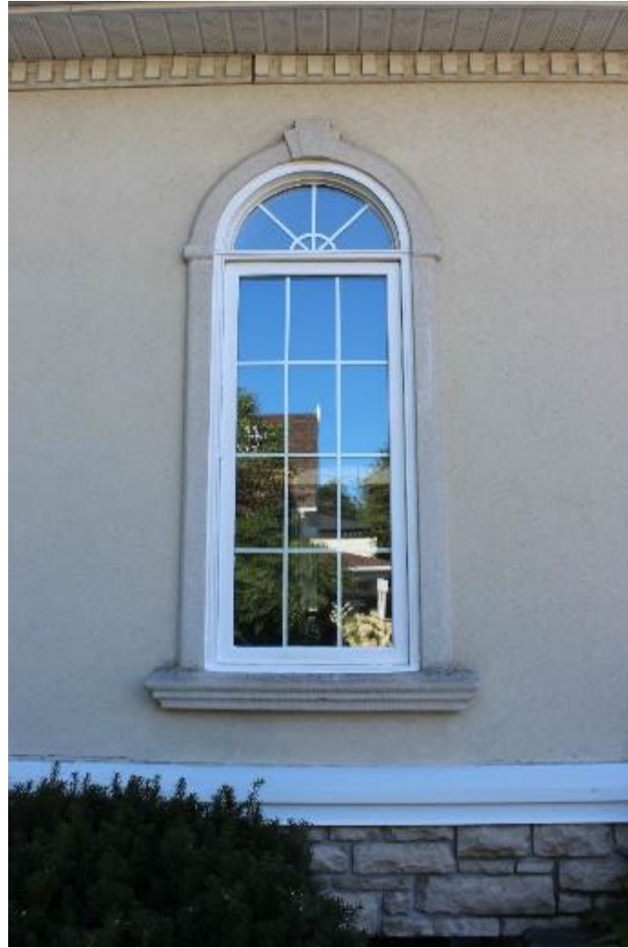
Existing Window North Elevation
