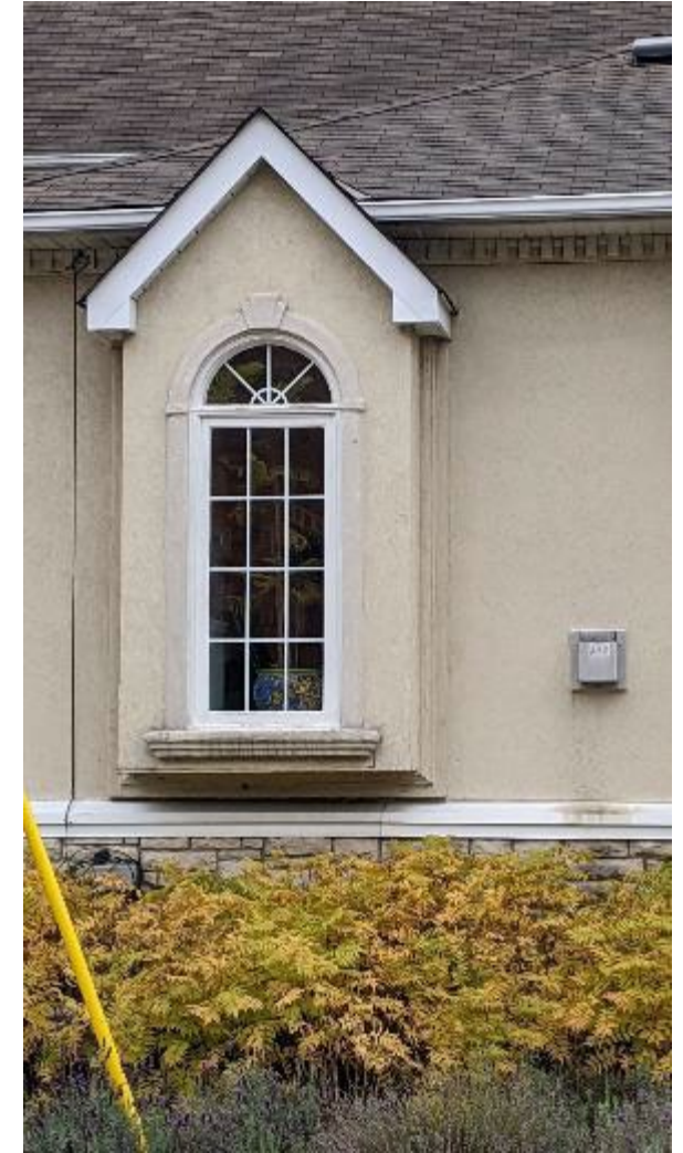
Existing Window West Elevation
