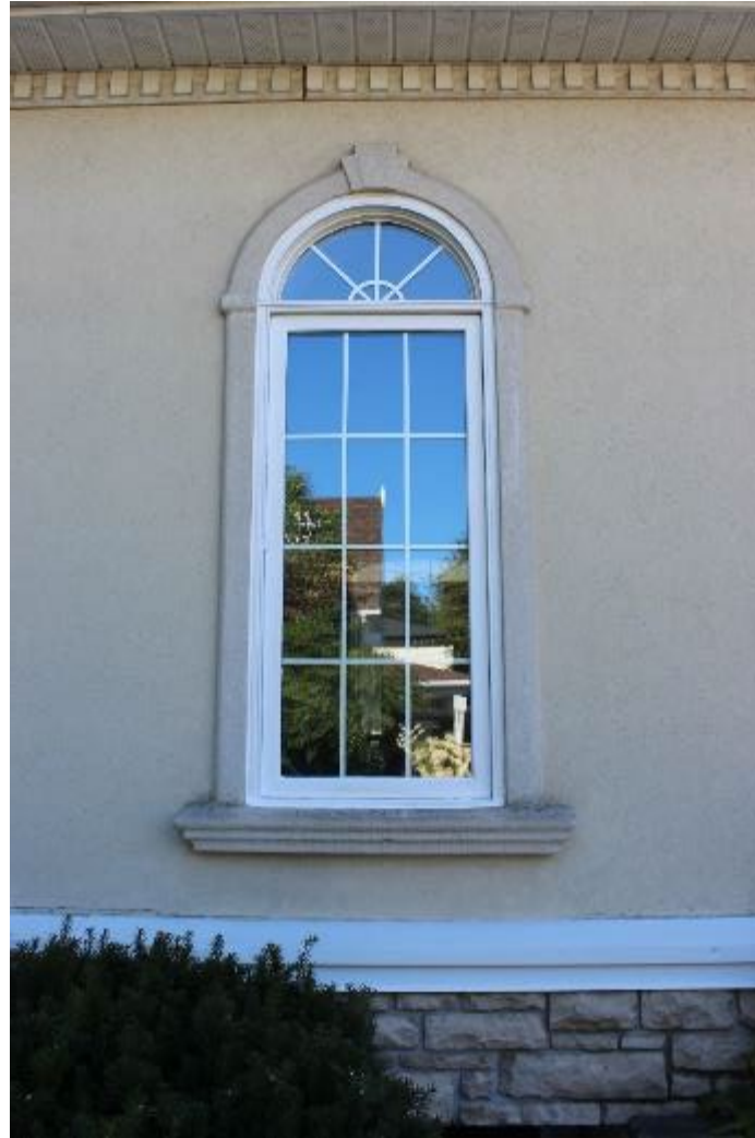
Existing Window North Elevation
