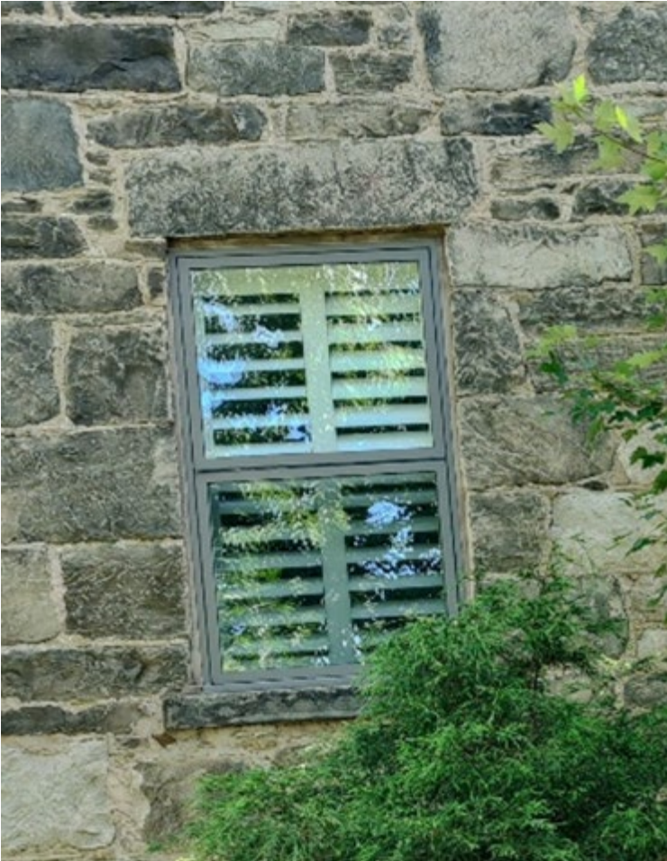
Windows at East Elevation
