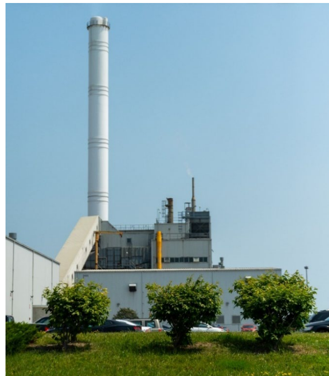
Figure 39. Manufacturing plant in Milton (Town of Milton files).
