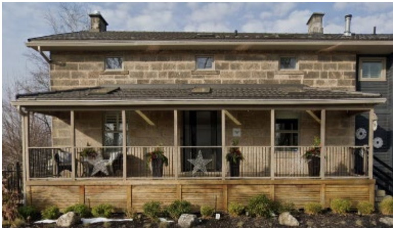
Elevation along Mill Street, 2023
