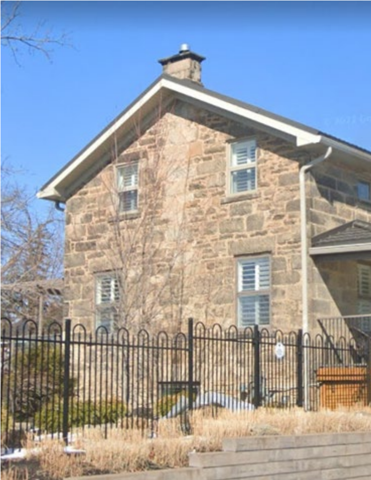
Windows on West Elevation
