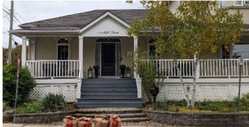
Existing Verandah Page 38 of 402
