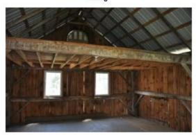
Square log timber framing, which is exposed to the interior
