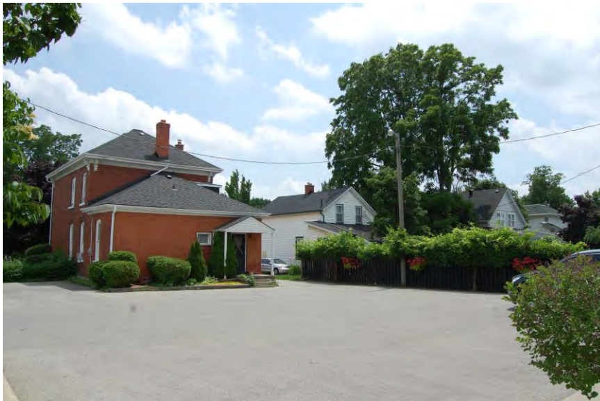
Figure 137 – 117, 111, 107 and 99 Mary Street, seen from rear at Brown Street (Photo: RHC, June 2014)
