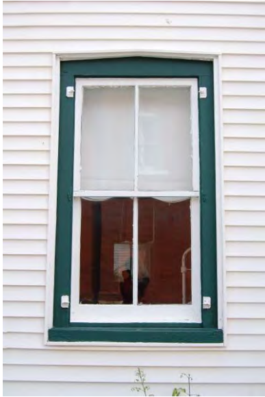
Original wood cladding with 2 over 2 windows
