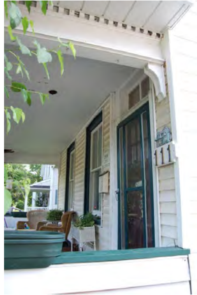
Front porch, enclosed upper sleeping porch and side bay window
