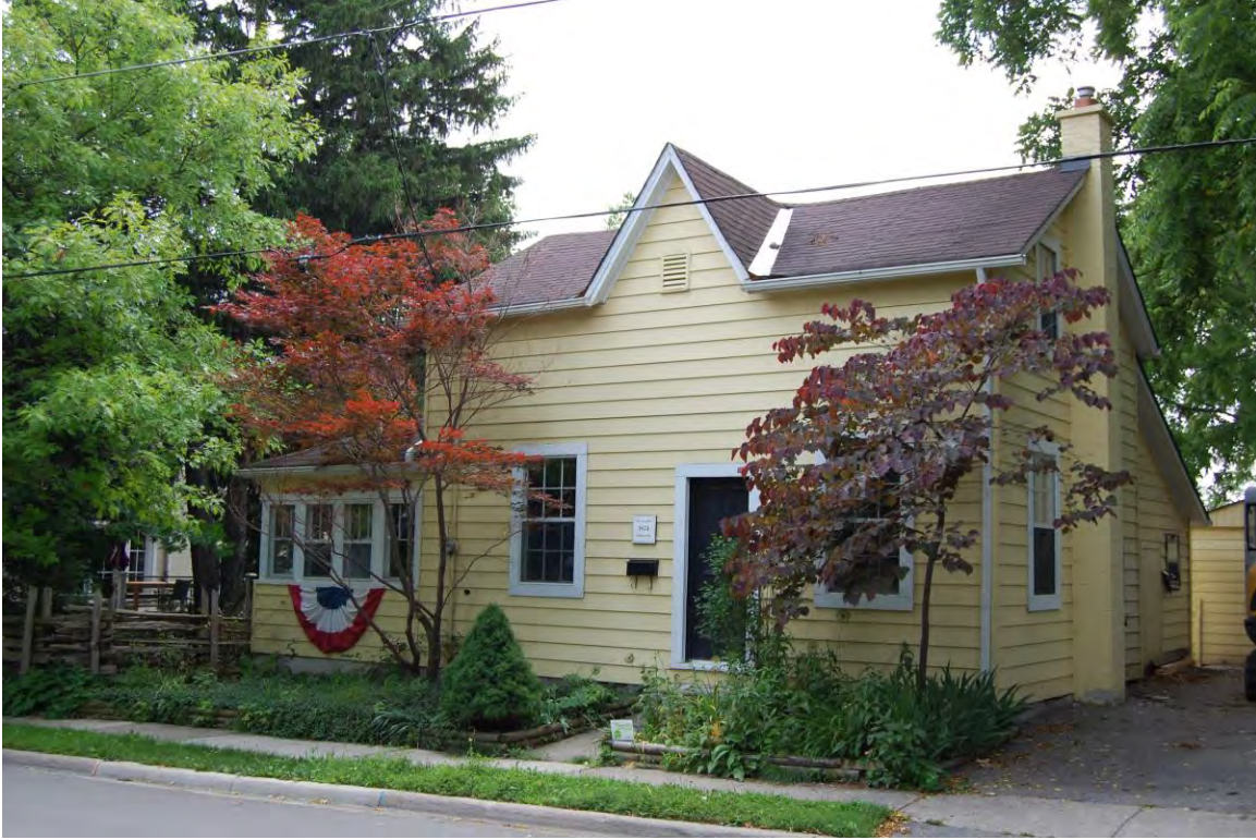
Figure 149 – 48 Bell Street (Photo: RHC, June 2014)
