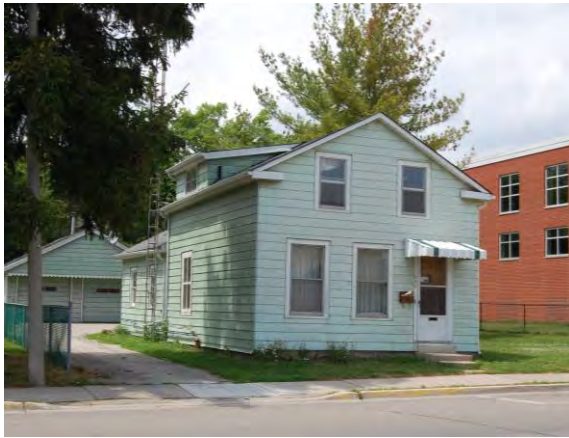
Figure 143a – 101 Main Street East (Photo: RHC, June 2014)
