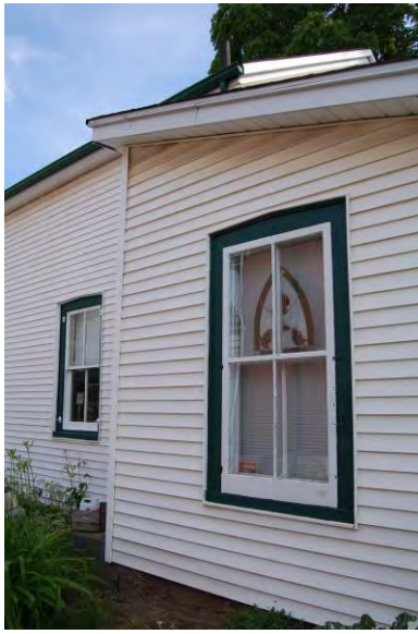
Original wood cladding (with horizontal orientation and V-groove joint).
