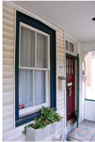
Original window and door elements of the original house (front and sides of the main block and kitchen tail) including their pedimented heads.
