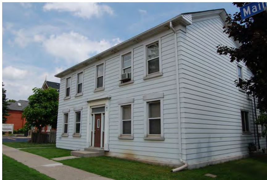
Figure 141 – 94 Main Street East (Photo: RHC, June 2014)
