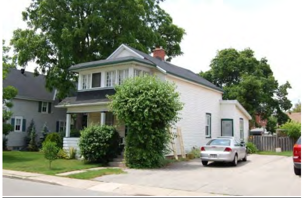
The original form, rooflines and massing of the one and a half storey house exterior
