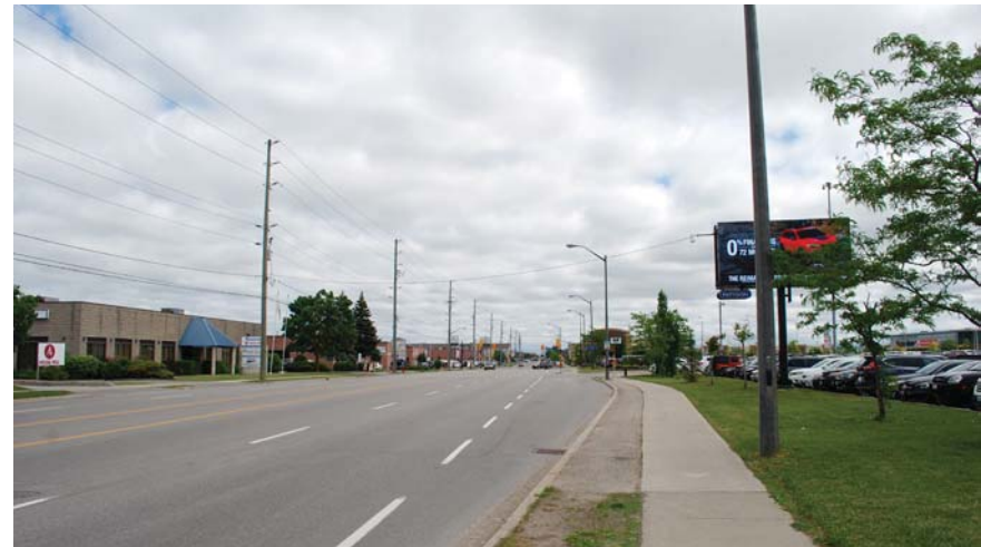
Automobile-oriented Main Street East with limited street tree planting and pedestrian amenities
