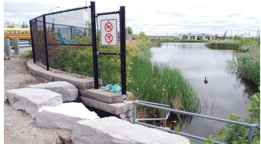
Storm water pond along the northern side of the railway tracks, east of Milton GO Station
