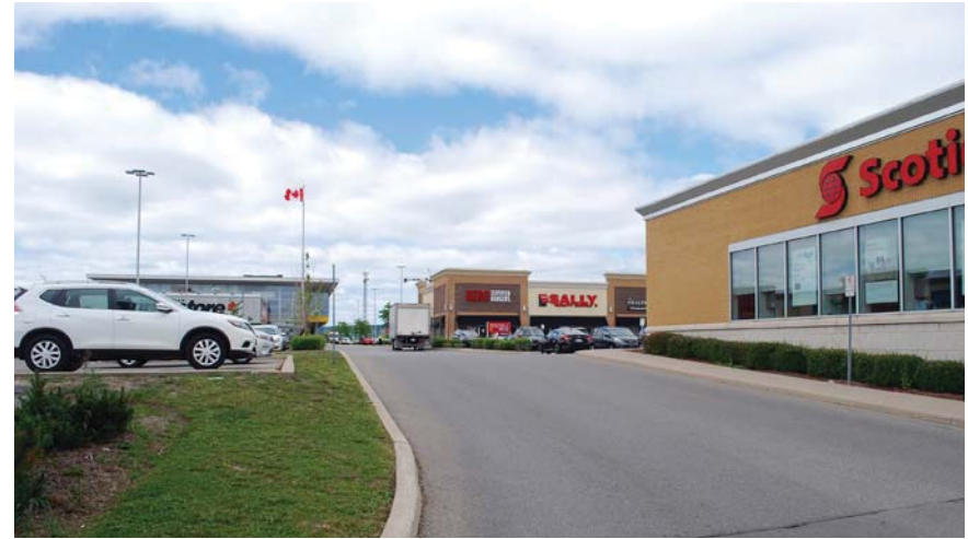
Commercial plaza, north east of the Milton GO Station
