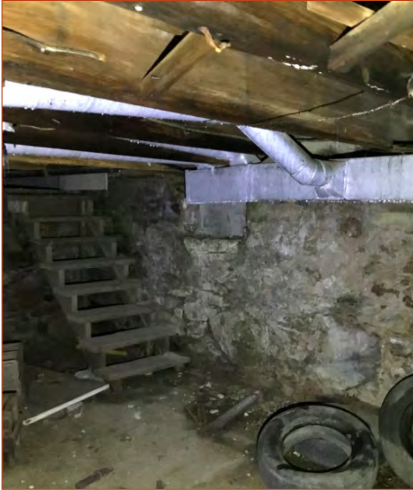
Figure 16: View of the basement (2020)
