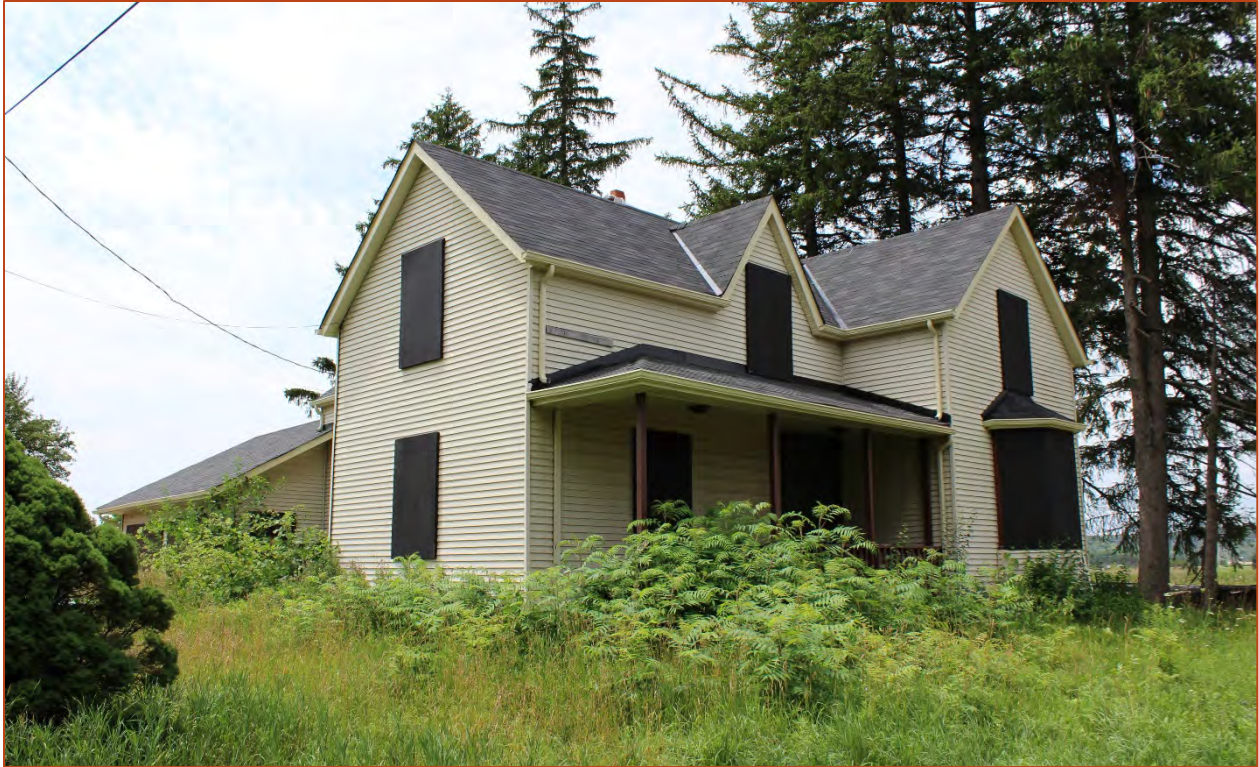
Figure 5: View west of the north and east elevations (2020)
