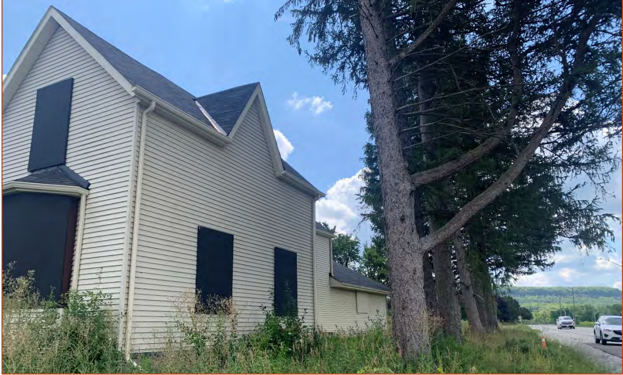
Figure 9: View southeast of the west elevation
