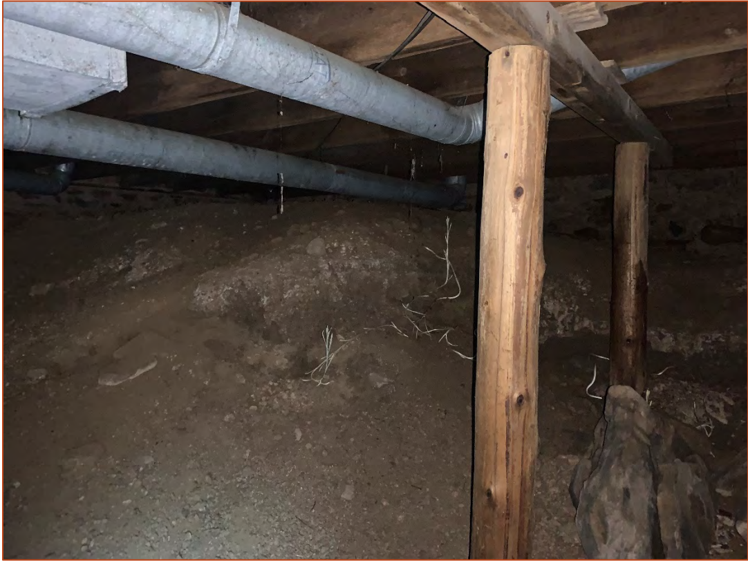
Figure 15: View of the crawlspace (Tacoma, 2020)
