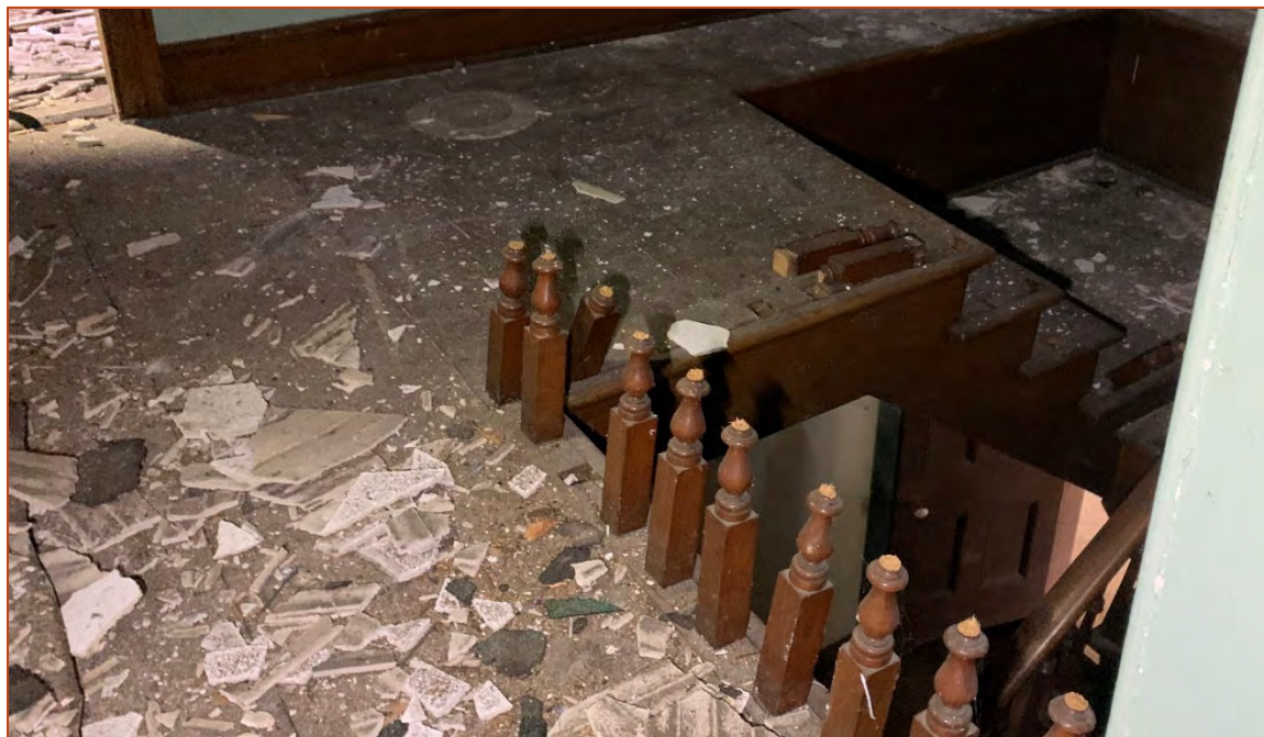
Figure 13: Second floor hall, front part of the house (2020)
