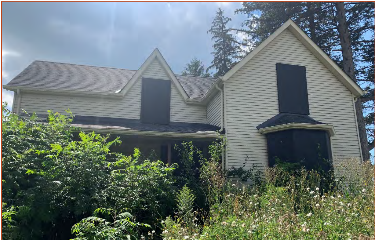
Figure 4: View southwest of the north elevation
