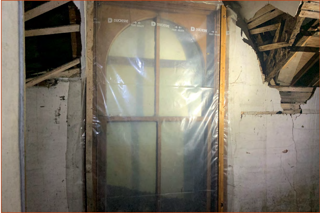
Figure 14: Second floor, semi-circular arched window
