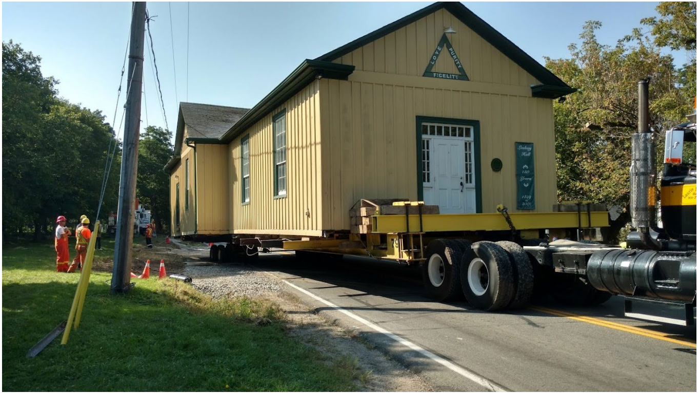
Similar frame heritage building on hydraulic dollies
