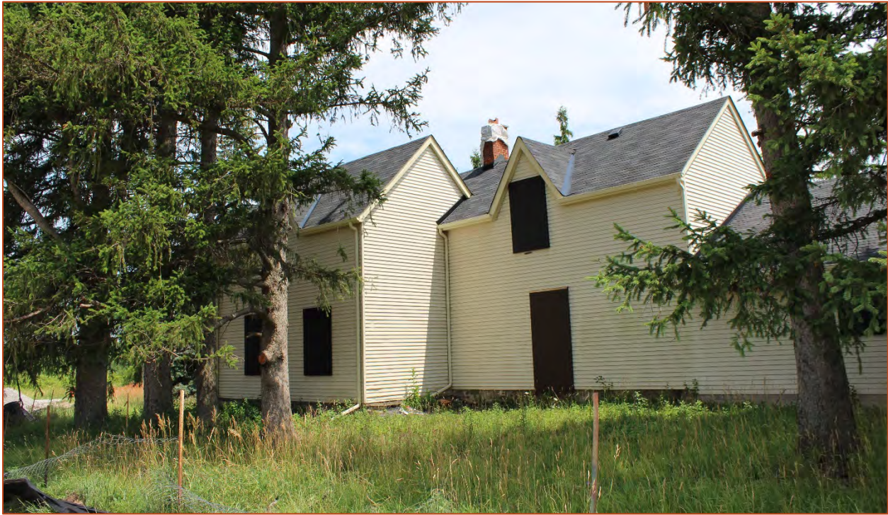
Figure 8: View southeast of the west elevation (2020)
