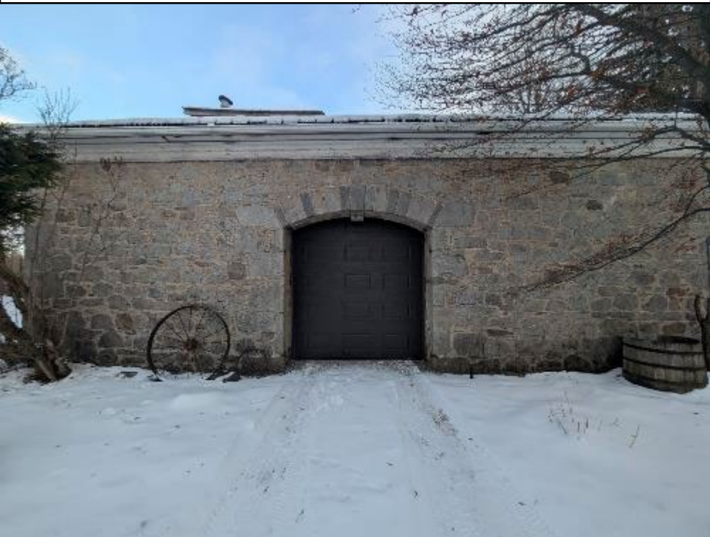
Dry Stone Shed
