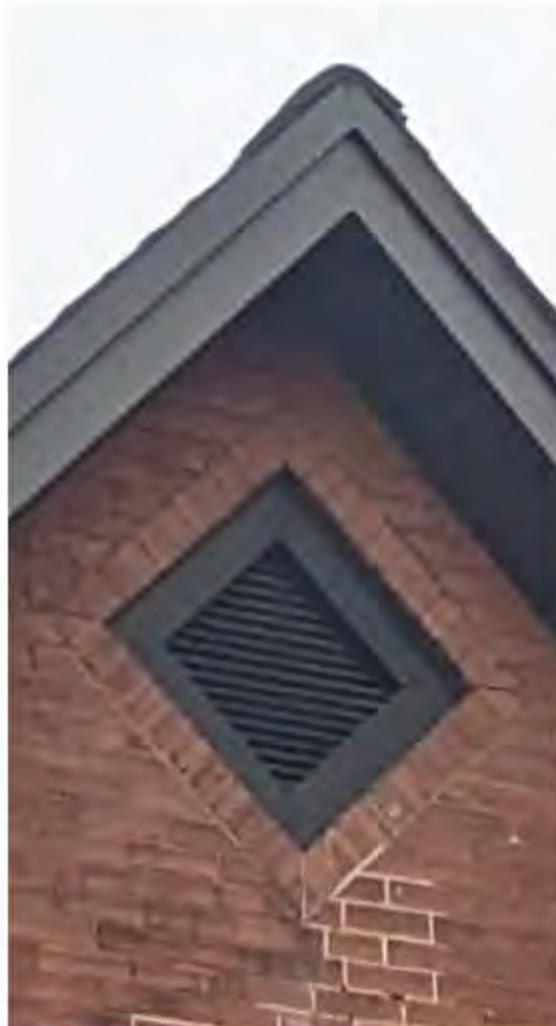
Diamond shape gable vent with plain moulding and brick surrounds
