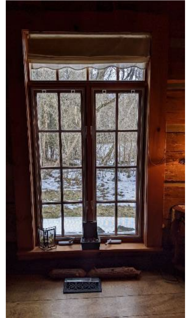
Pair of eight lite windows with four lite rectangular transom on the ground floor of the log house
