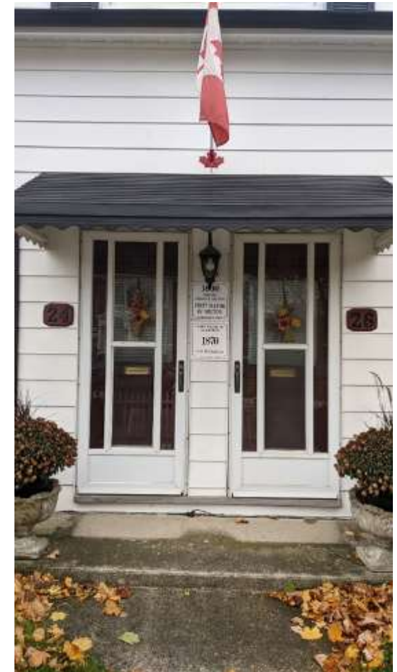
Two Entrance Door
