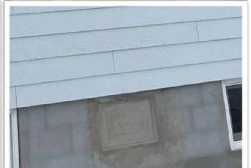
Location of Builder's engraving on North Elevation
