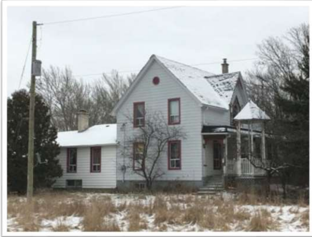
West and South Façade Before Rehabilitation
