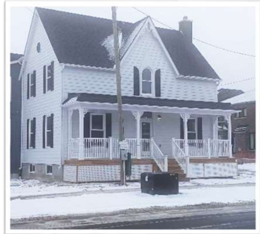
West and South Façade After Rehabilitation
