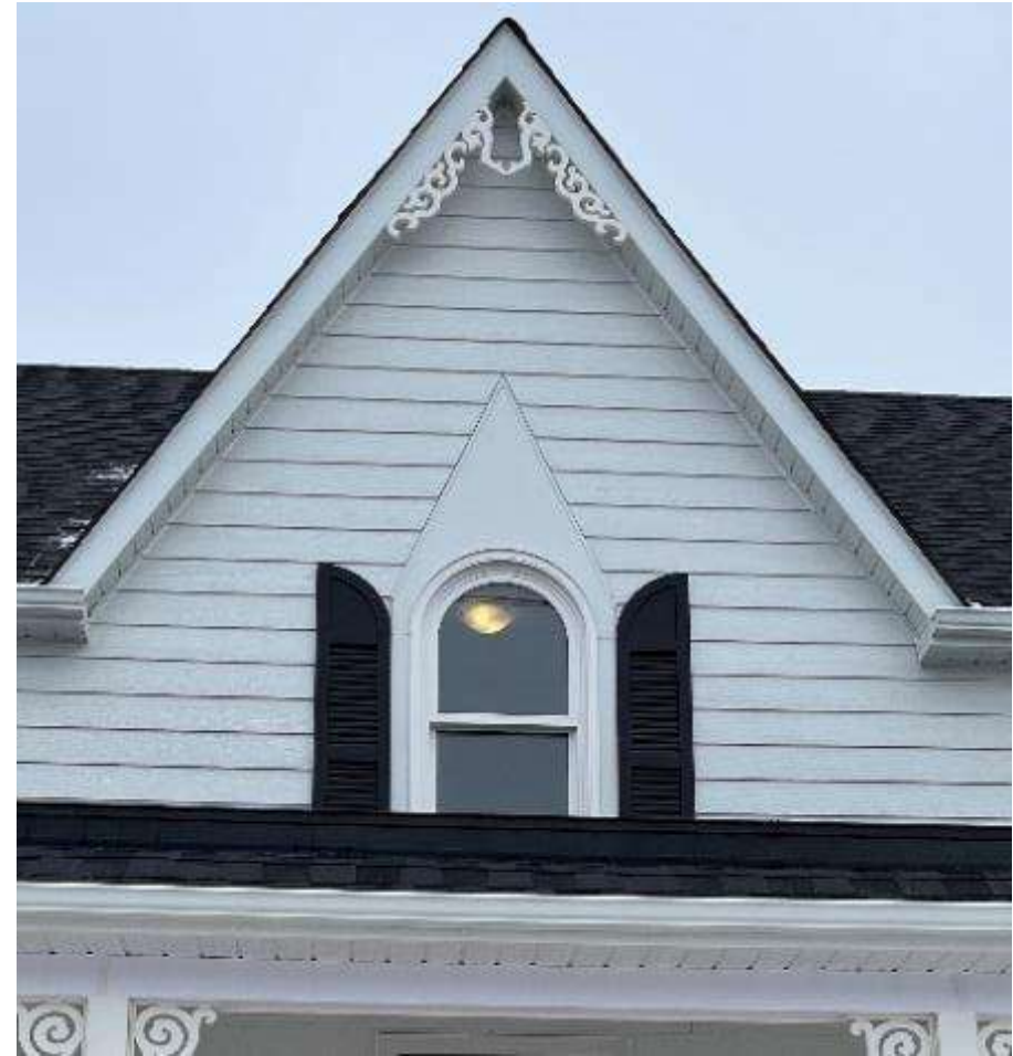
North East Façade After Rehabilitation
