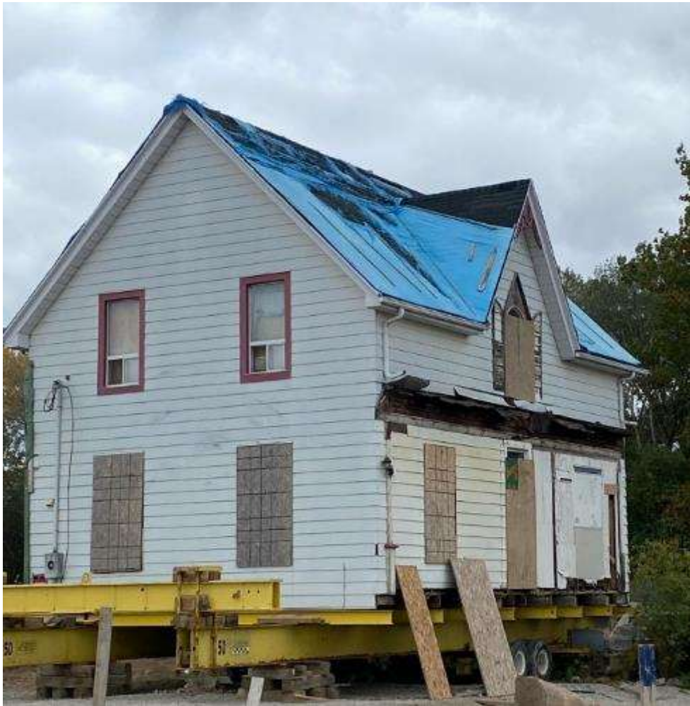
North Façade Before Rehabilitation
