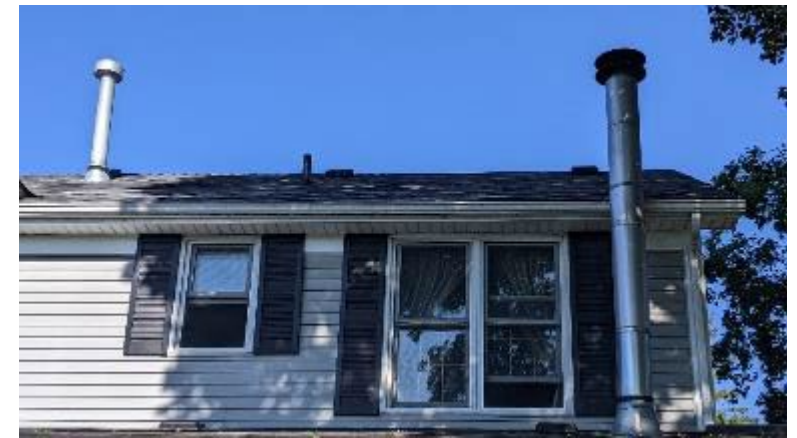
Second Floor Addition
