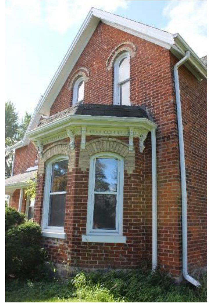
Bay Window at South Elevation
