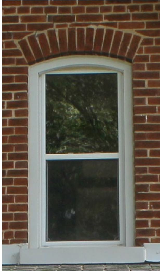
Window on Second Floor _ West Elevation
