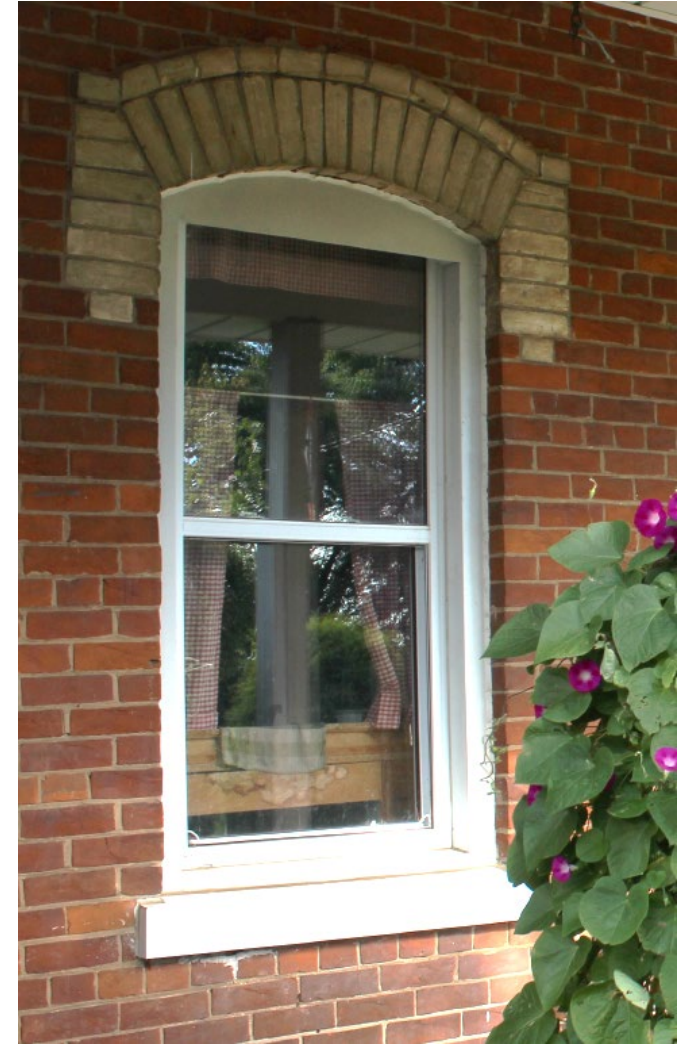
Window on Ground Floor _ East Elevation
