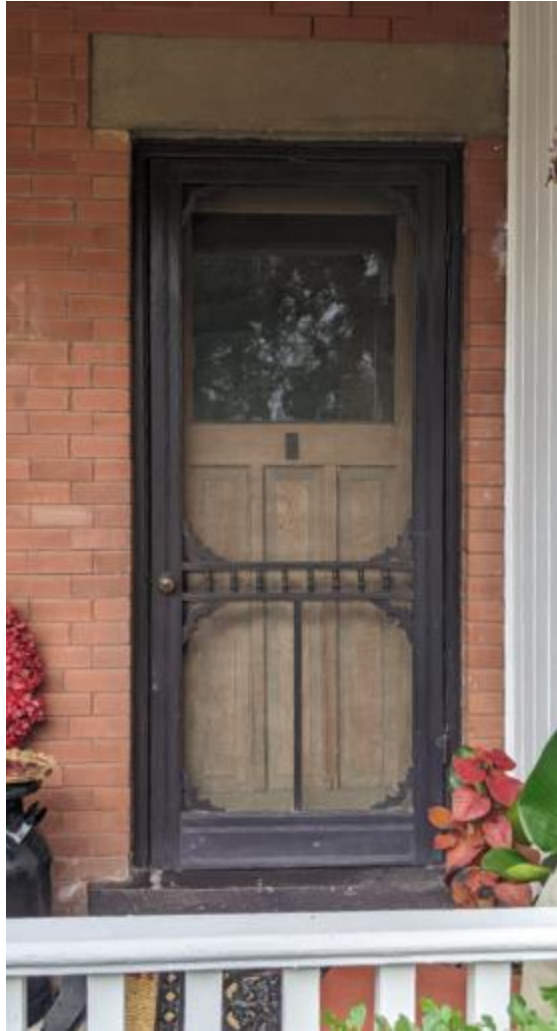
View of Door with Storm Door
