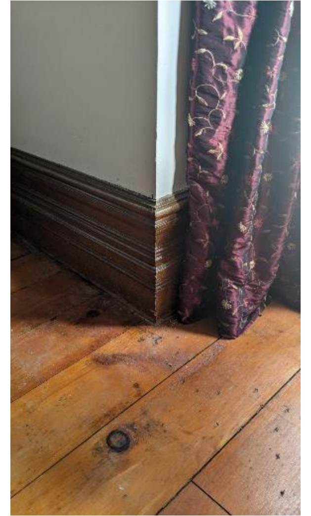
Original baseboard trims
