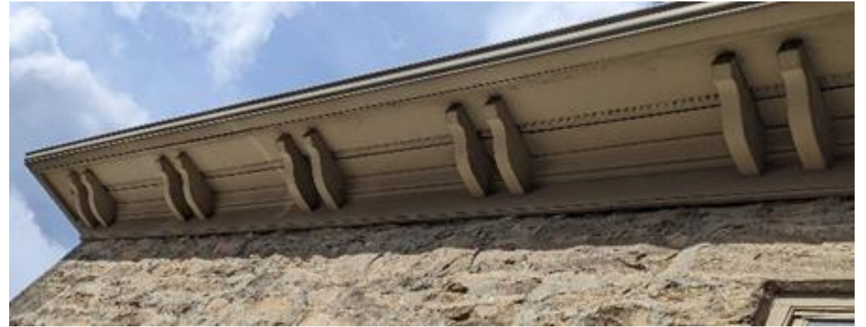
East Elevation Roof Cornices
