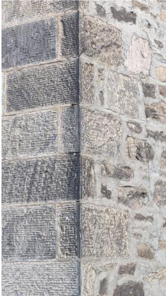
Detail at Corner
