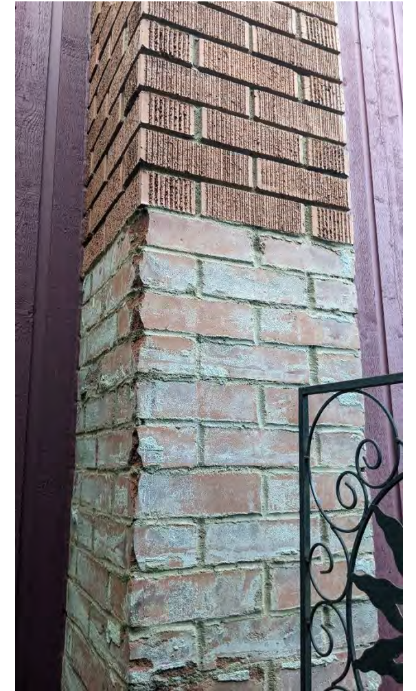
Brick Chimney Base
