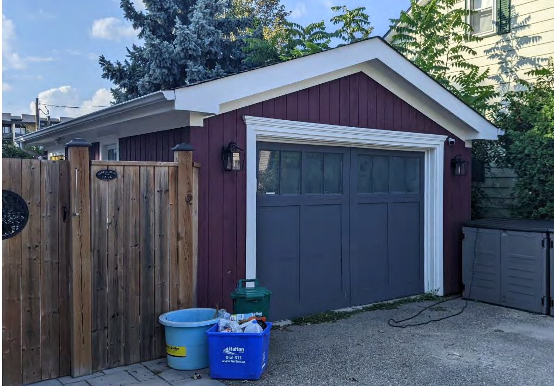
Existing Garage Non Heritage View along Pearl Street
