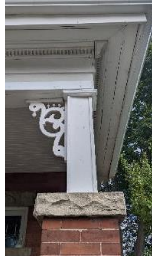
Wood post on brick piers
