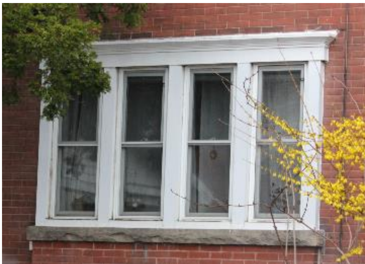
Gang of four one over one windows
