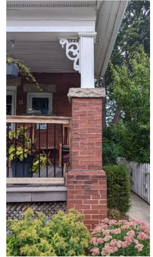
Wood post on brick piers
