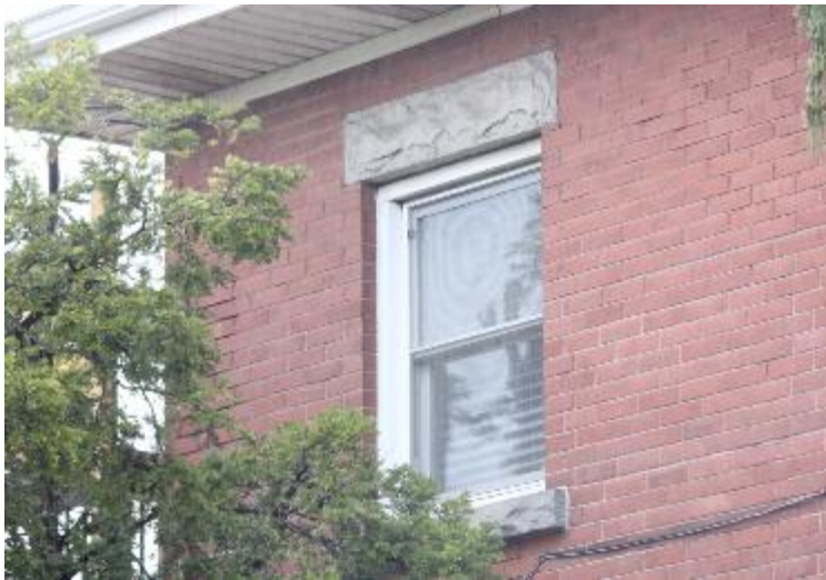
One over One window second floor
