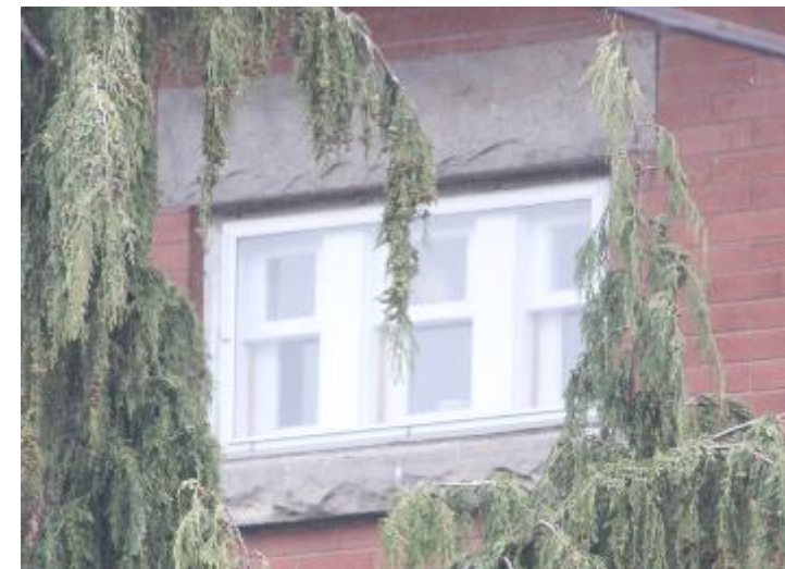
Gang of three one over one windows
