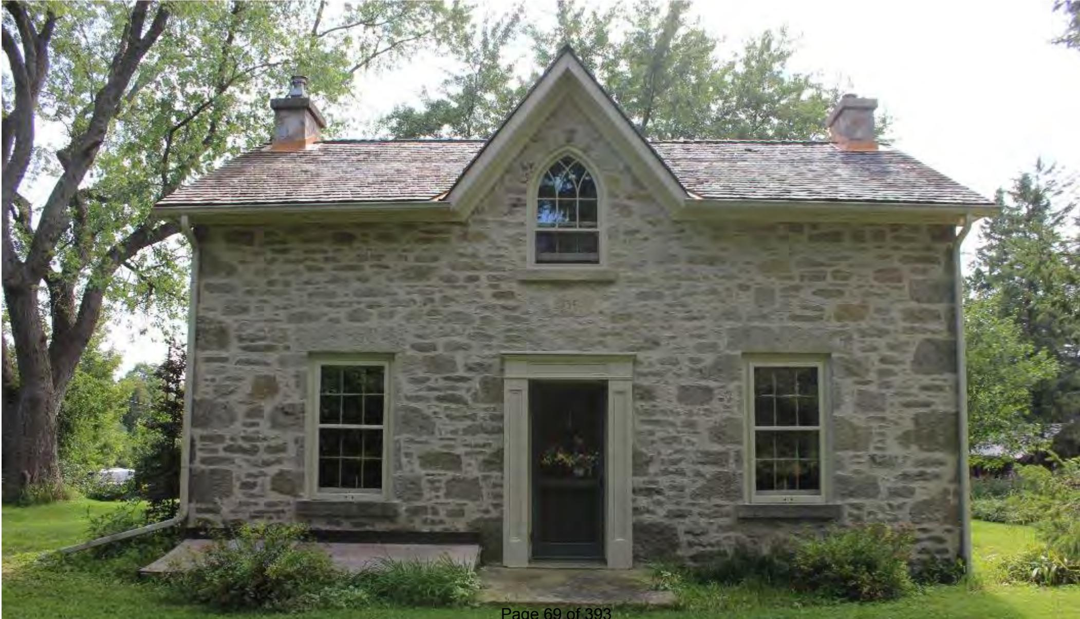
**East Elevation\_ Cedar Roof reinstallation, Cross Gable and Gothic window added 2014**
