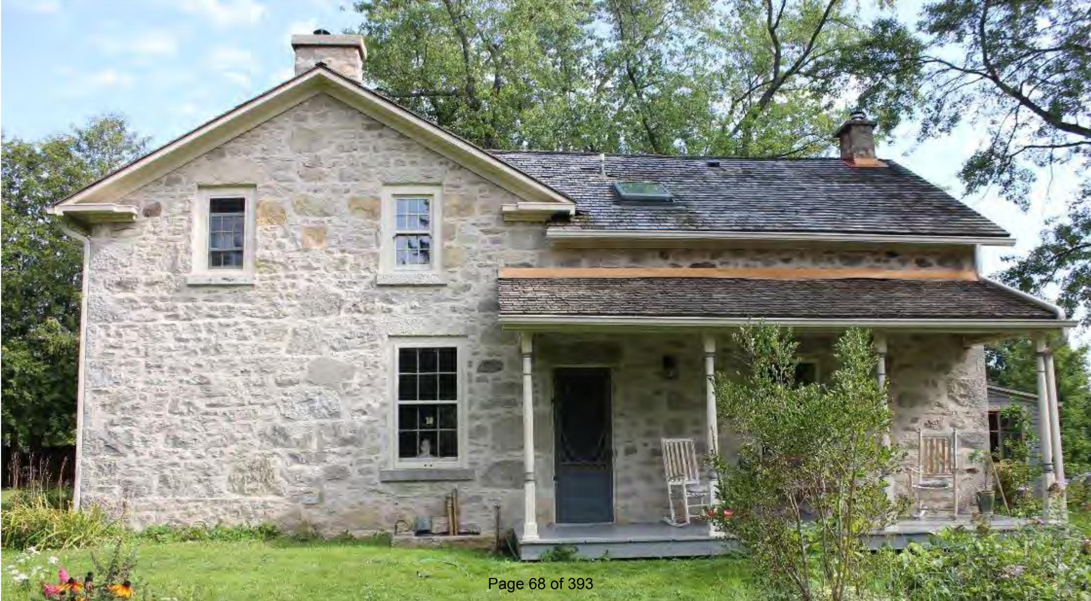
**North Elevation \_ Cedar Roof Replacement, Cross Gable and Gothic Window added 1984**
