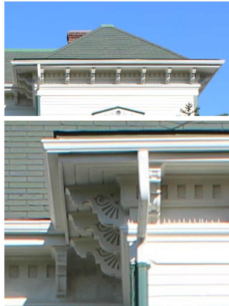
Hip roof with decorative eaves bracket
