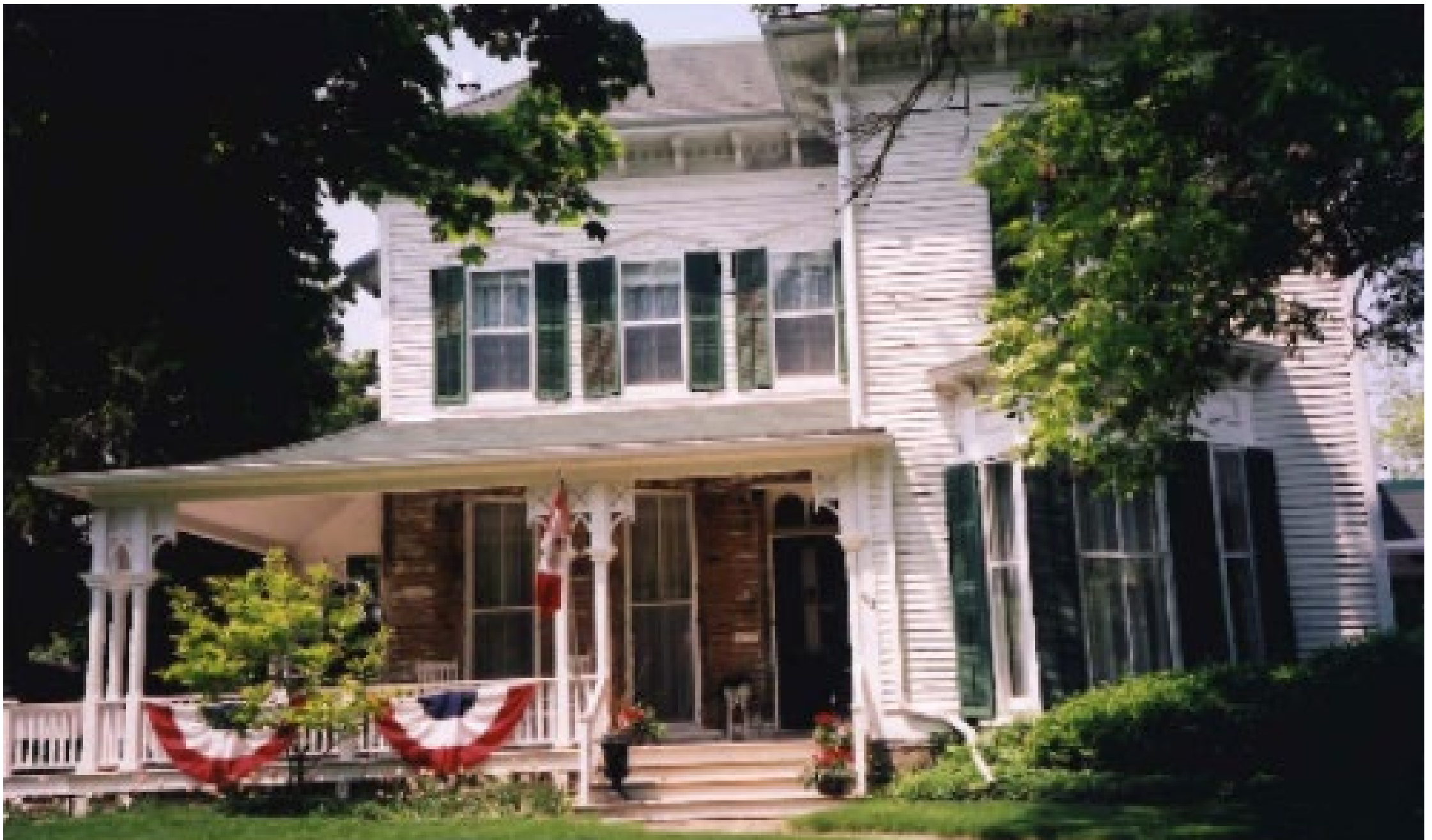
Page 77 of 546 Front Porch Restoration
