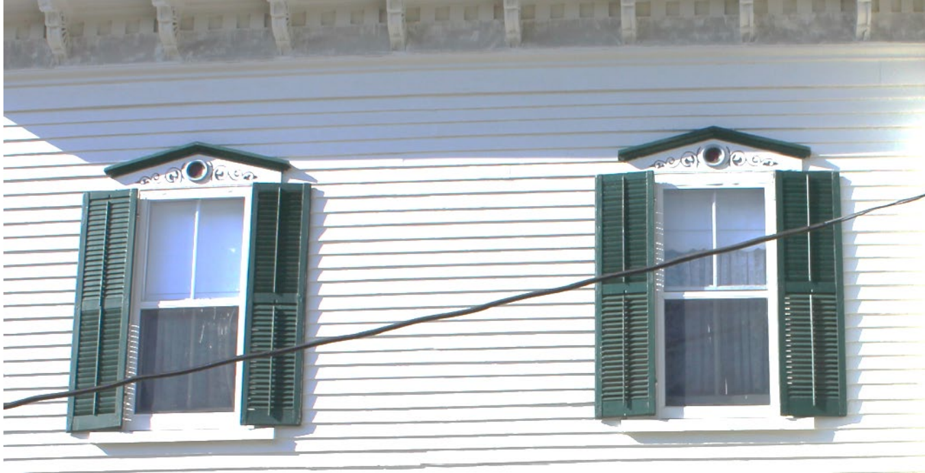
Second Floor East Elevation Window
