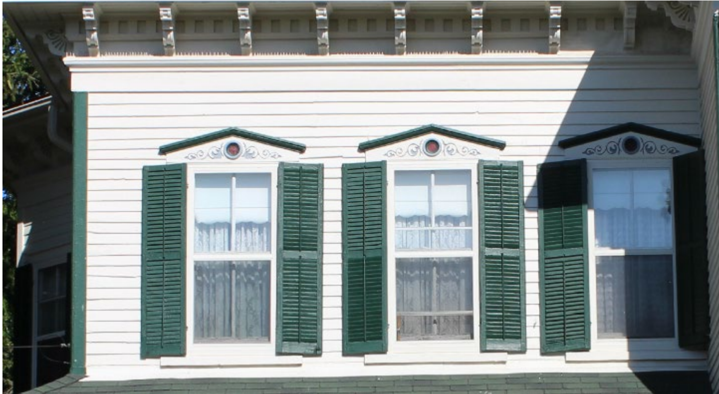
Second Floor Windows _ Front Elevation
