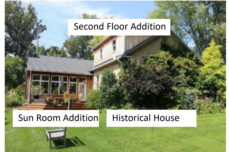
Rear sun room addition
