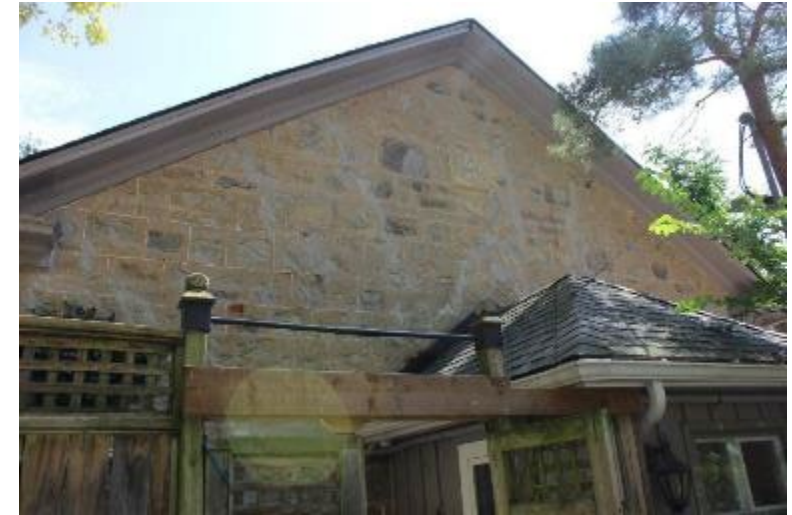
Medium gable roof on top of original stone.
