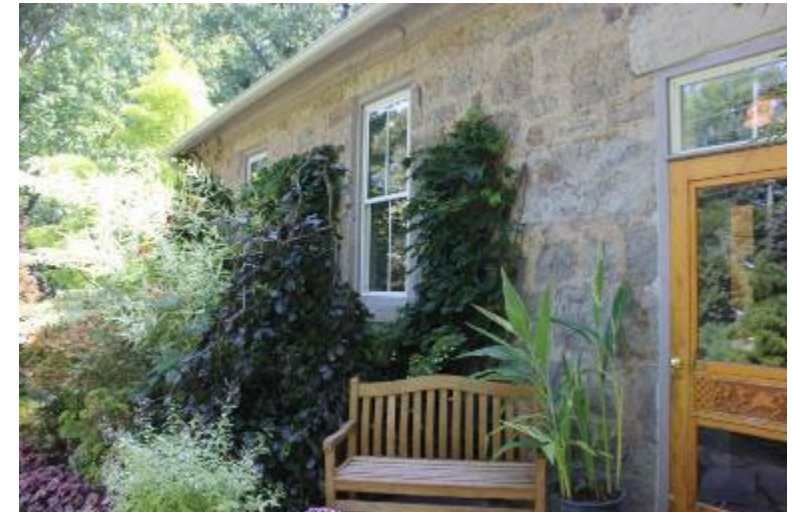
Stone wall at front elevation
