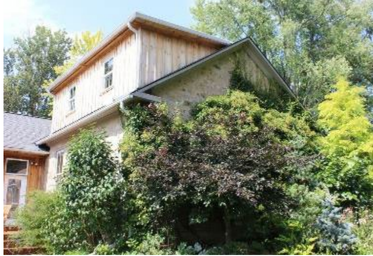
Second floor addition at rear
