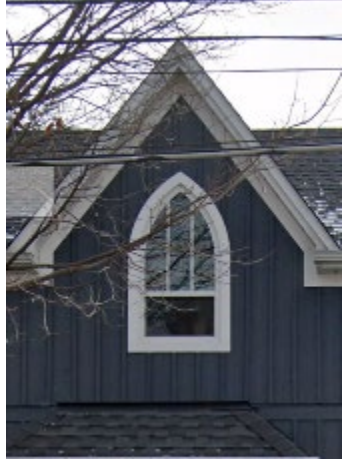
Central Gable Gothic Window
