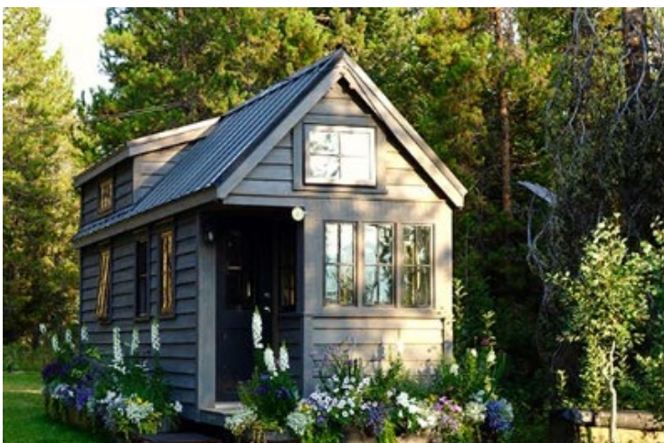
Figure 18. Example of Additional Residential Unit (City of Brampton, n.d.).
