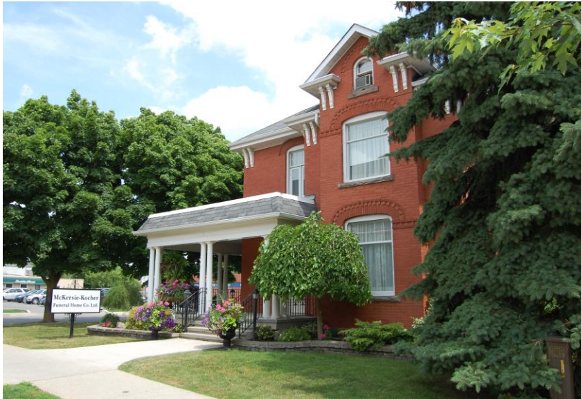
Figure 142 – 114 Main Street East (Photo: RHC, June 2014)
