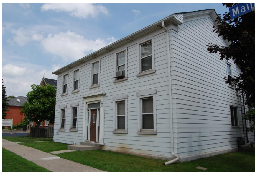
Figure 141 – 94 Main Street East (Photo: RHC, June 2014)
