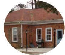
c) Original window and door openings, 6 over 6 windows with limestone sills and panel doors.
