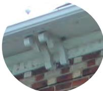
c) Hand-made bricks laid in Common and Flemish bond patterns, beaded mortar and contrasting buff brick detailing.
