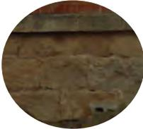
e) Hand-made bricks laid in Common and Flemish bond patterns with brick voussoirs.
