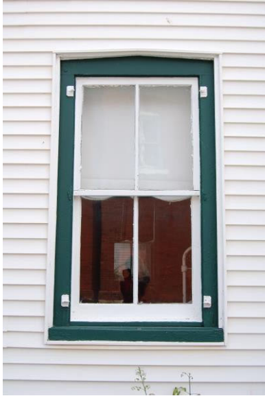
Original wood cladding with 2 over 2 windows
