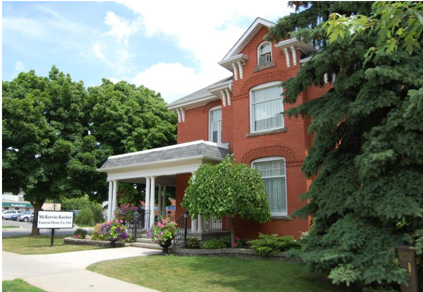
Figure 142 – 114 Main Street East (Photo: RHC, June 2014)
