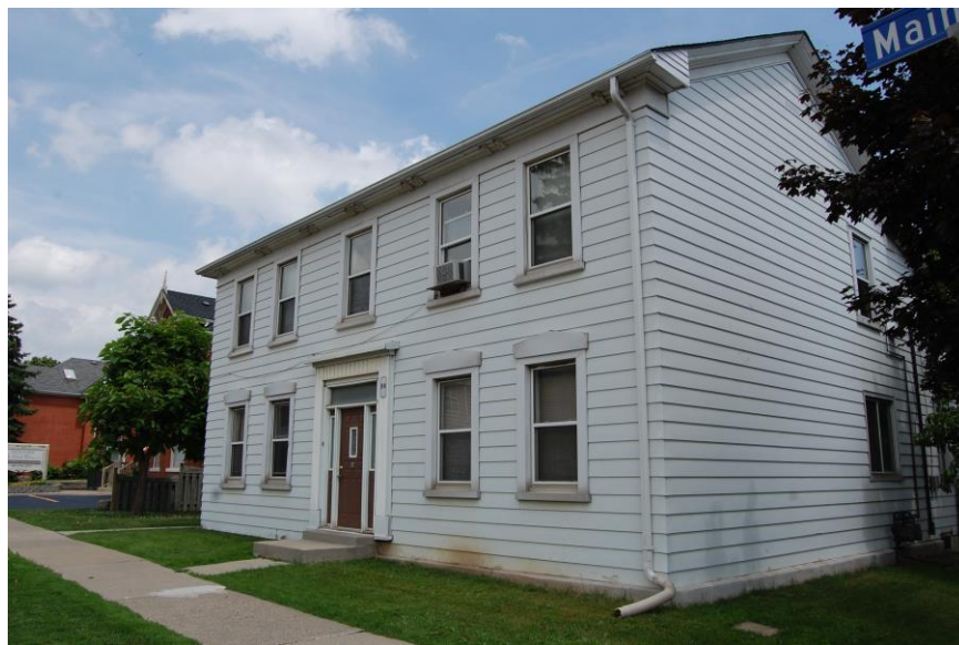
Figure 141 – 94 Main Street East (Photo: RHC, June 2014)
