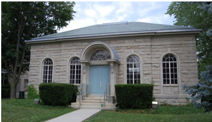
Figure 146 – 141 King Street (Land Registry Building) (Photo: RHC, June 2014)
