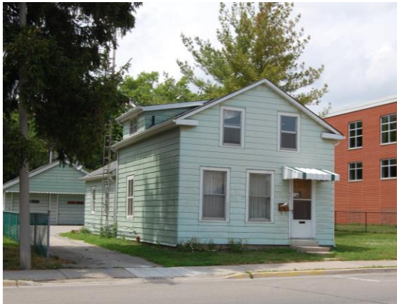
Figure 143a – 101 Main Street East (Photo: RHC, June 2014)
