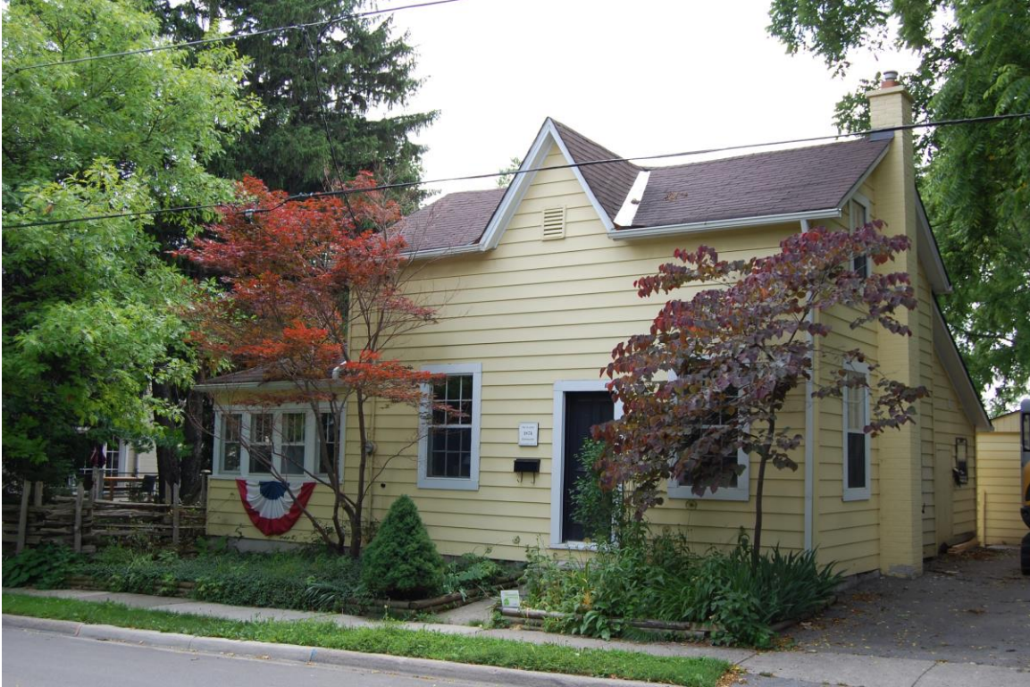
Figure 149 – 48 Bell Street (Photo: RHC, June 2014)
