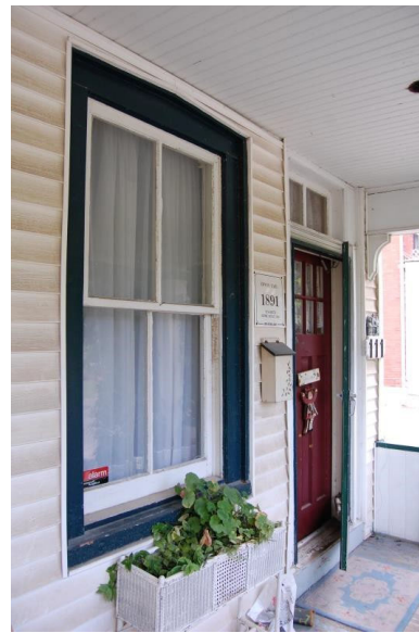
Original window and door elements of the original house (front and sides of the main block and kitchen tail) including their pedimented heads.
