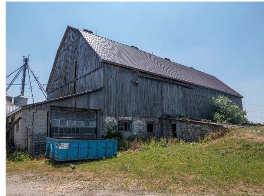
Figure 8: Looking southwest at the two-storey barn, showing raised embankment to the second storey entrance and shed roof addition at the left.
