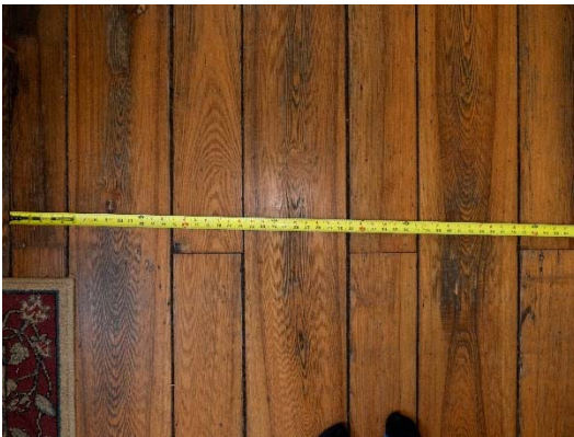
Figure 25: Hardwood flooring in the kitchen is of varying widths.
