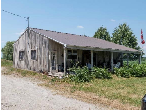
Figure 5: The one-storey wood shed is northwest of the farmhouse, and was originally constructed as a farm store.
