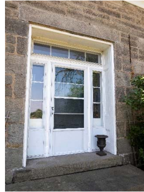
Figure 16: The main entrance door is recessed and set within sidelights and a transom.
