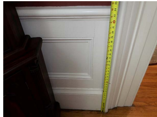
Figure 28: Typical wainscoting in the dining room is an embellishing version of that in the kitchen.
