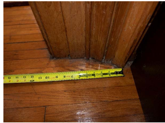
Figure 26: The profile of the typical Grecian ogee is seen in the living room, roughly between the 1 1/4" and 4 3/4" marks on the tape measure.
