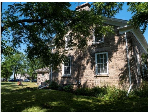
Figure 13: The south elevation mirrors the north elevation at the house's front portion.
