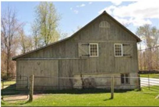
Rubble Wall foundation and vertical barn boards and batten siding
