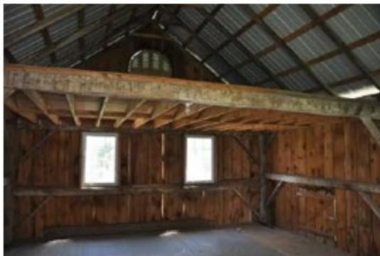
Square log timber framing, which is exposed to the interior
