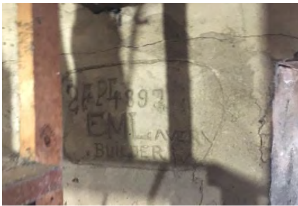
Builder's engraved marking of - "SEP 24 1897, E. M. Laver Builder" in basement
