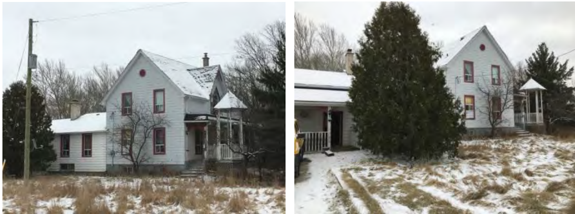
Figure 8: North-east (left) and north-west (right) views of residence building [AREA, 2018]
