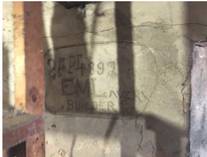
Figure 22: Builder's engraved marking in basement– “SEP 24 1897, E.M.Laver Builder”
