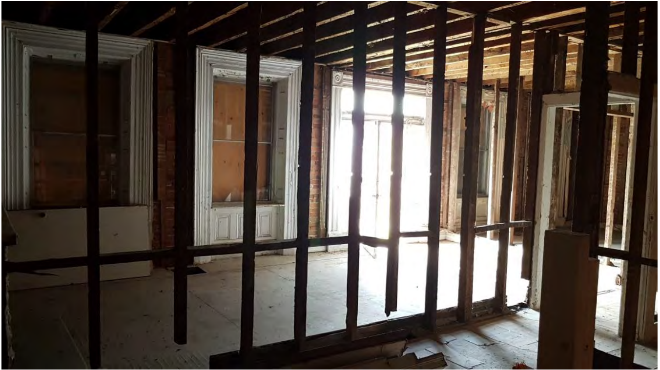
Figure 29: View of main entrance and four windows from southeast corner.
