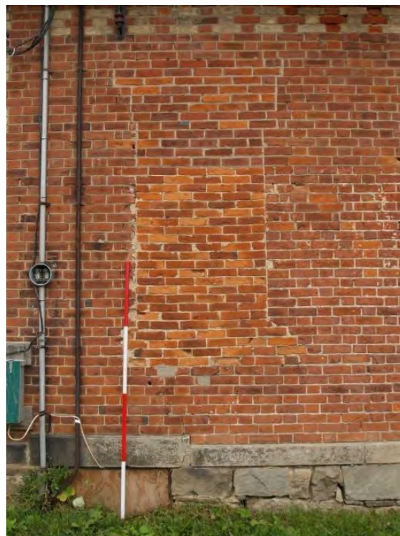
Figure 24: Blind window on south end wall (August 2018)
