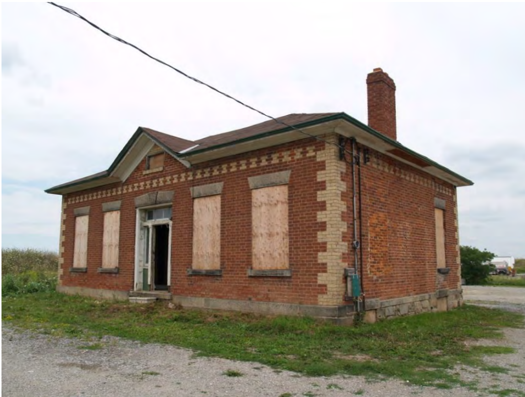
Figure 7: West façade and south end wall (August 2018)
