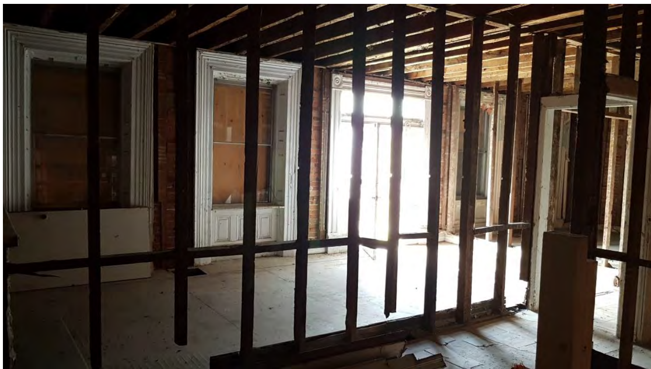
Figure 29: View of main entrance and four windows from southeast corner.
