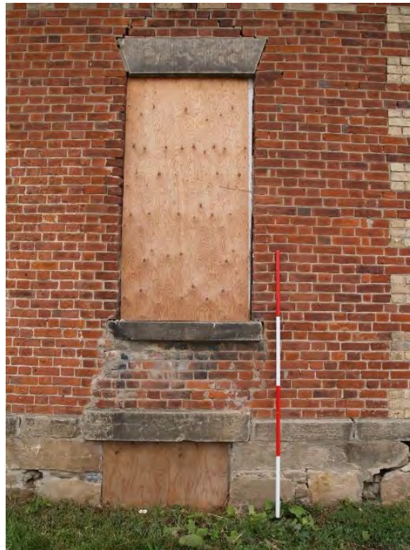
Figure 23: Typical window on the south end wall (August 2018)
