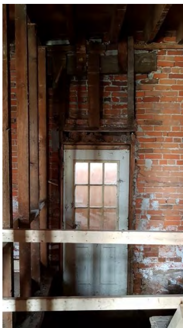
Figure 34: Rear vestibule with door and access to basement.
