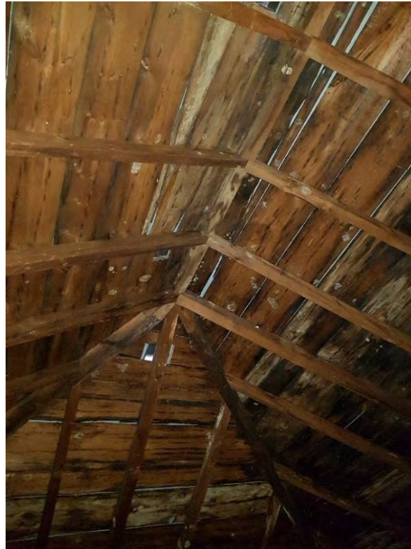
Figure 41: Rafter roof (August 2018)
