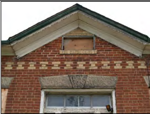
Cross gable with curvilinear verge board
