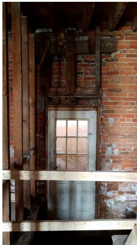
Figure 36: Rear vestibule with door and access to basement (August 2018)
