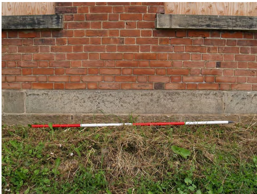
Figure 20: Ashlar stone top course.
