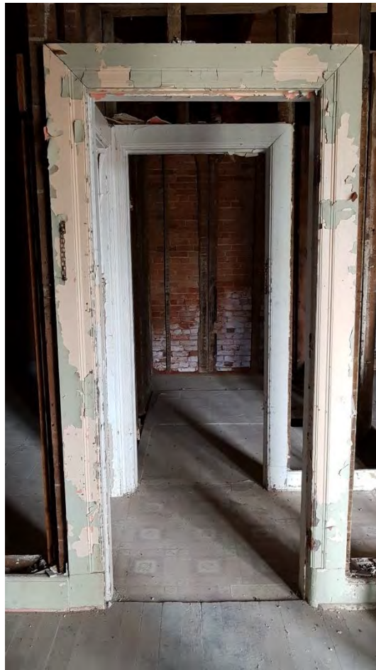
Figure 32: Central hallway facing east.
