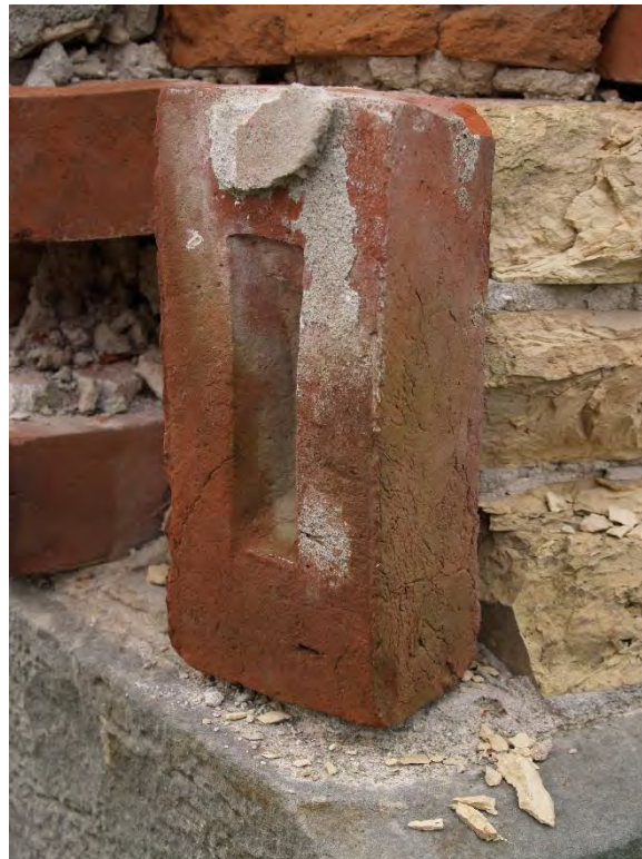
Figure 15: Frogged brick found at the northeast corner (August 2018)
