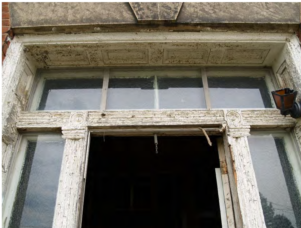
Figure 26: Entrance with wood lintel, pilasters with rosettes, transom, and panelled architrave (August 2018)
