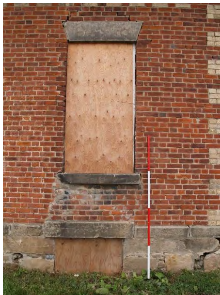
Figure 24: Covered window on south façade.
