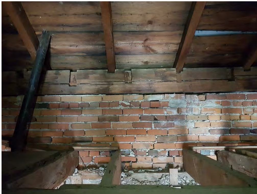
Figure 42: Redundant mortices in wood beams of roof (August 2018)
