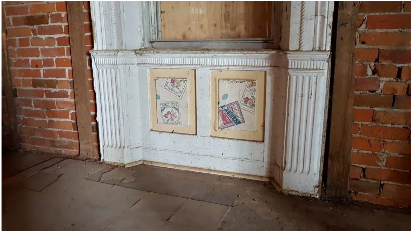
Figure 33: Window with trim and panelling along the south wall.
