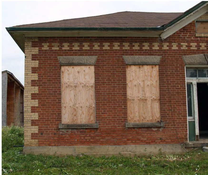
Figure 17: Flemish bond red brick with buff brick quoins and band on the west façade (August 2018)
