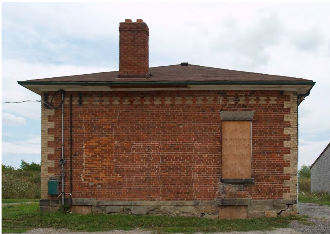
Figure 8: South end wall (August 2018, corrected for distortion)
