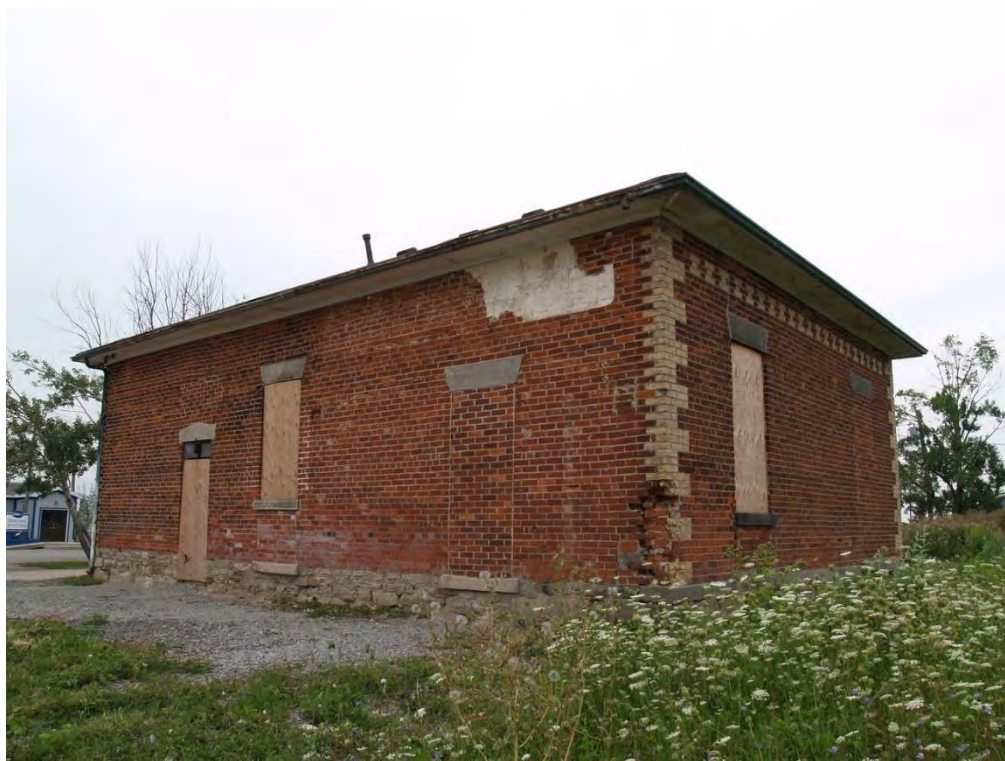
Figure 15: East and north façades.
