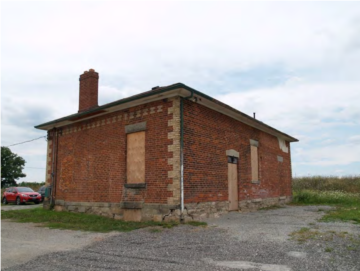
Figure 9: South end wall and east façade (August 2018)
