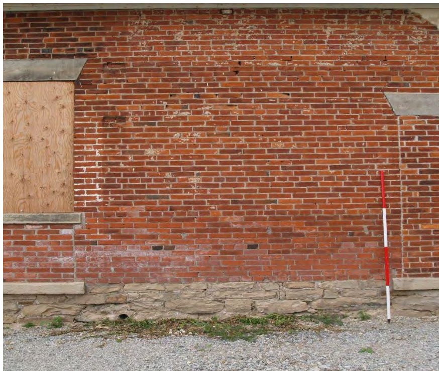
Figure 18: Five-in-one American or common bond masonry of the east façade (August 2018)
