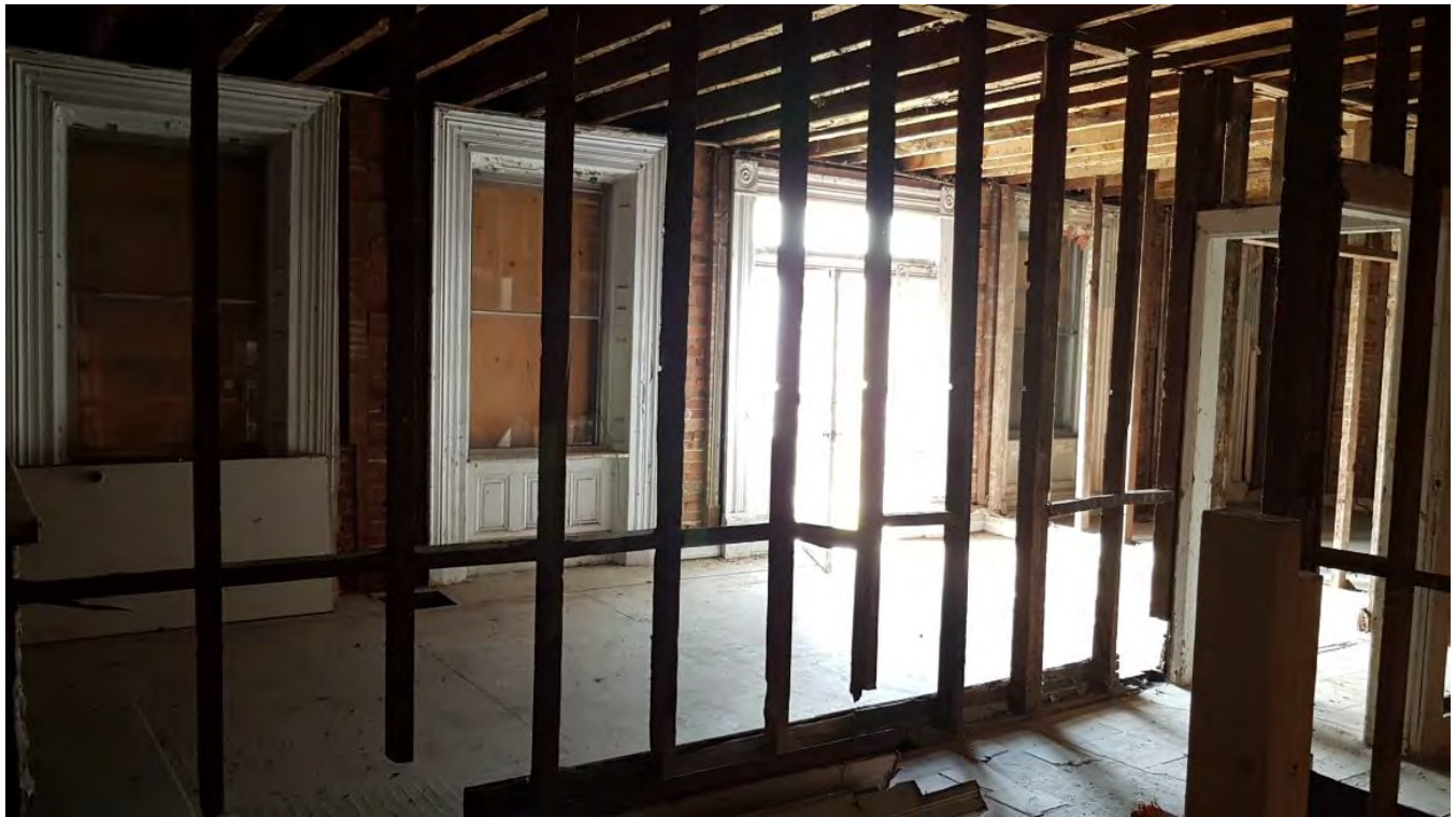
Figure 31: View of main entrance and four windows from southeast corner (August 2018)
