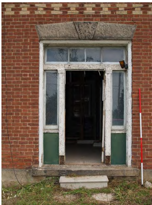
Figure 25: Front door with sidelights, transom and stone lintel with mock keystone.
