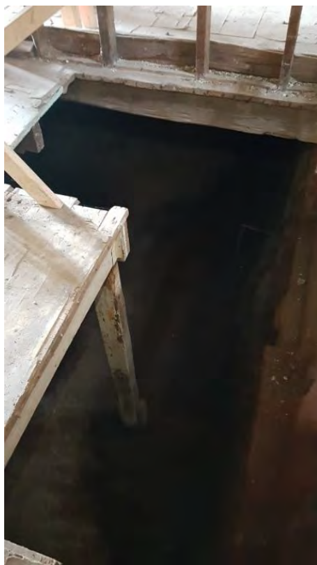
Figure 35: View of basement from main storey.
