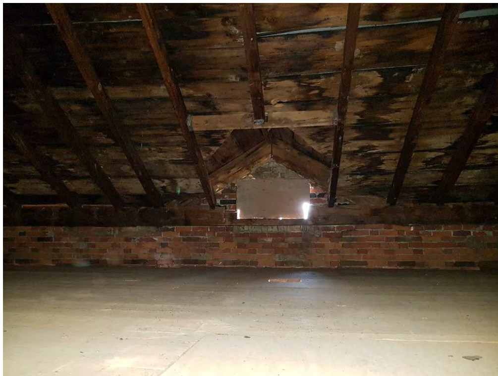
Figure 38: Attic with blind window in the cross gable.
