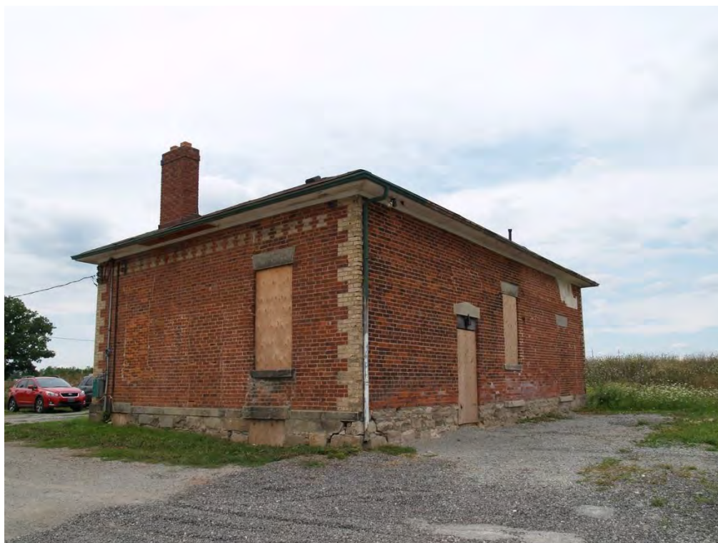
Figure 13: South and east façades.
