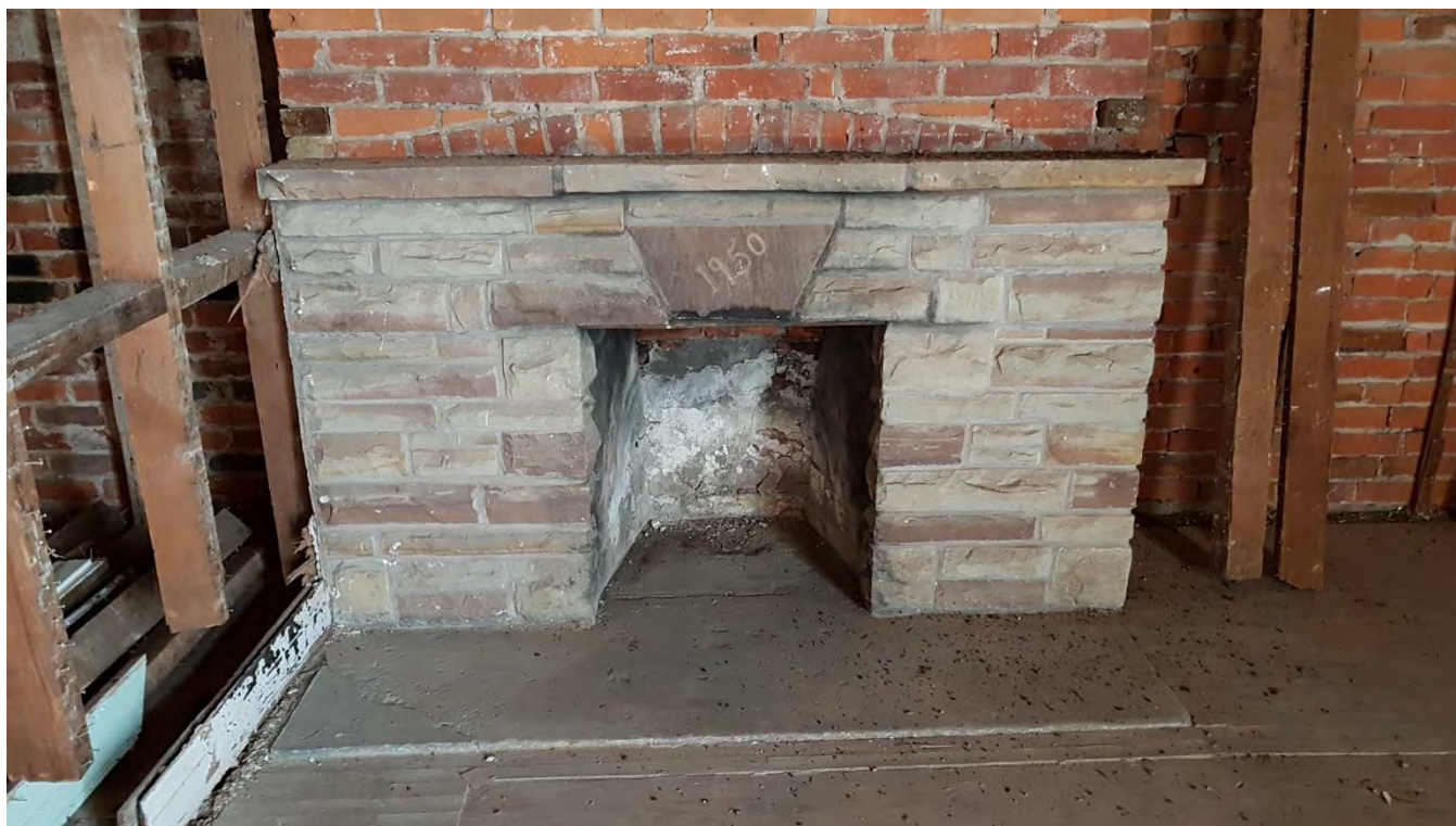
Figure 31: Fireplace on south end wall with 1950 datestone on the stone veneer.
