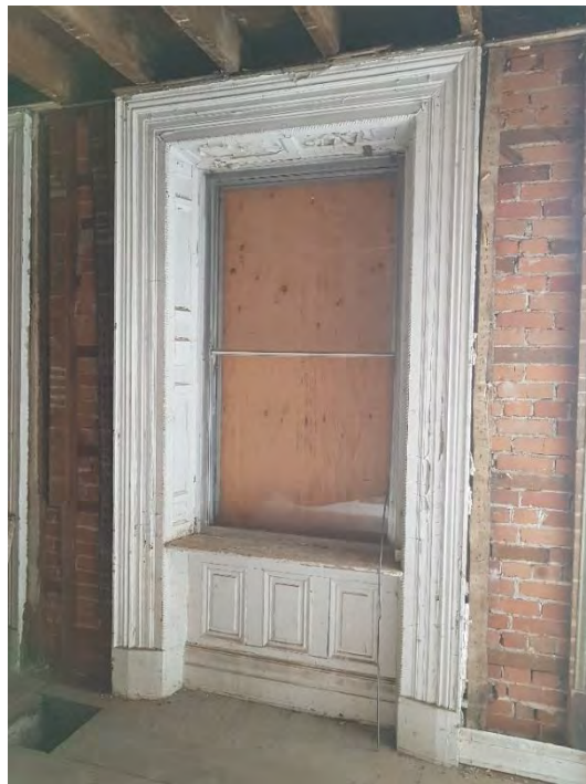
Figure 30: West wall window with moulded casing and trim.
