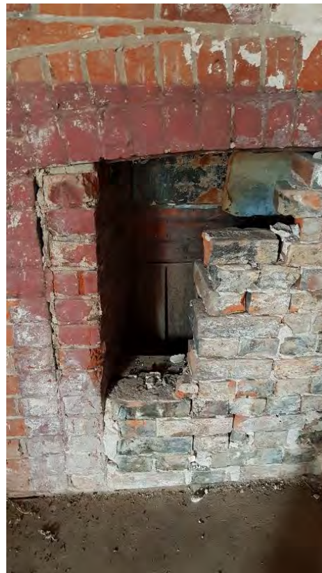
Figure 39: Exposed fireplace, partially filled in with brick (August 2018)
