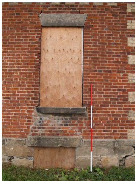
Figure 24: Covered window on south façade.
