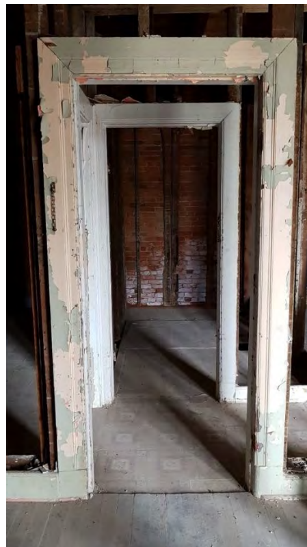
Figure 34: Central hallway facing east (August 2018)
