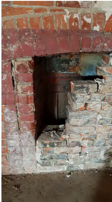
Figure 37: Exposed fireplace, partially filled in with brick.
