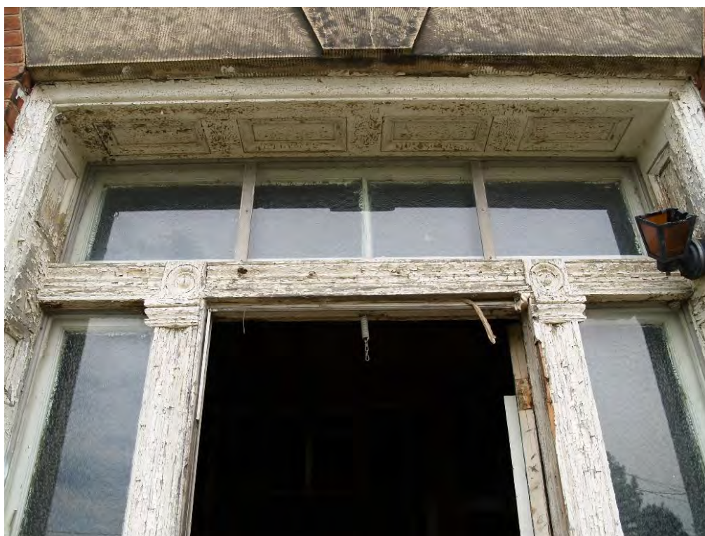
Figure 26: Front door showing wood detailing.
