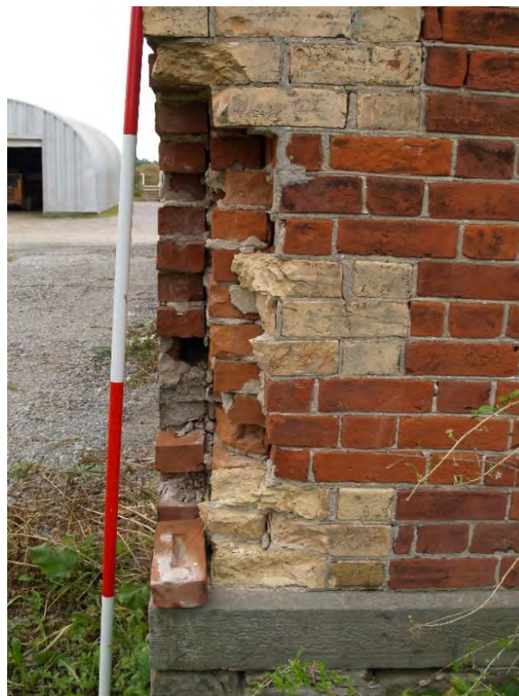
Figure 16: Double wythe construction exposed at the northeast corner (August 2018)
