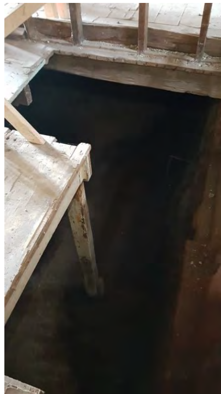
Figure 37: View of basement from main storey (August 2018)
