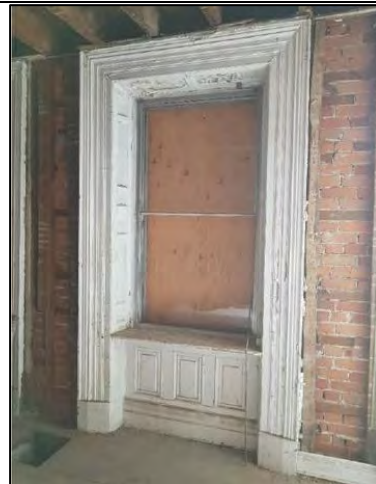
West wall window with moulded casing and trim
