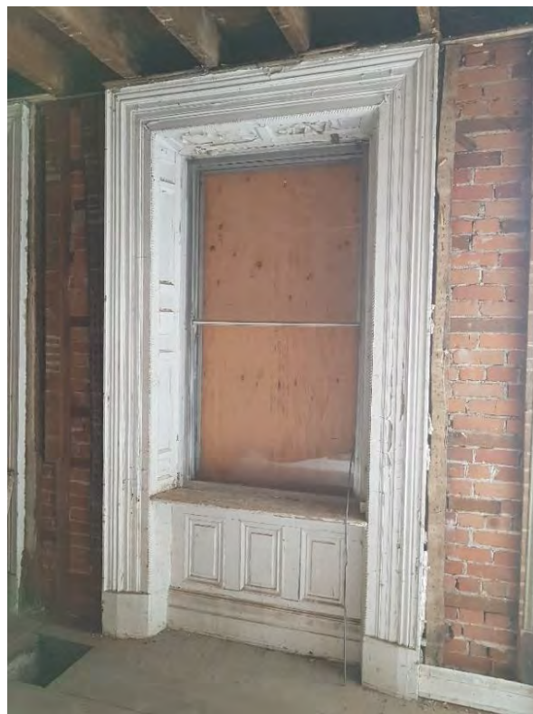
Figure 32: West wall window with moulded casing and trim (August 2018)
