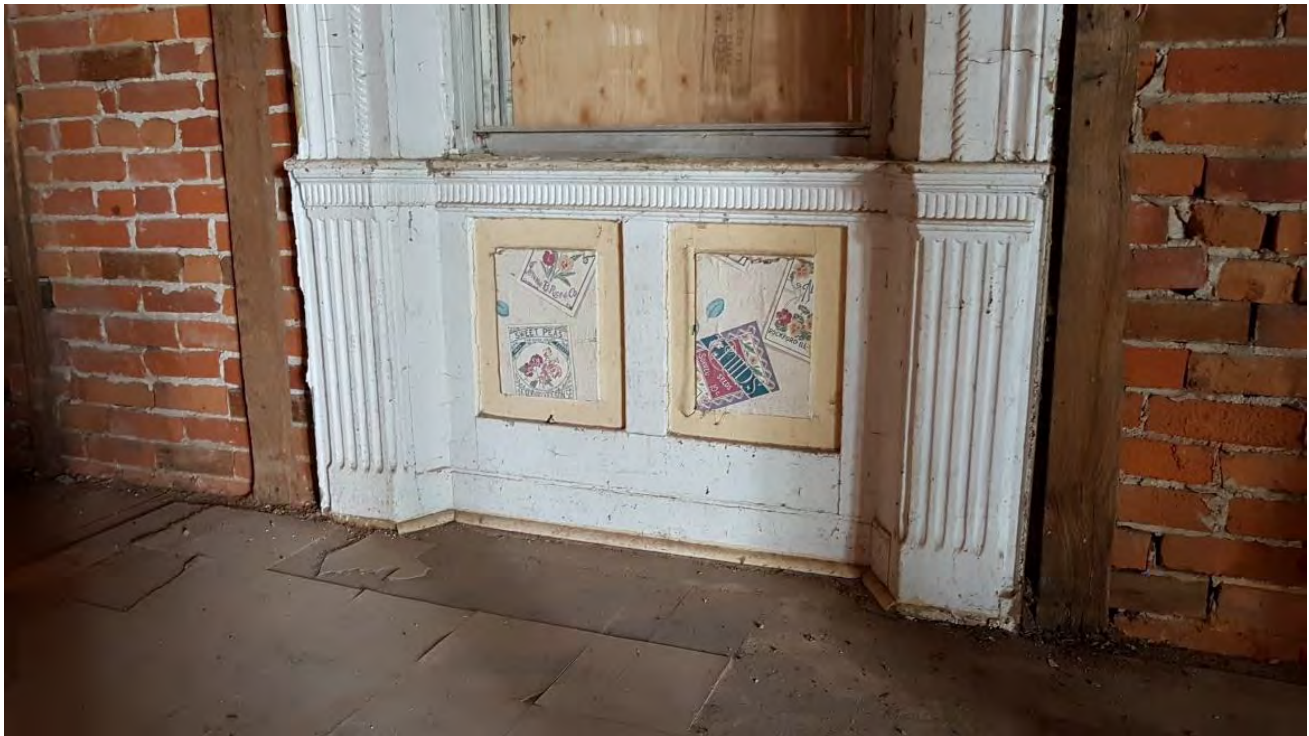
Figure 35: Window with trim and panelling along the south wall (August 2018)
