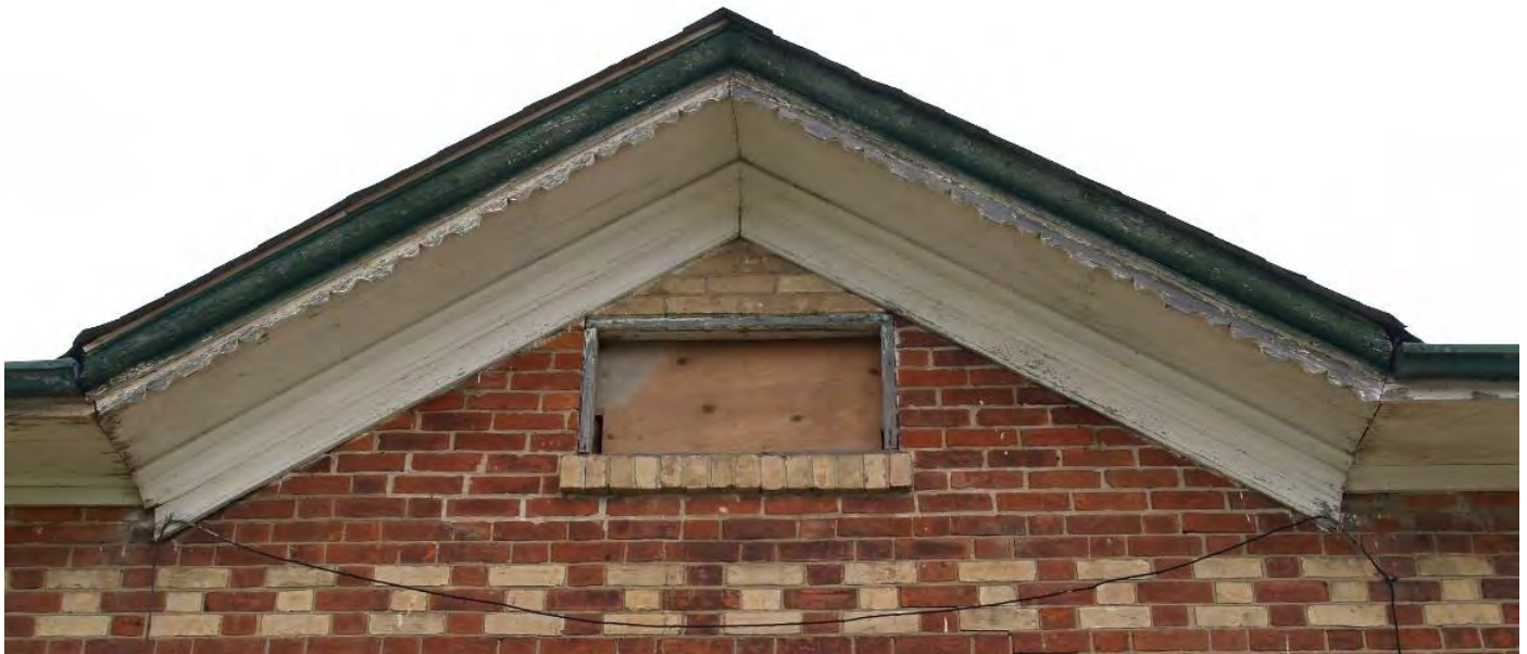
Figure 21: Central cross gable with moulded soffit, fascia, and narrow curvilinear vergeboard. Also shown is the buff brick in the apex of the gable can also be seen (August 2018)
