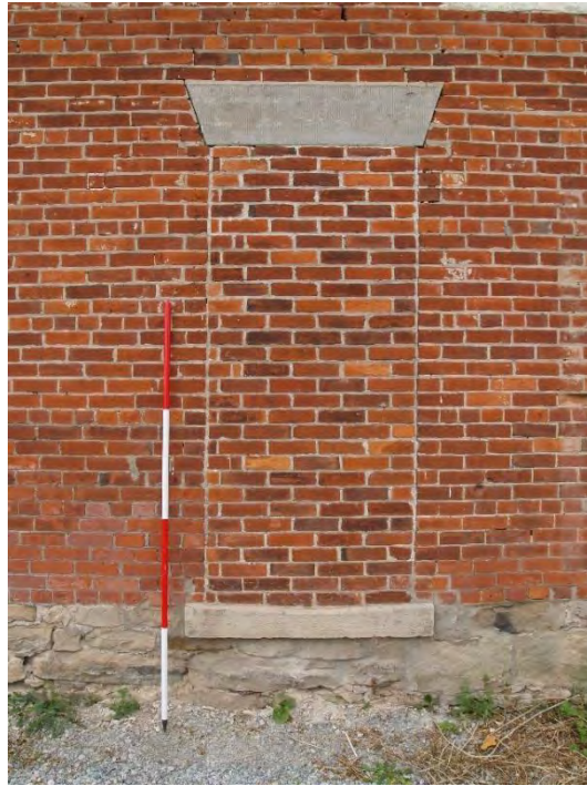
Figure 27: Blind entrance on east façade.
