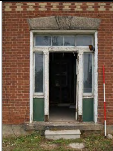
Front door with sidelights, transom and stone lintel with mock keystone
