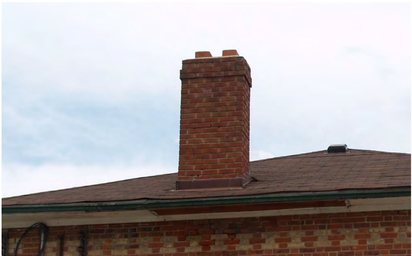
Figure 22: Brick chimney inside the south end wall (August 2018)
