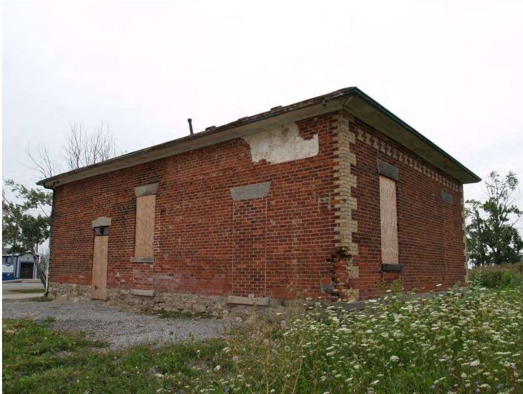
Figure 11: East façade and north end wall (August 2018)
