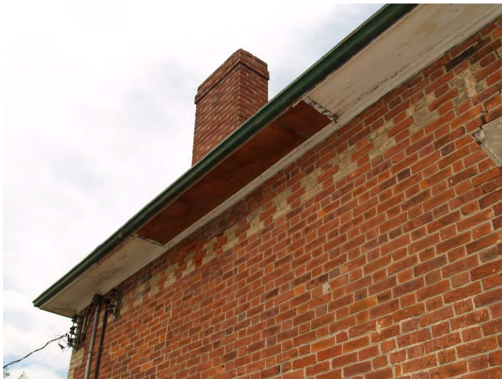
Figure 22: Brick chimney, with projecting eaves and plain soffit.
