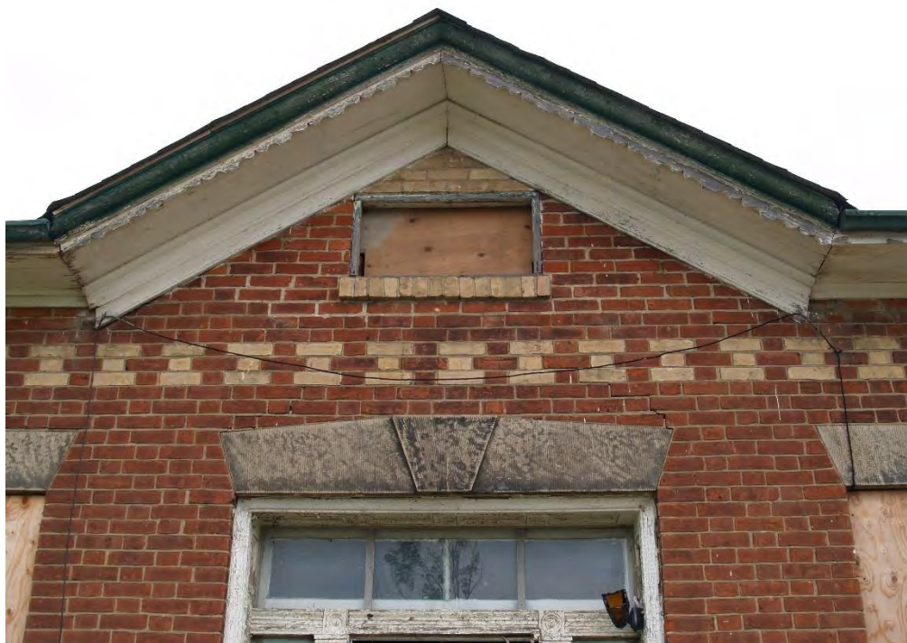
Figure 21: Cross gable with curvilinear vergeboard
