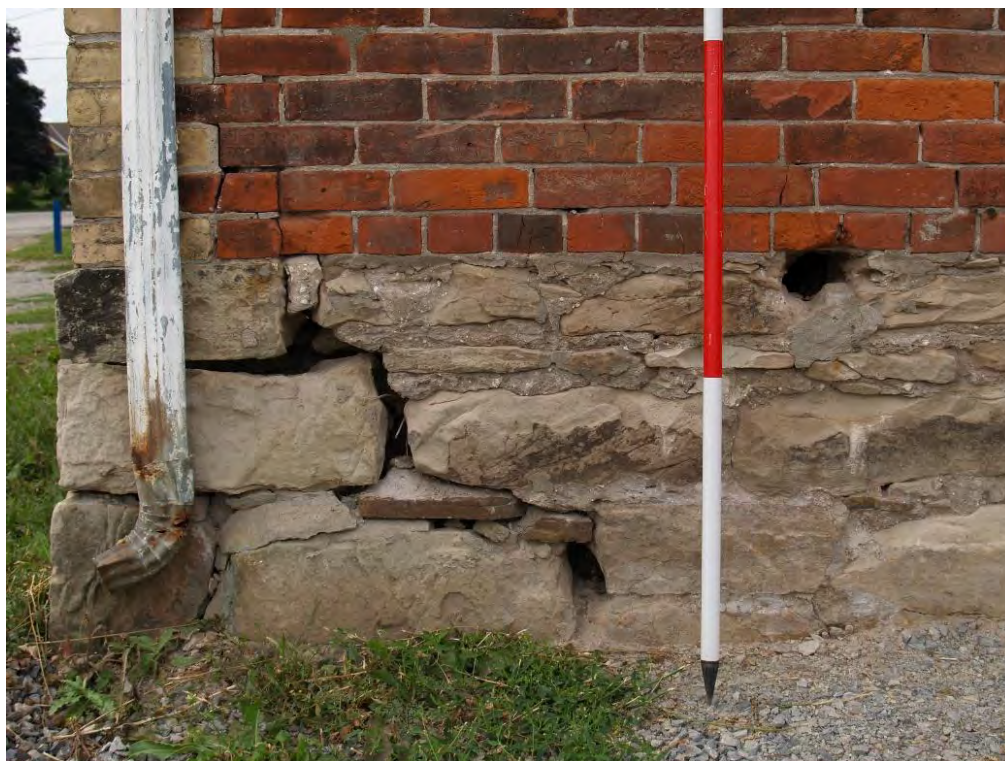
Figure 17: Stone foundation on the east façade.
