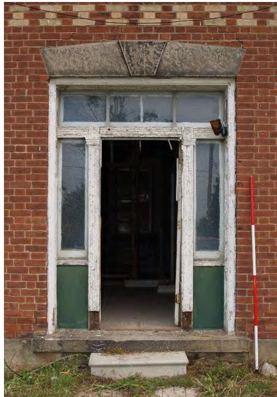
Figure 25: Front door with sidelights, transom and stone lintel with mock keystone (August 2018)
