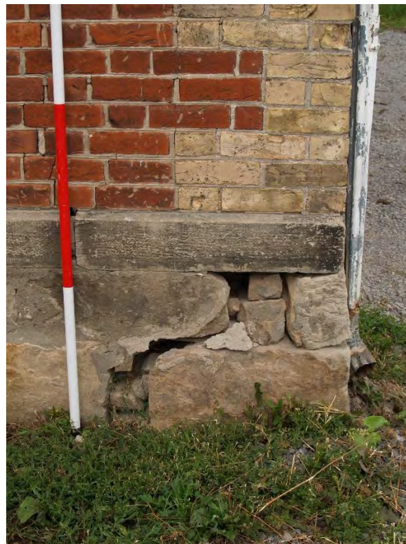
Figure 14: Capping stone and coursed rubble foundation at the southeast corner (August 2018)
