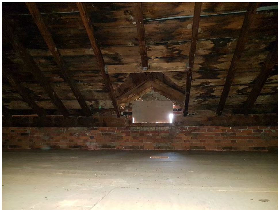
Figure 40: Attic with blind window in the cross gable (August 2018)
