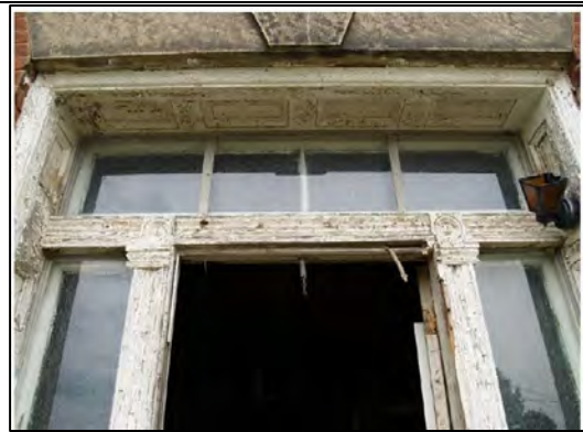
Front Door showing wood detailing
