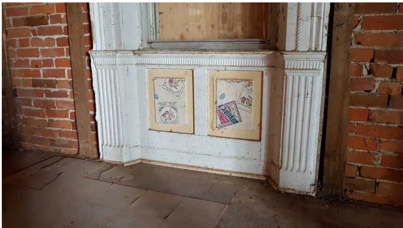
Figure 33: Window with trim and panelling along the south wall.
