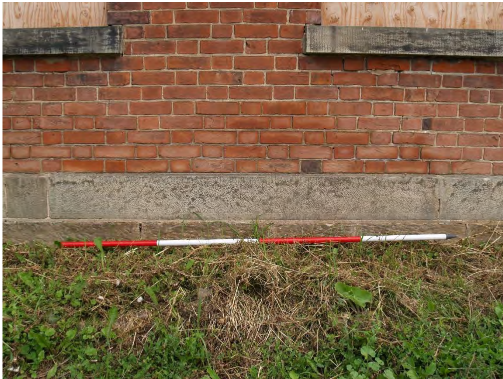
Figure 13: Ashlar stone plinth on the east façade (August 2018)
