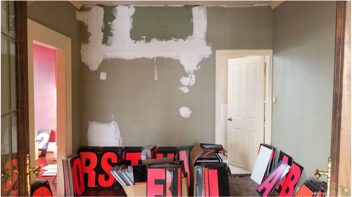
Figure 24: Central room showing entrance to southwest room (left) and bathroom (right)
