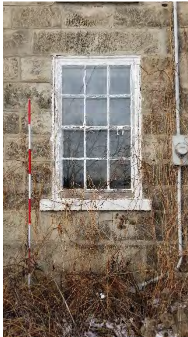
Figure 17: Six-over-six window
