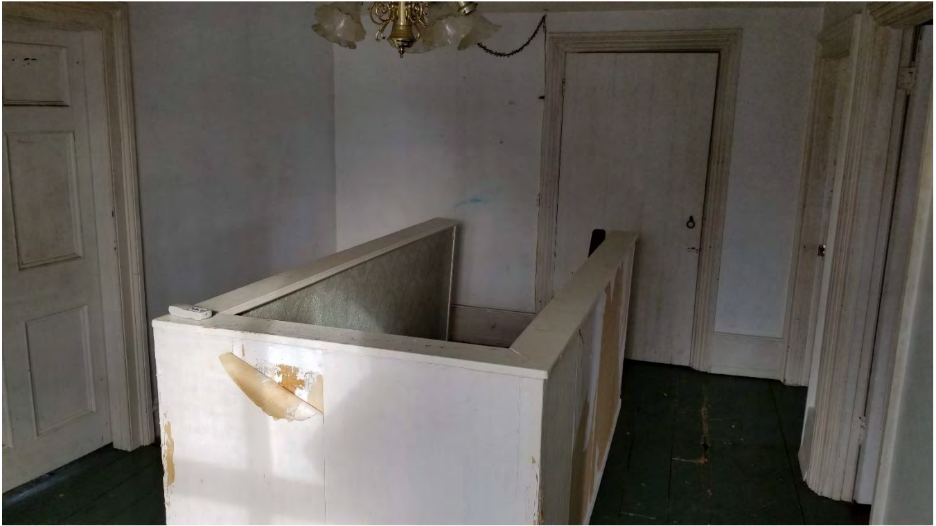
Figure 31: Second storey hallway facing north
