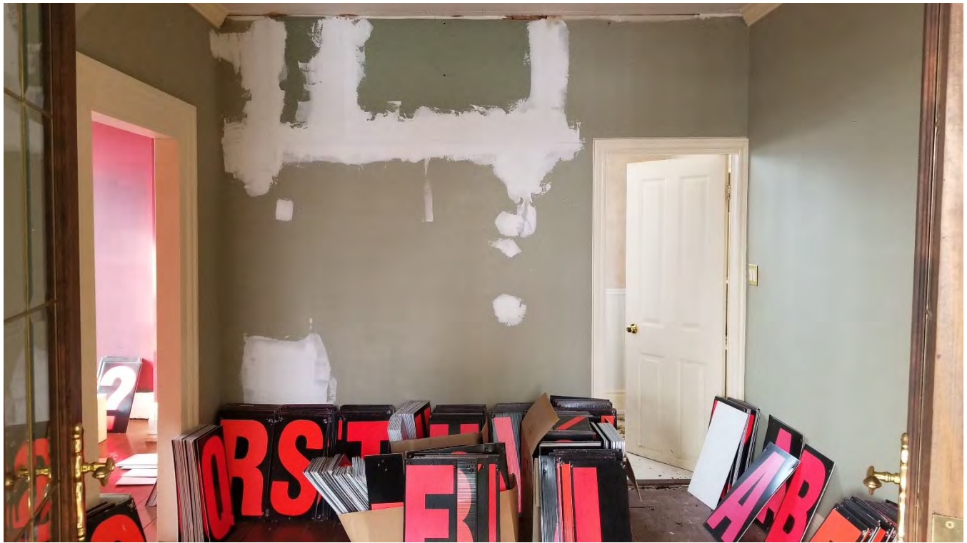
Figure 25: Central room showing entrance to southwest room (left) and bathroom (right)
