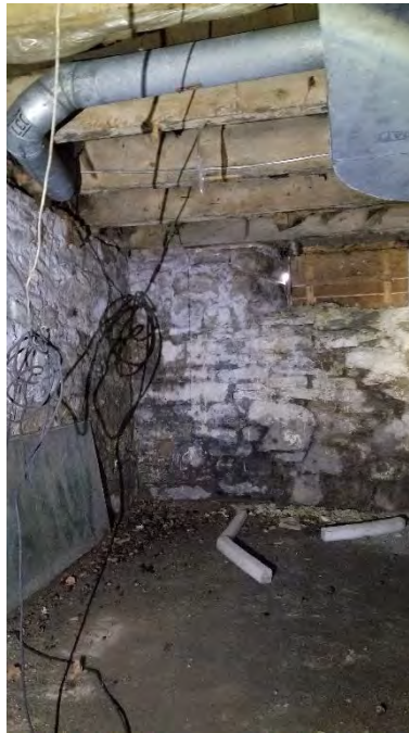
Figure 44: Milled joists
