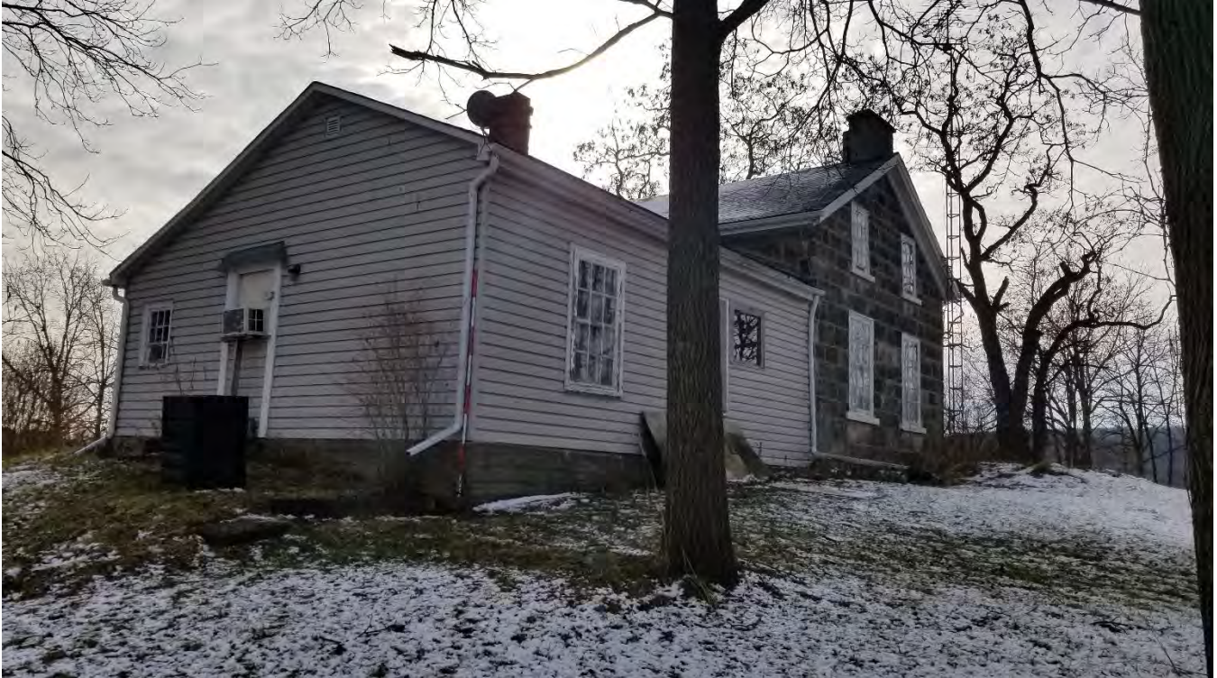
Figure 45: West and north façades
