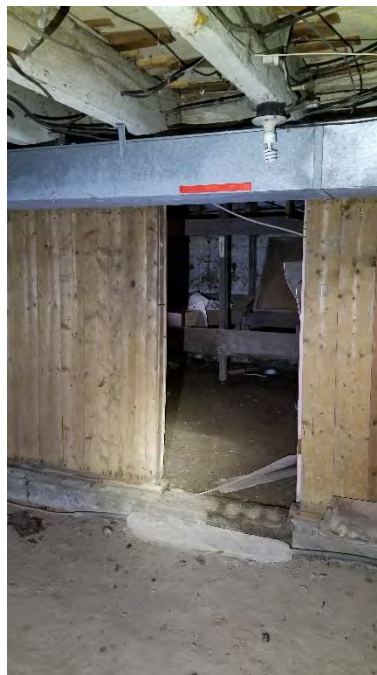
Figure 41: Wood panelled wall
