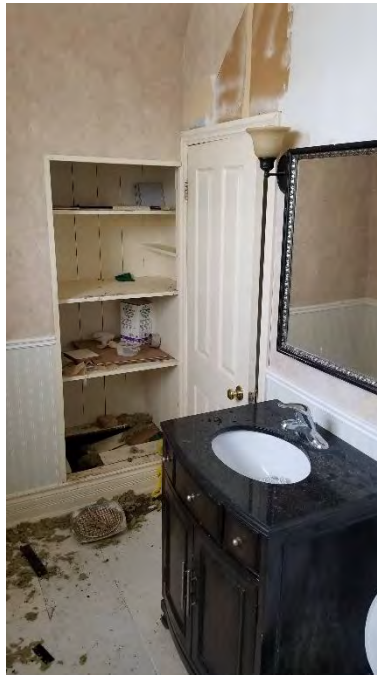
Figure 28: Main floor bathroom to the west of the central room
