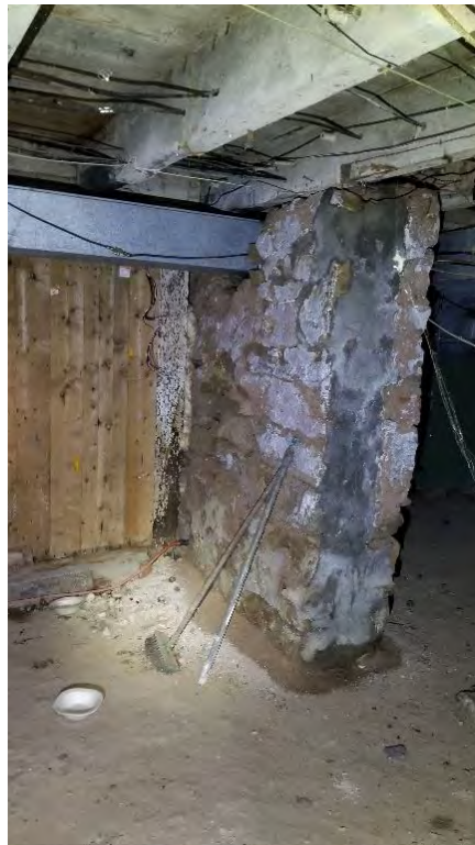
Figure 39: Stone partition wall
