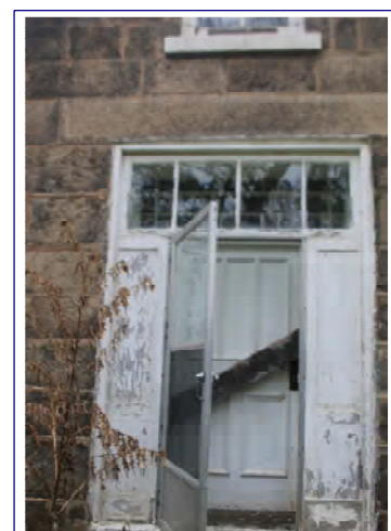
STORM DOOR SET RECONSTRUCT AND RETURN TO HISTORIC DETAIL
