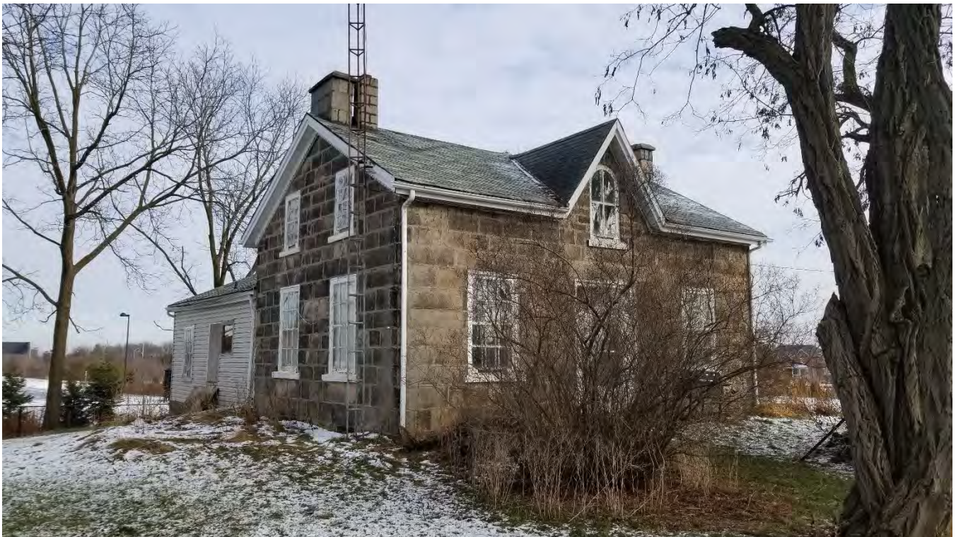
Figure 12: South and west façades
