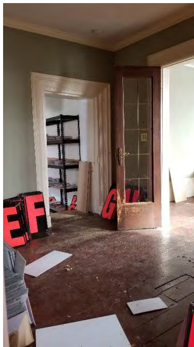
Figure 25: Central room showing access to the extension (left)
