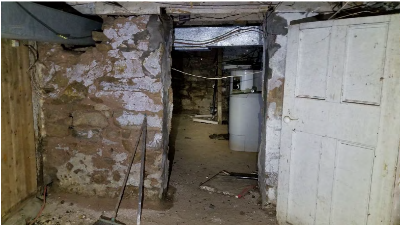
Figure 43: Basement facing north
