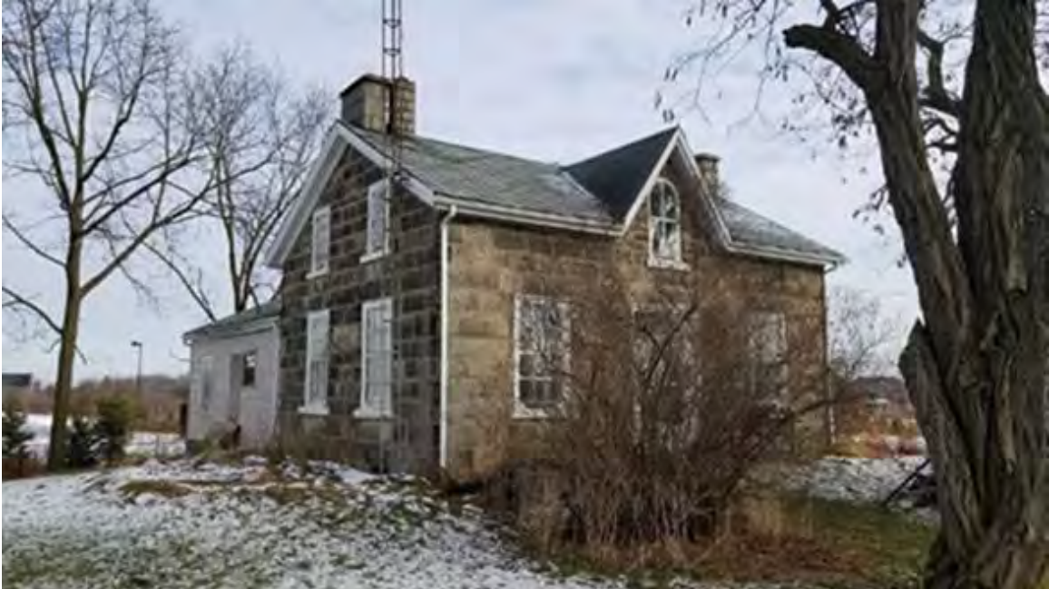
South and West Facade
