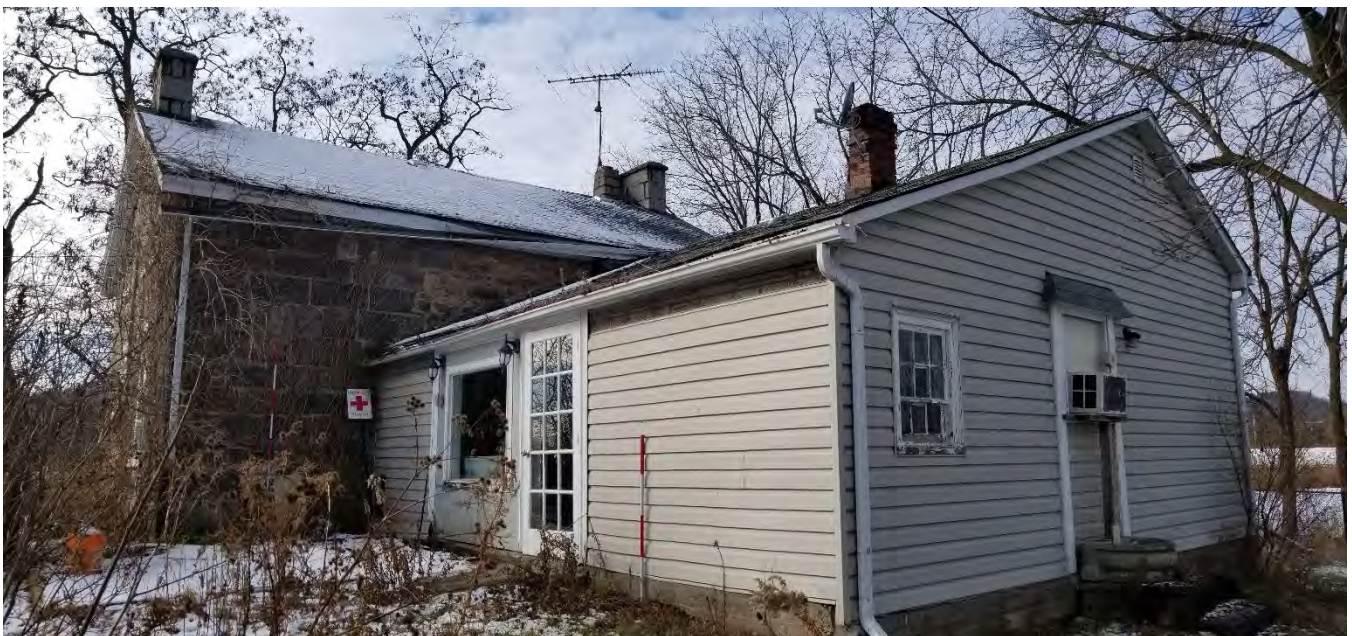
Figure 11: East and north façades
