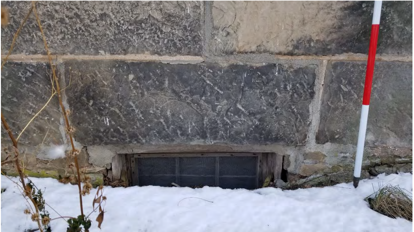
Figure 15: Cut stone cladding in even courses and double struck mortar joints
