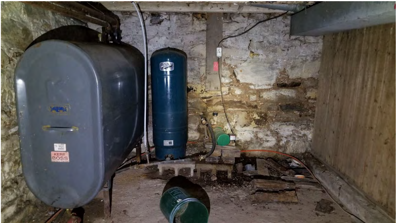
Figure 41: Oil tank at the southwest corner of the basement.
