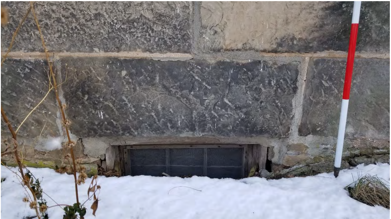
Figure 14: Ashlar masonry above the coursed rubble foundation
