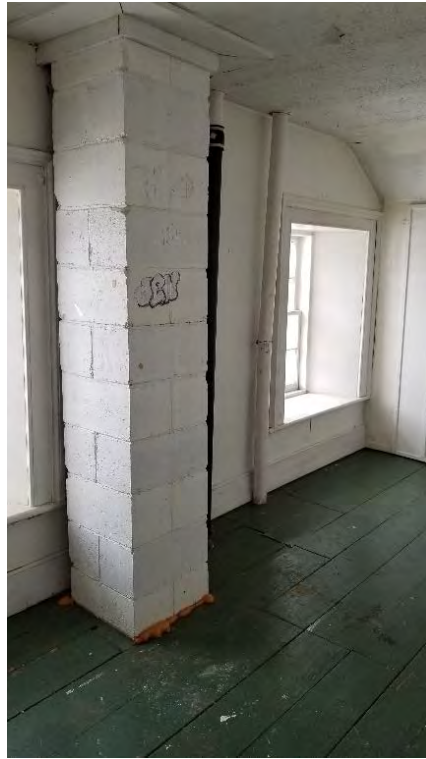
Figure 36: CMU chimney stack in the west room
