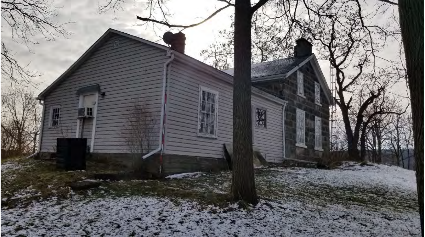
Figure 45: West and north façades
