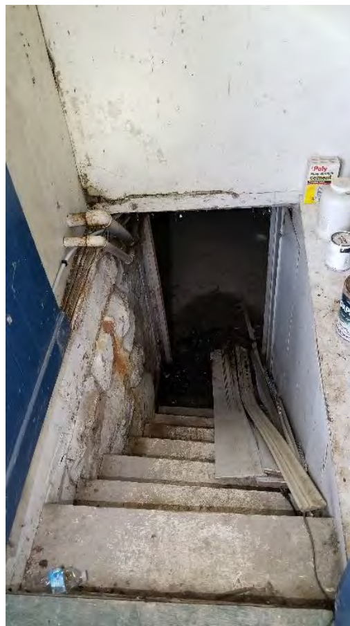
Figure 38: Stairs leading to the basement
