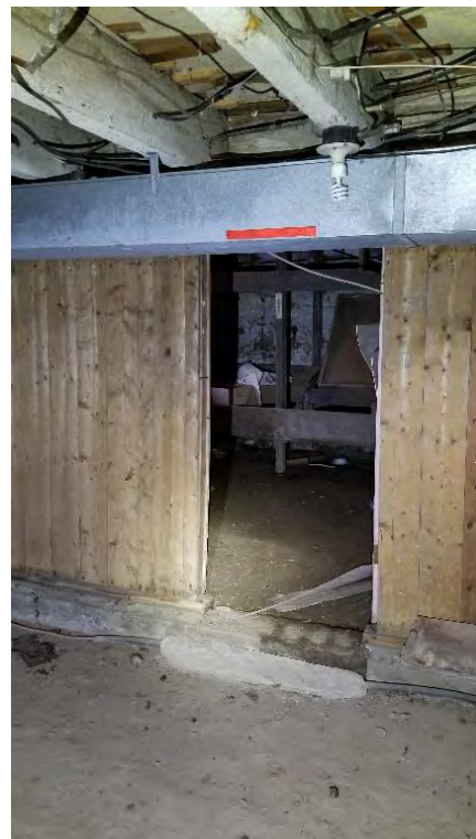
Figure 40: Wood panelled partition wall
