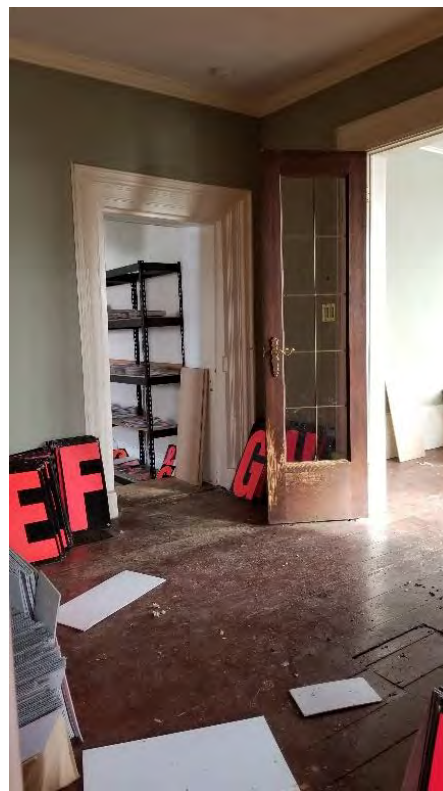
Figure 26: Central room showing access to the extension (left)
