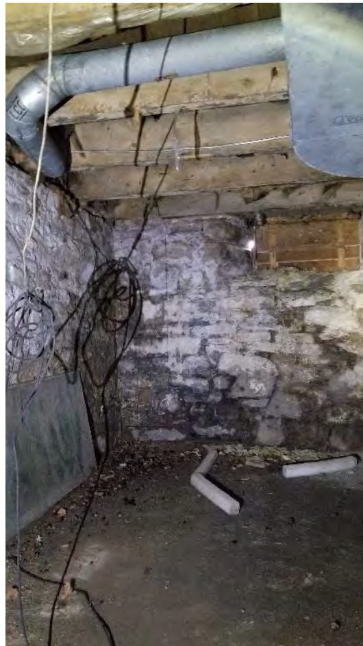
Figure 43: Milled first level floor joists as seen from the basement
