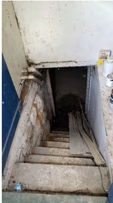
Figure 39: Stairs leading to the basement
