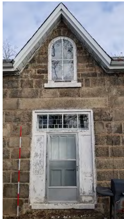
Figure 18: Main entrance on the south facade with four-pane transom
