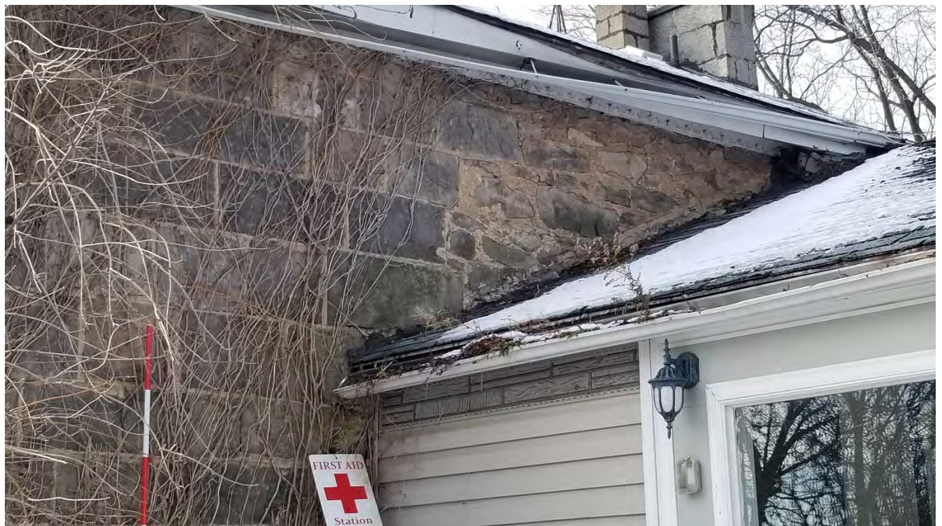
Figure 15: Section of rubble masonry on the north wall
