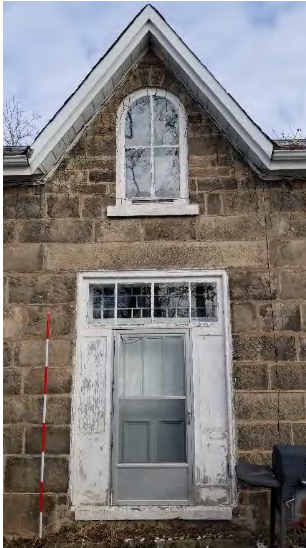
Figure 19: Central entrance and cross-gable on the south façade
