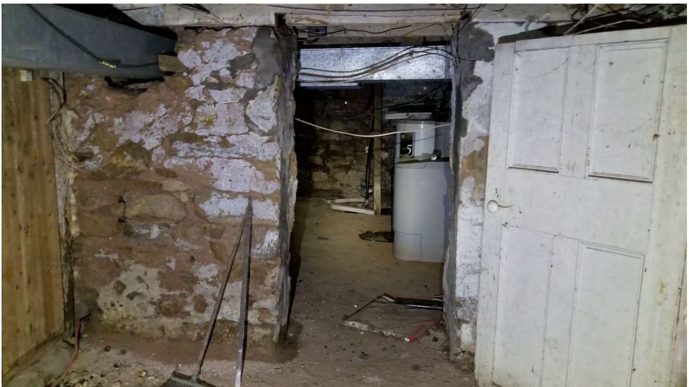
Figure 42: Basement facing north
