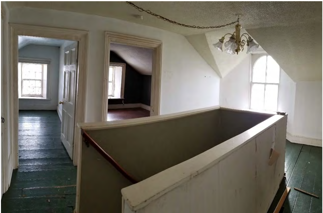
Figure 31: Second storey central hallway facing south
