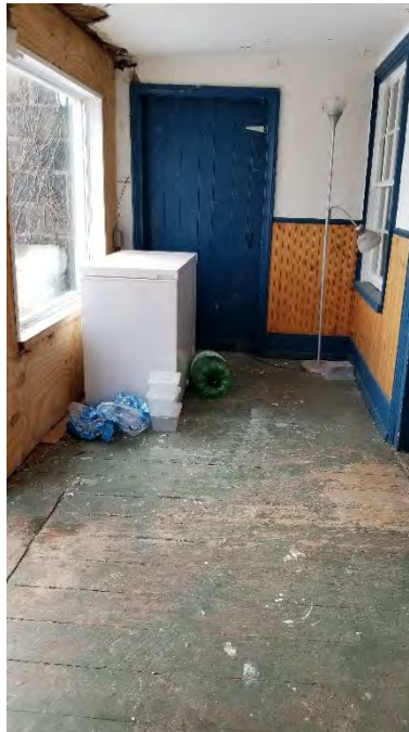
Figure 47: Mudroom facing south towards the basement entrance
