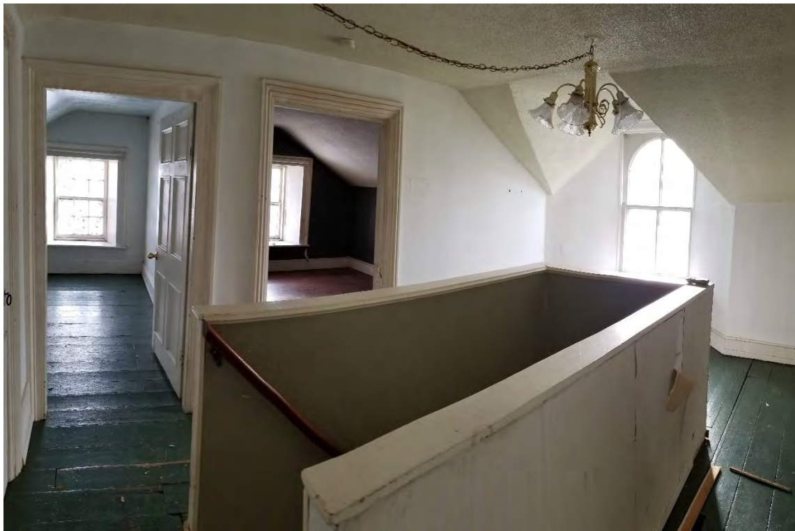
Figure 30: Second storey central hallway facing south
