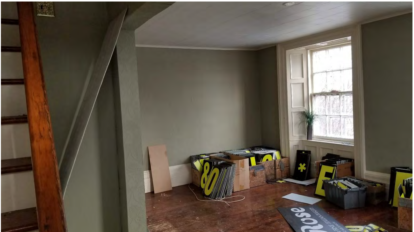
Figure 22: Room to the east of the main entrance
