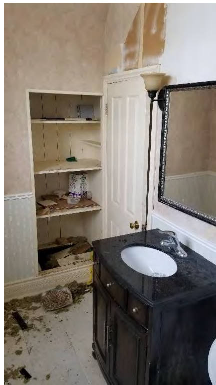
Figure 29: Main floor bathroom to the west of the central room
