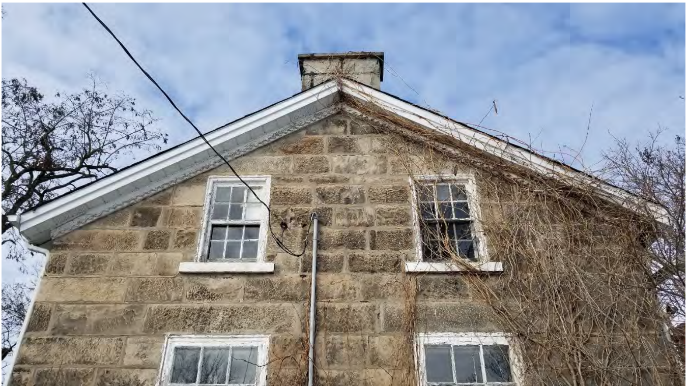
Figure 16: Medium gable roof with moulded fascia
