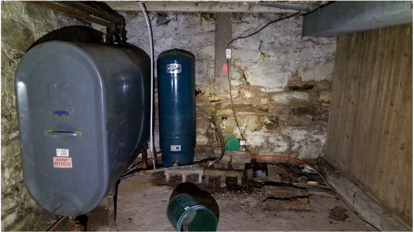
Figure 42: Oil tank at the southwest corner of the basement.
