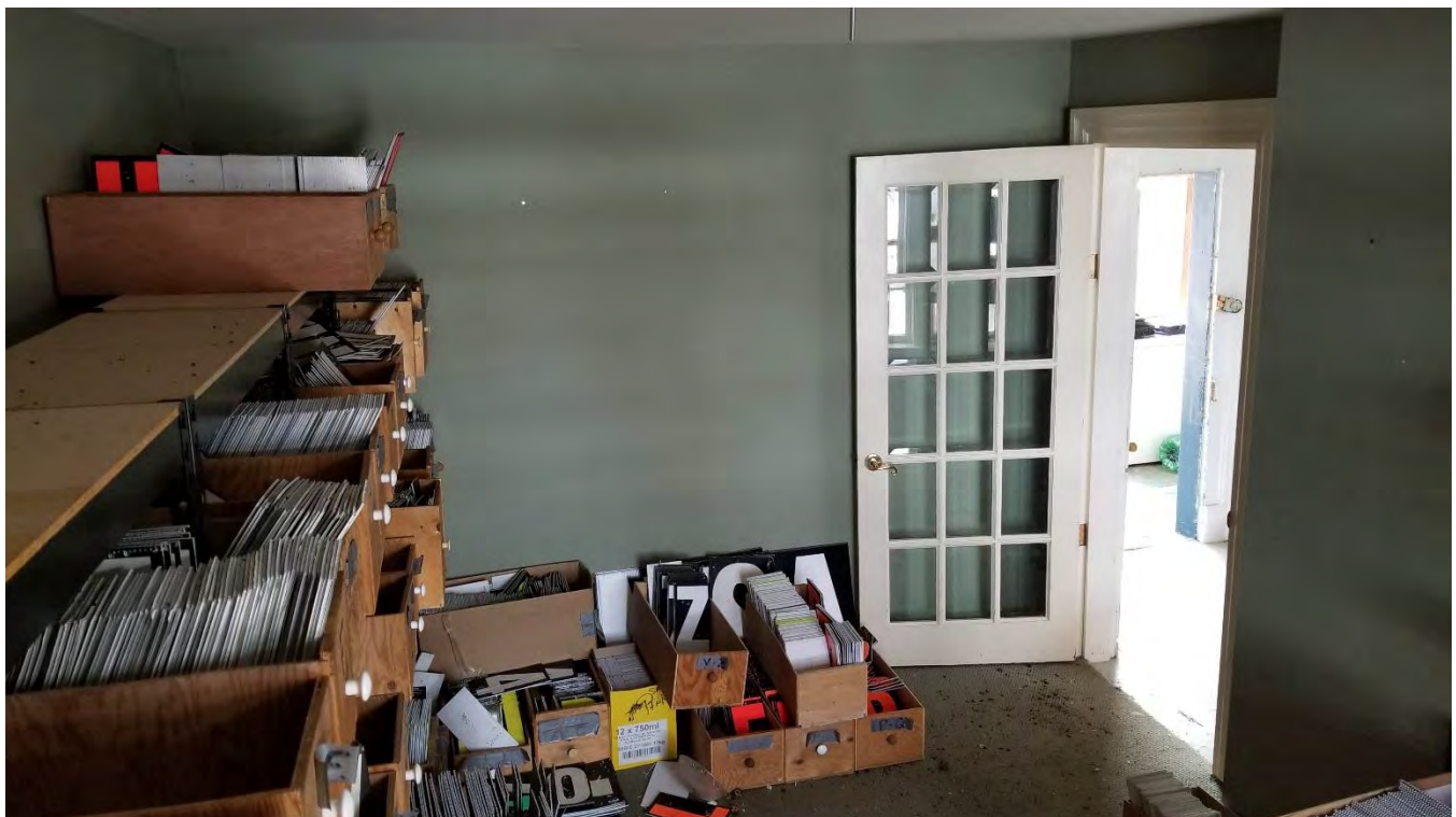
Figure 53: Room to the north of the kitchen
