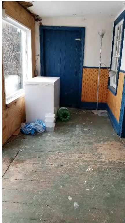
Figure 48: Mudroom facing south towards the basement entrance
