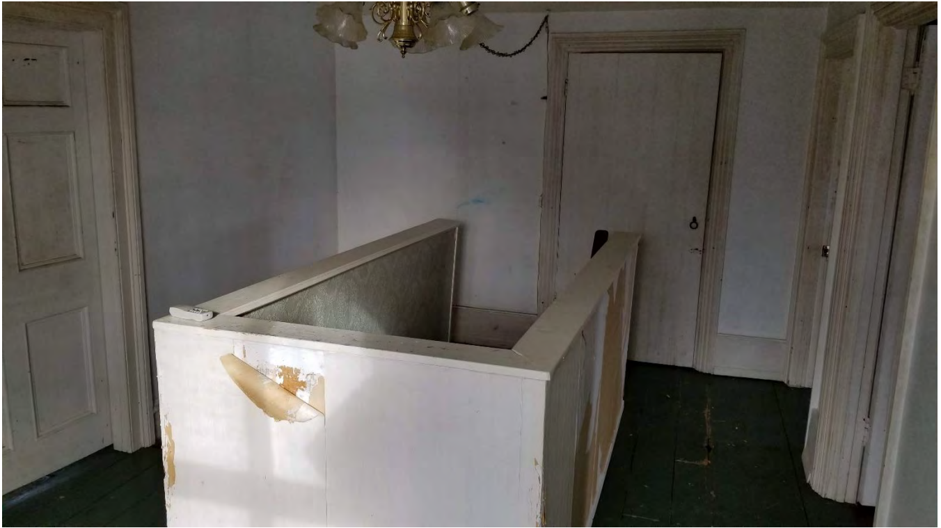
Figure 31: Second storey hallway facing north
