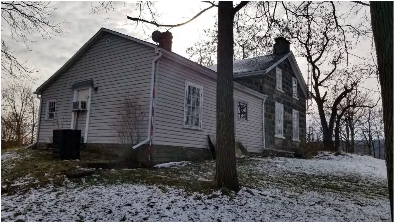
Figure 10: North and west façades
