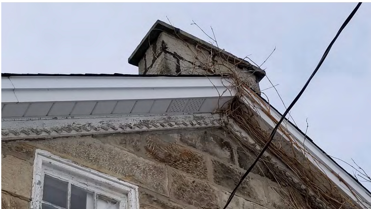
Figure 17: Stone chimney with chamfered cap
