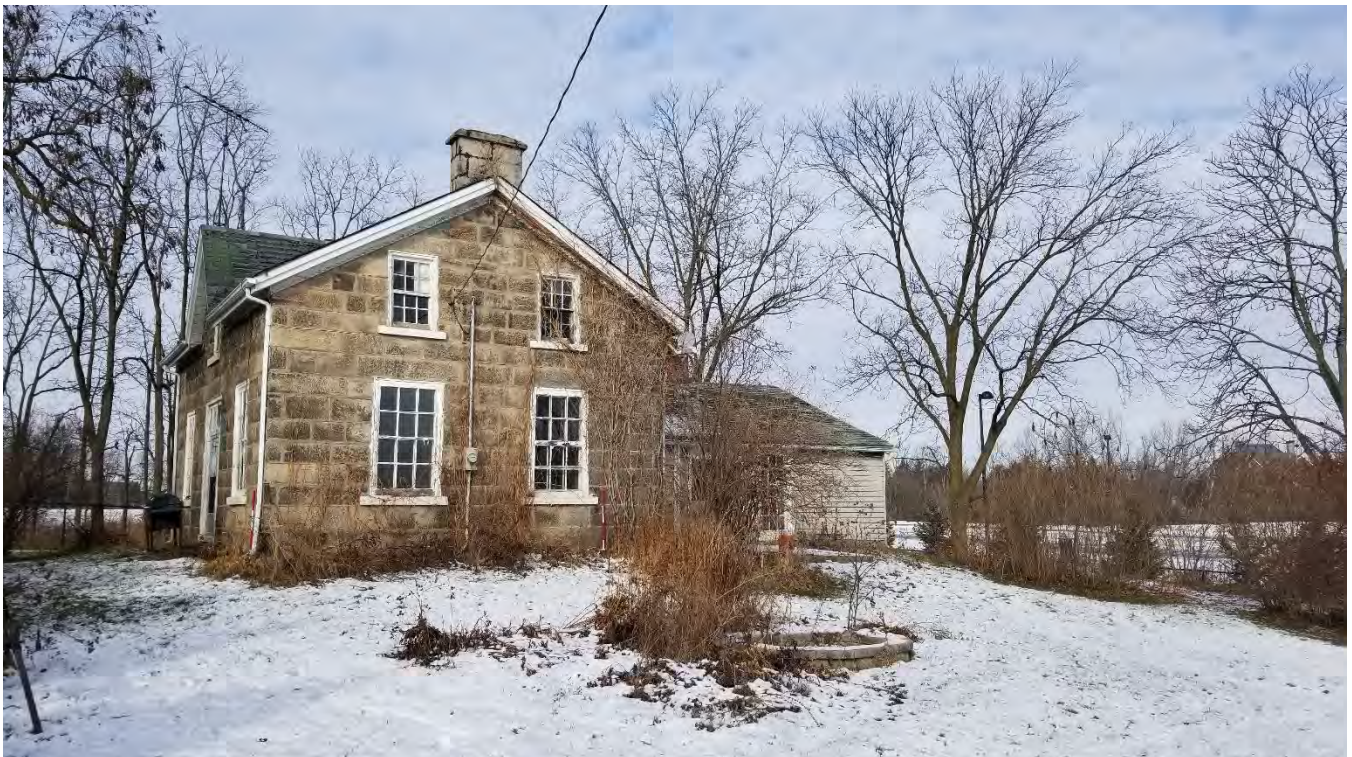
Figure 13: South and east façades
