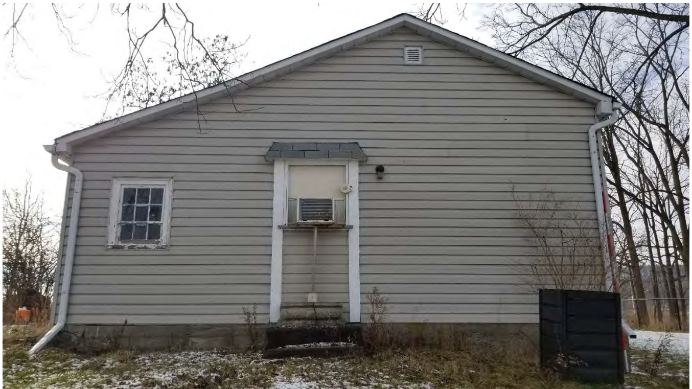
Figure 45: North end wall
