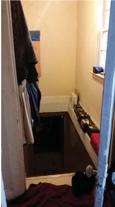
Figure 59: Basement access in the north wing extension.
