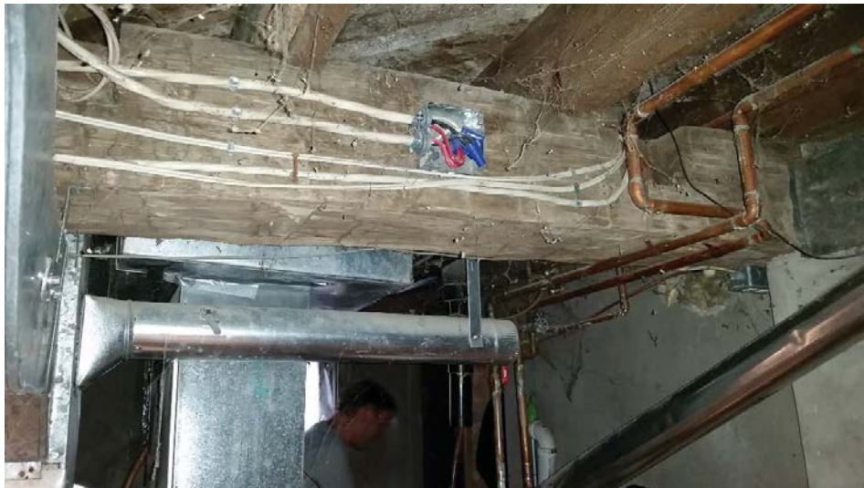
Figure 61: Hand hewn beam in the north wing basement.
