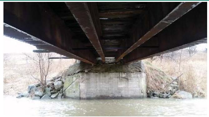
I-beam framing and concrete embankment, facing north
