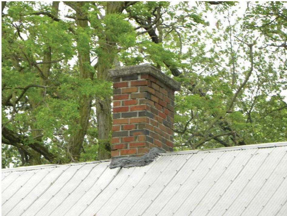
Figure 55: North wing chimney with concrete cap (2012).
