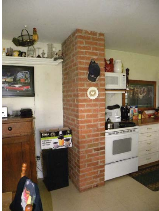
Figure 57: Exposed stack in the north wing kitchen.
