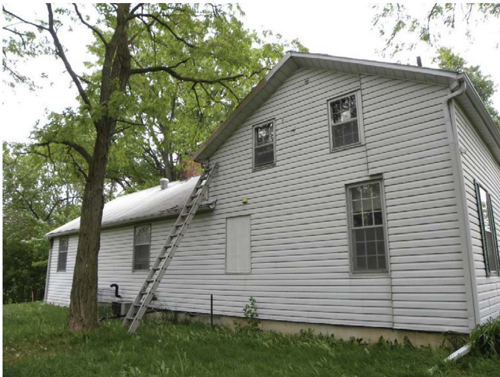
Figure 22: West façade of Bowes House (2012).
