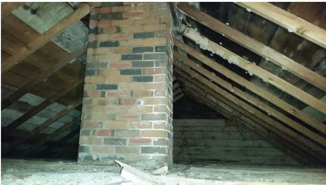
Figure 63: Roof construction and chimney stack in the north wing attic.
