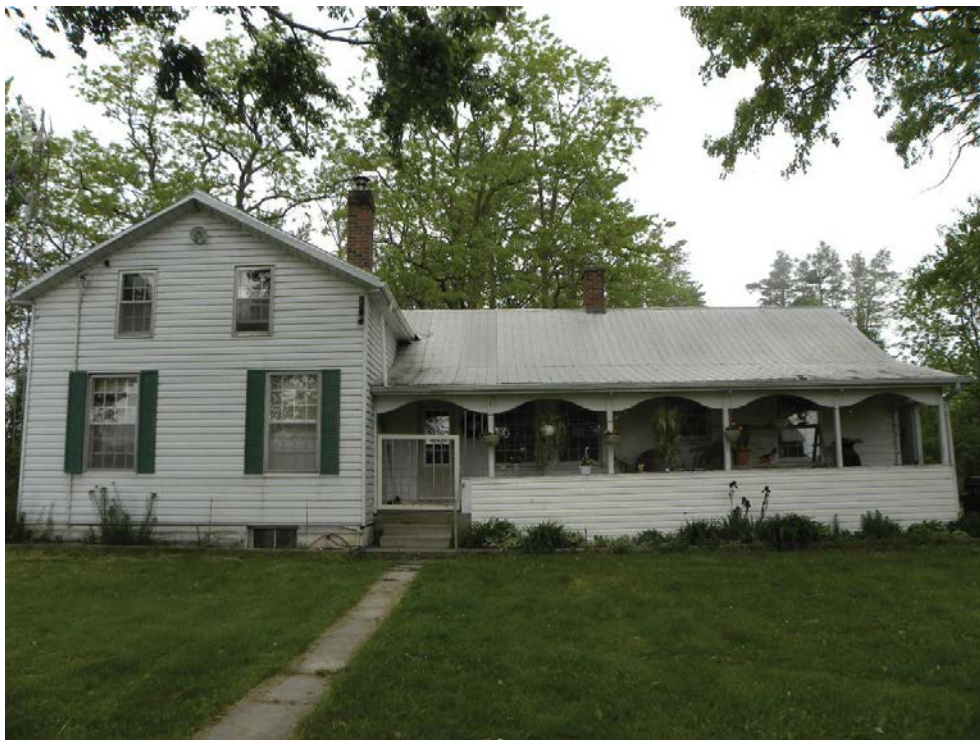
Figure 26: East façade of Bowes House (2012).
