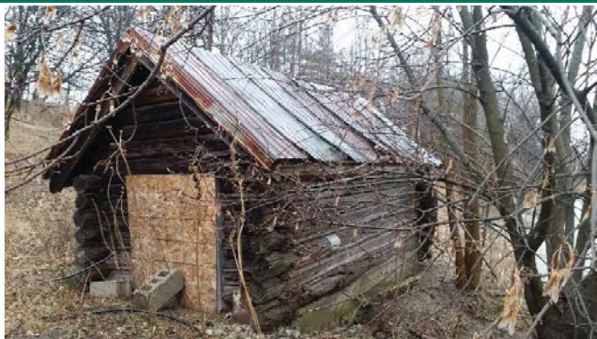
Left: East and north façades
