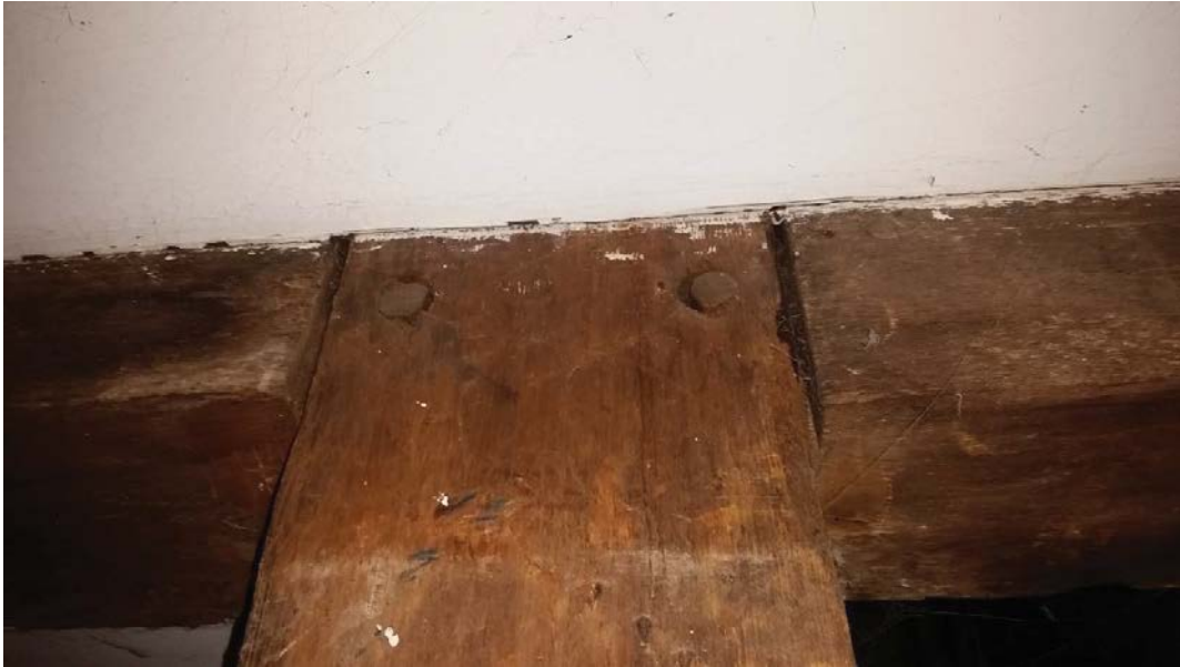
Figure 30: Principal post for a central bent, morticed and pinned to cross-braces.
