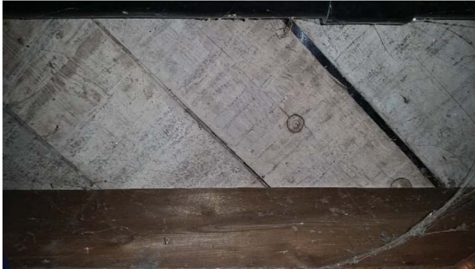
Figure 62: Diagonal flooring as seen from the north wing basement.
