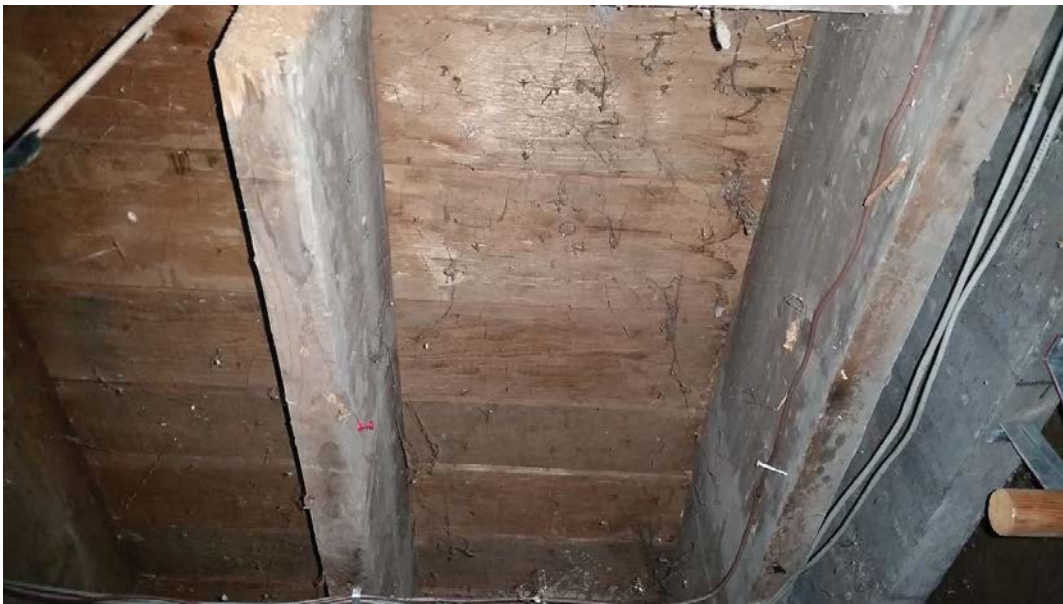
Figure 52: Joist and floorboard construction as seen from the main block basement.
