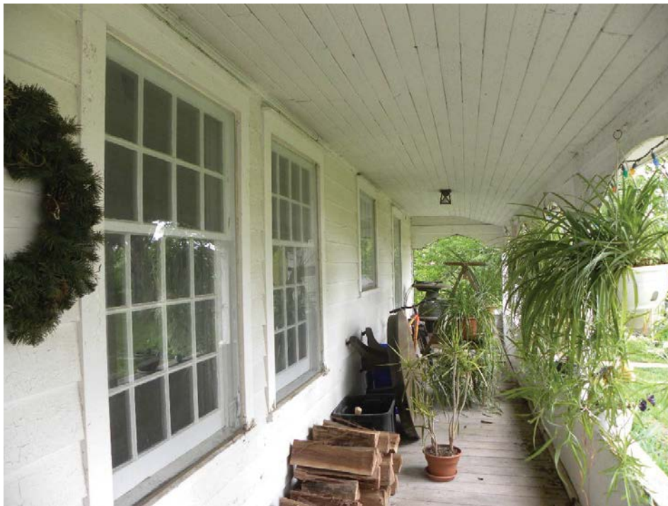
Figure 64: View of the verandah, facing north (2012).
