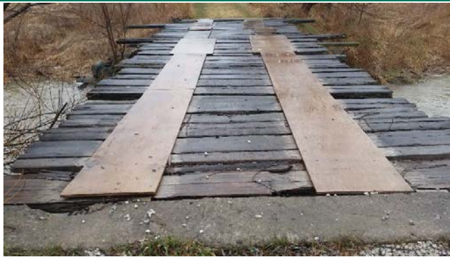
Decking, facing north
