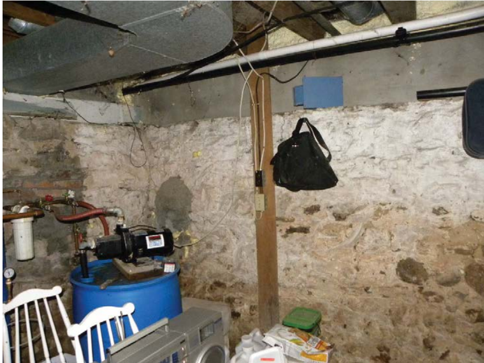
Figure 60: Coursed rubble foundation in the north wing basement.
