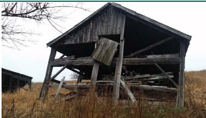
South façade of the east barn
