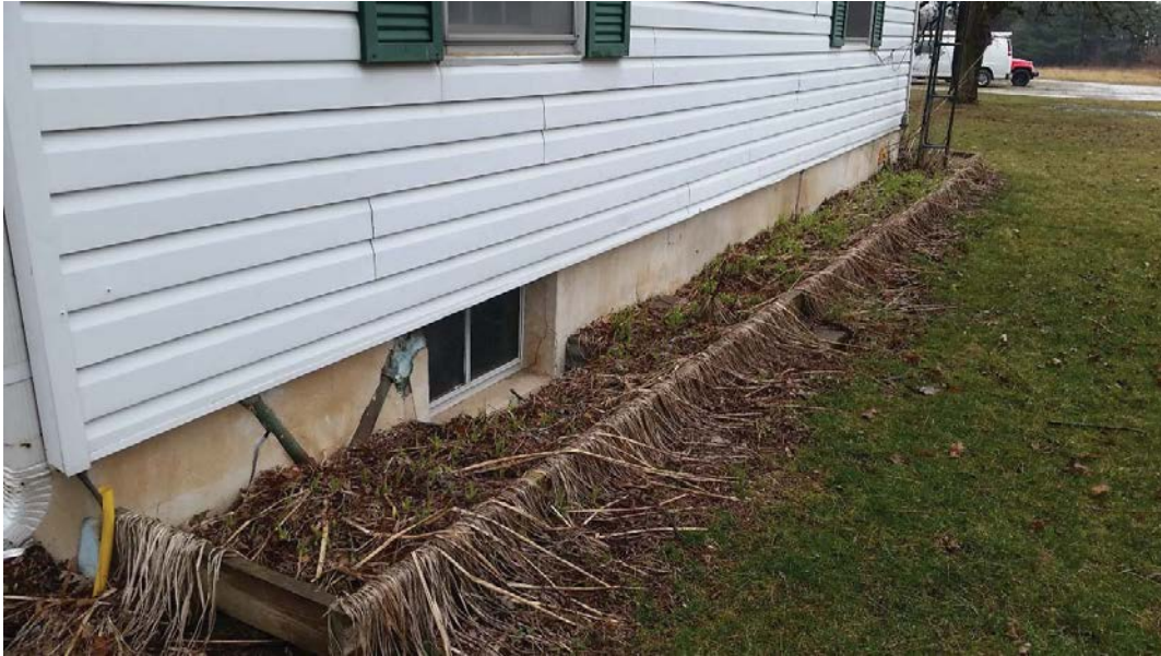
Figure 28: Portland cement parging on the south foundation.
