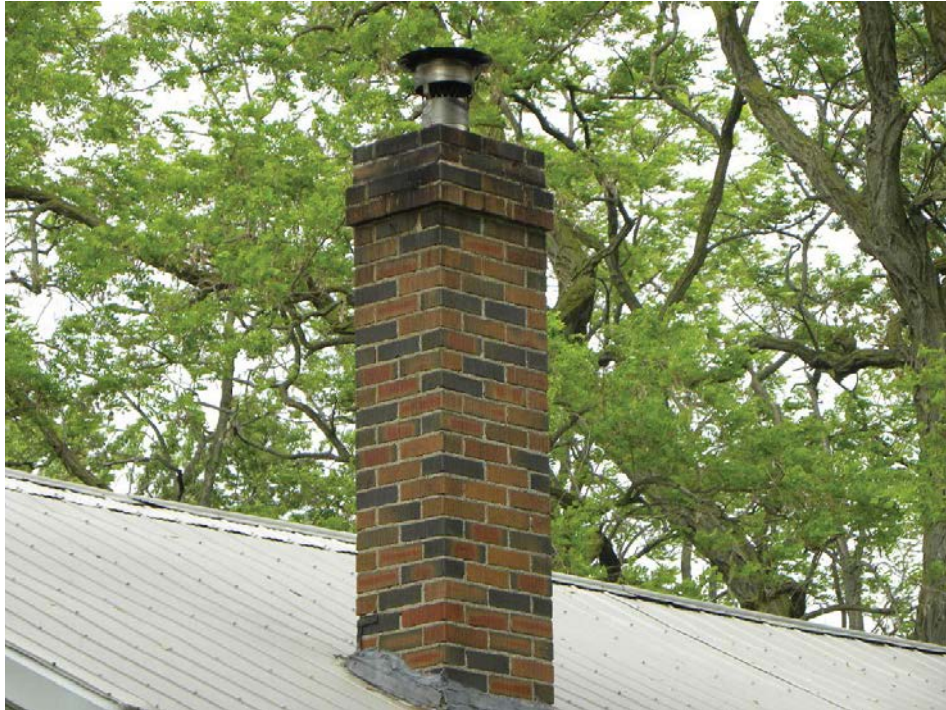
Figure 36: Main block chimney stack (2012).
