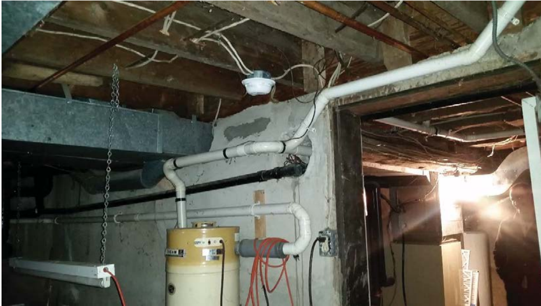
Figure 53: Joists running to the hand hewn sill on the north wall of the main block.
