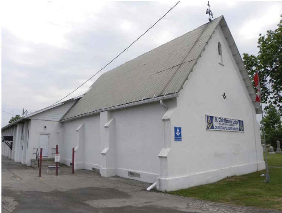
Figure 4: View facing northeast of the former Bowes Presbyterian Church (2012).
