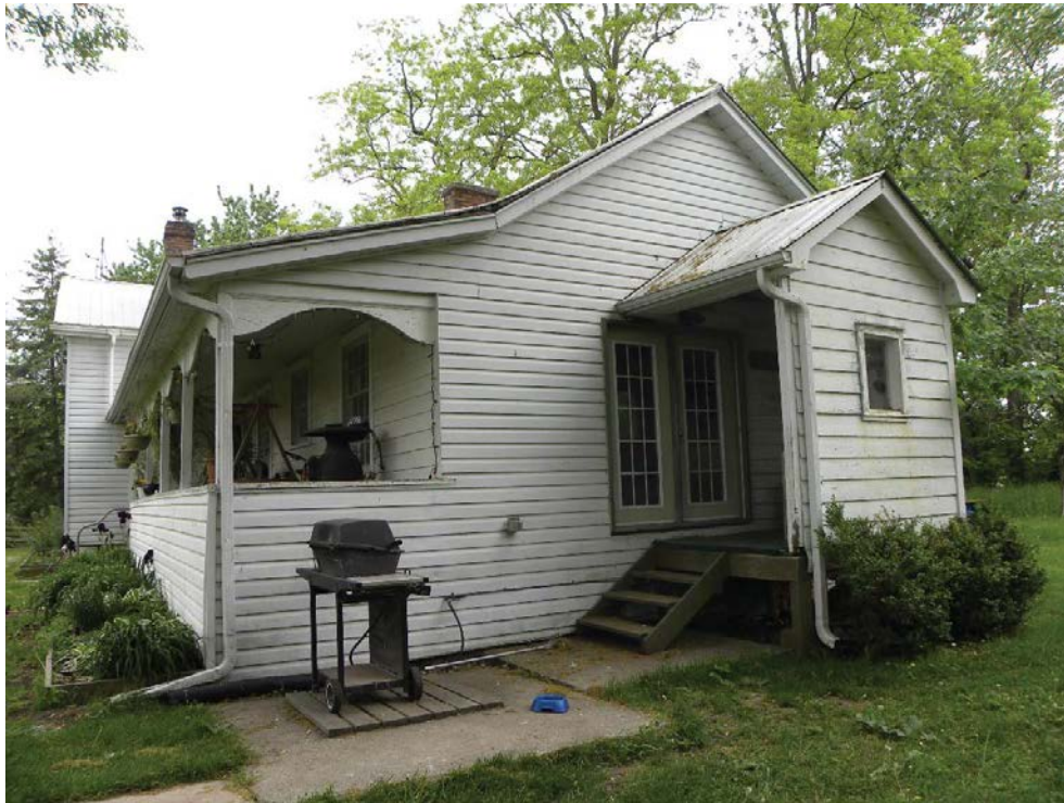
Figure 25: East and north façades of Bowes House (2012).
