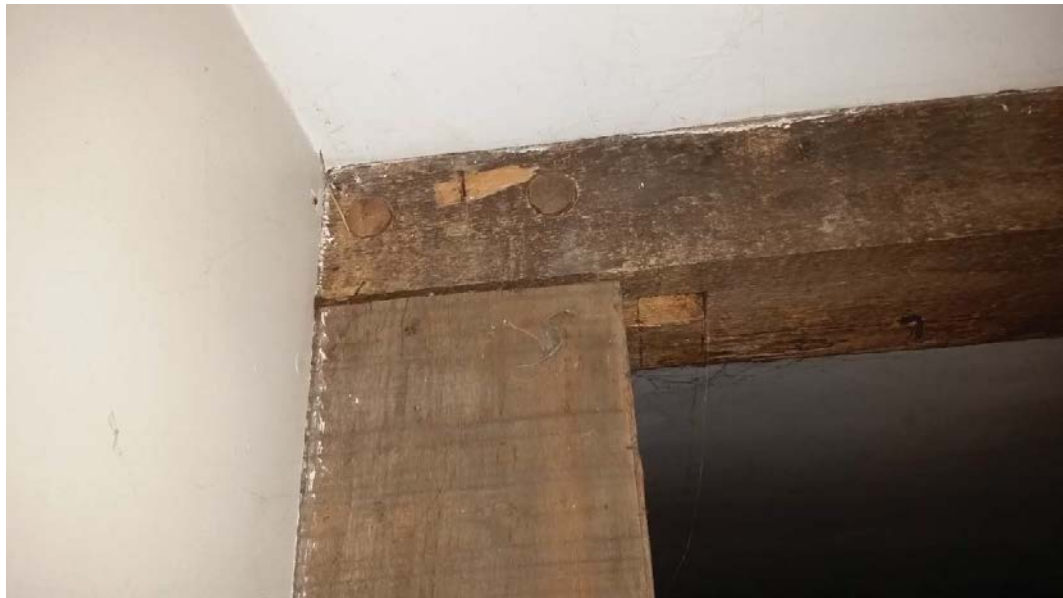
Figure 31: Vertical stud pinned to a cross brace.
