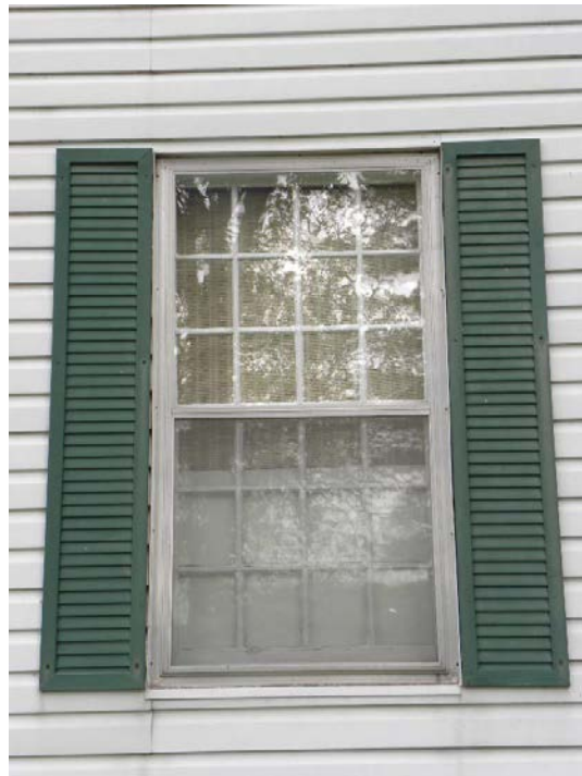
Figure 37: Typical ground floor window on the main block (2012).
