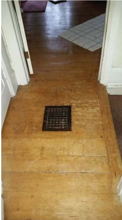
Figure 46: Landing at the main block second level, facing west.
