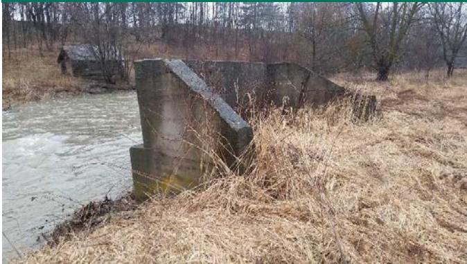
View of the embankment facing south
