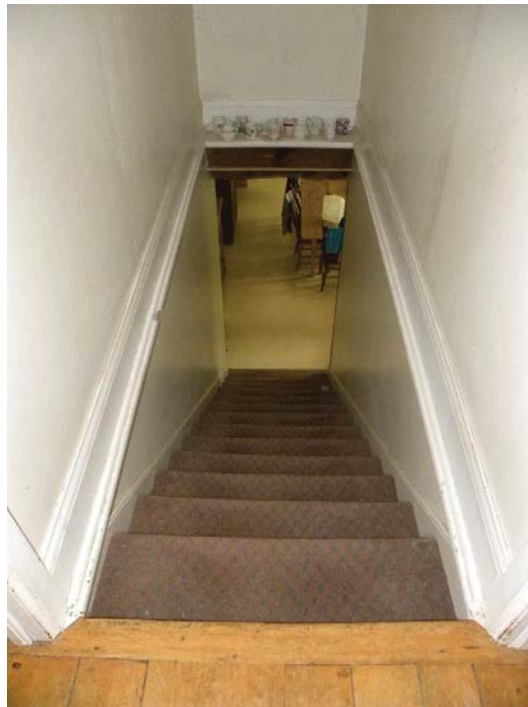
Figure 45: Main block staircase, facing north.
