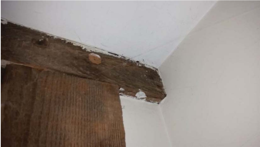
Figure 32: Vertical stud pinned to a cross brace.
