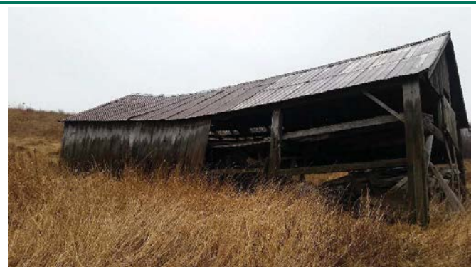
West façade of the east barn
