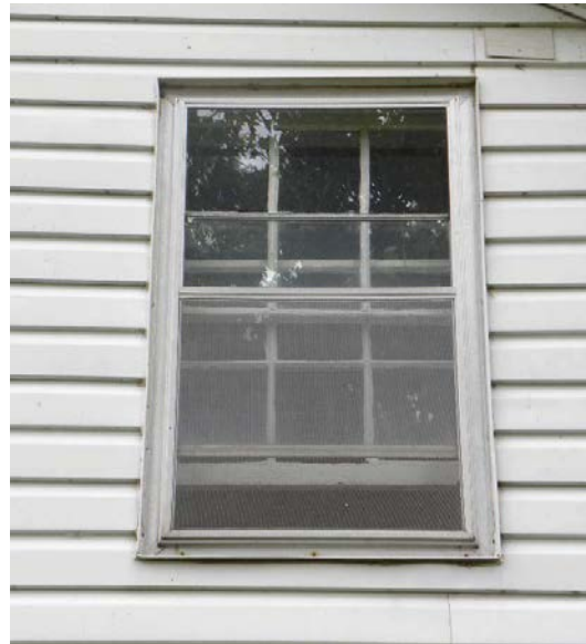
Figure 38: Typical second floor window of the main block (2012).
