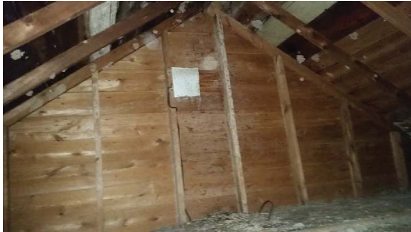
Figure 65: Plank sheathing in the gable of the north wing extension.
