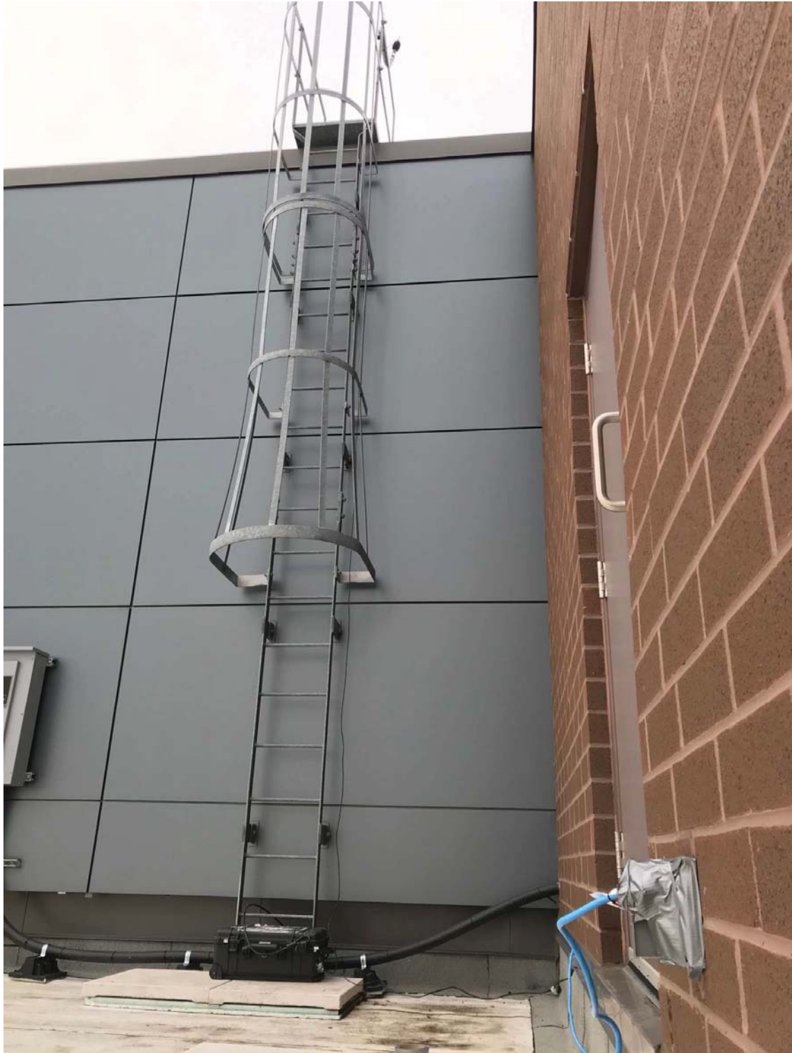
B 4: Measurement Location 4 Set Up
