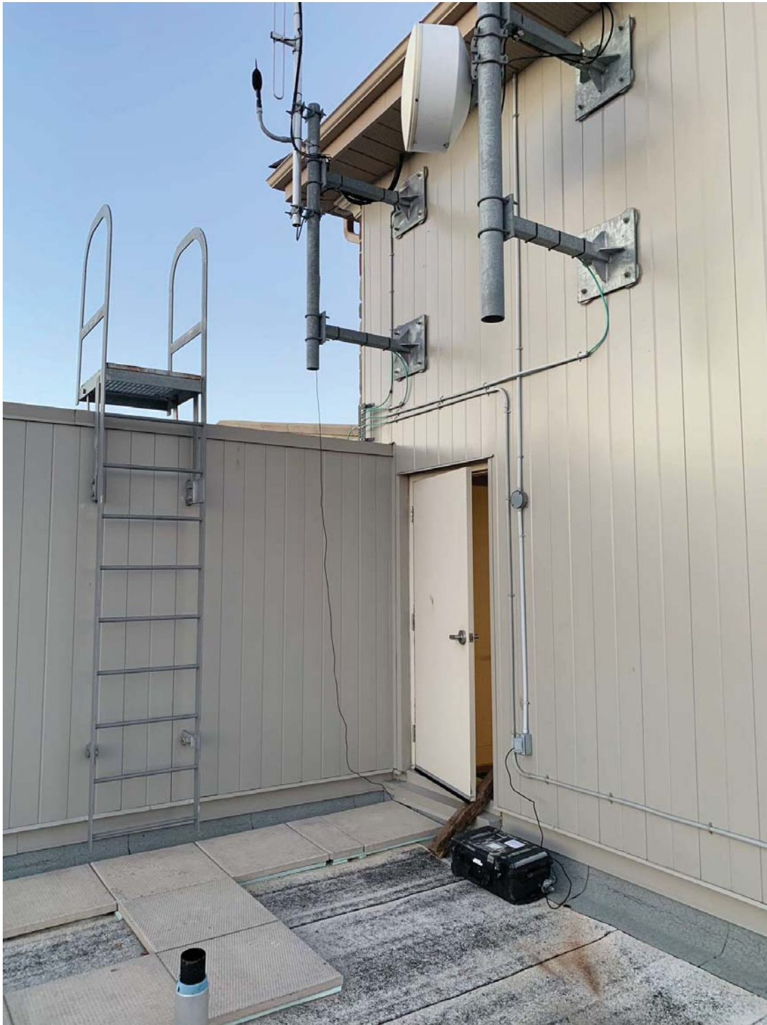
B 1: Measurement Location 1 Set Up
